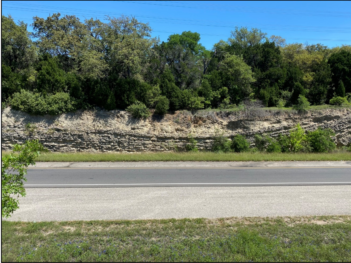
Project Photo 2. The Loop 1 Syncline is an expression of downward folded bedding in the Georgetown Formation. Folded beds can be seen along the ramp from southbound Mopac to southbound State Loop 360. The hinge line of the sinkhole is shown as a purple line on the geologic map (COA 2014).
