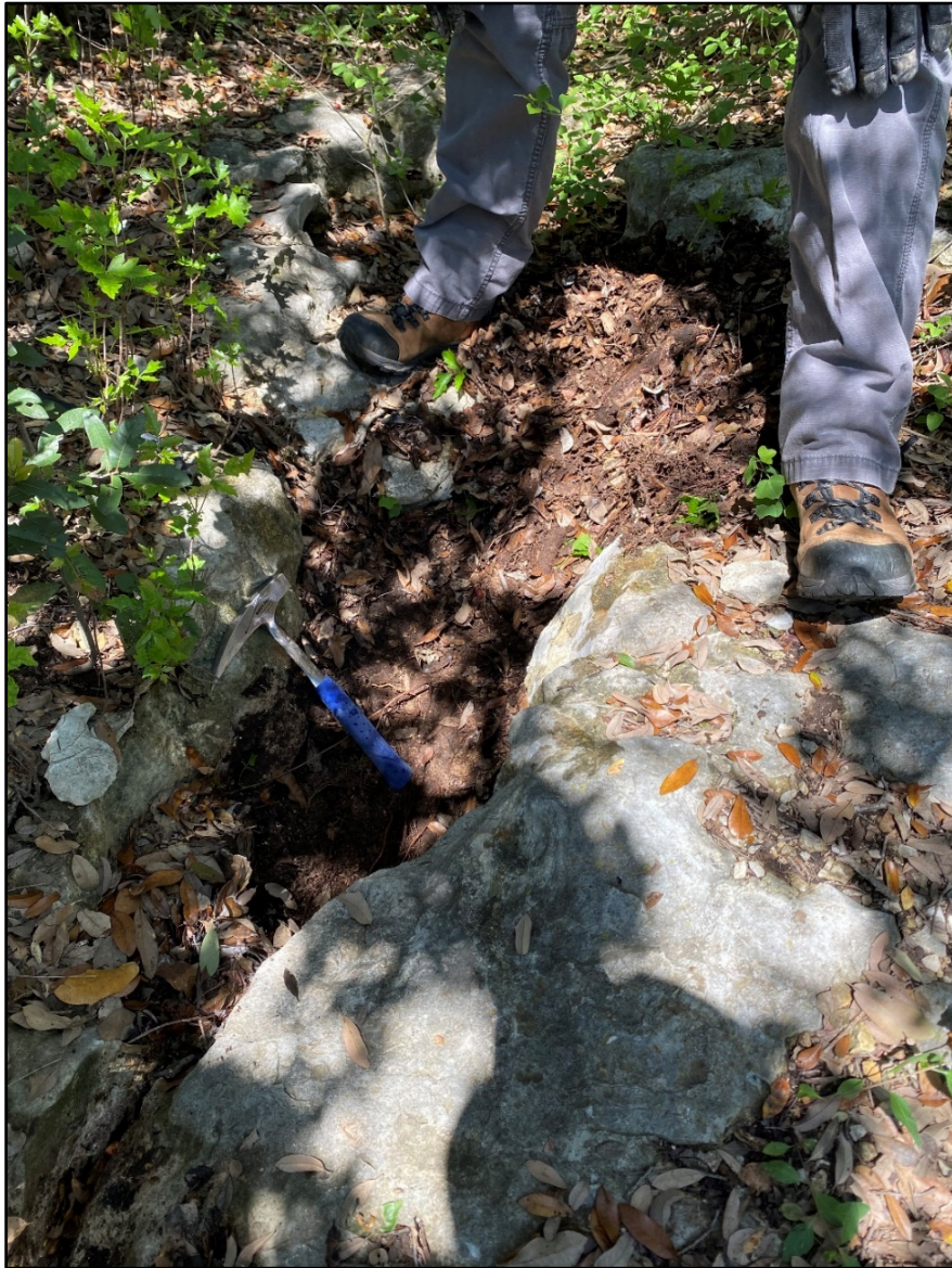
Feature Photo MPS-19 Solution Enlarged Fracture (Photo 2 of 2). The hammer is for scale at the widest part of the fracture (18 inches). The depth is at least 15 inches but could extend further as the leaves and soil filling the fracture are loose.
