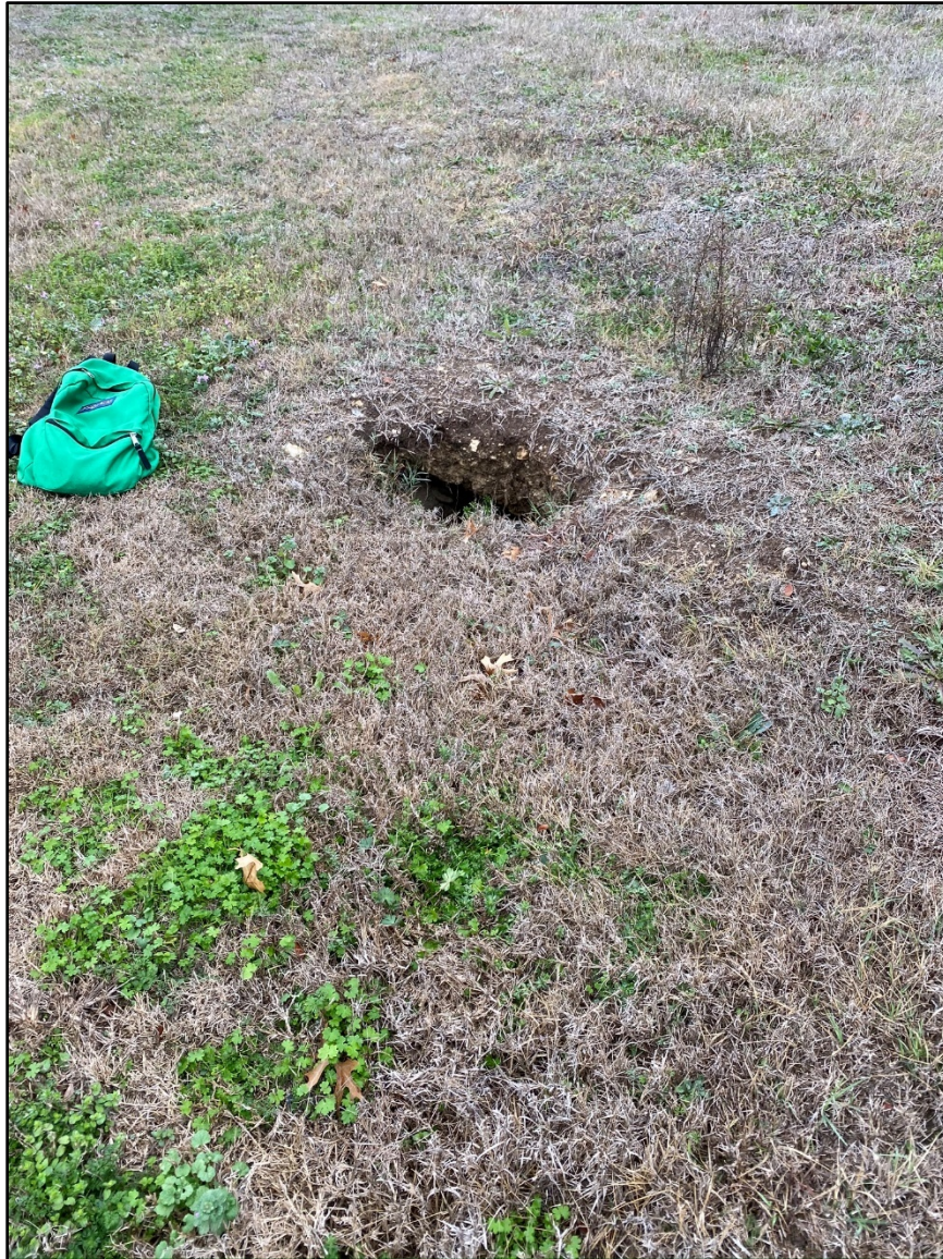
Feature Photo MPS-27 Non-karst Closed Depression.
