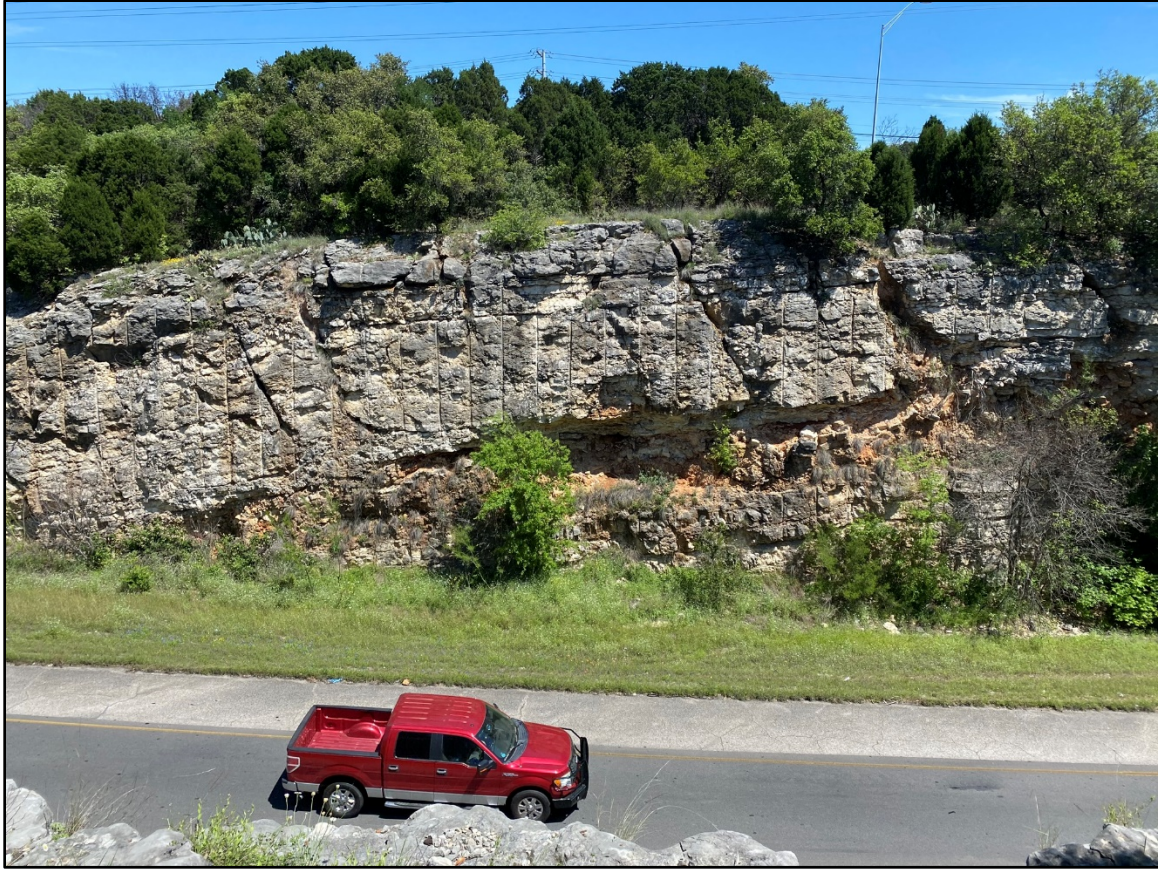
Project Photo 1. Fault lines of the Balcones Fault Zone are expressed in sets that reflect adjustments within damage zones. There is an angular contrast between vertical drill scars and slashed fracture lines. This image is facing northeast along the ramp from southbound MoPac to southbound SL 360 (towards South Lamar Boulevard). On the left side of the photo, strata are dipping northwest towards the Loop 1 Syncline (Detail in Project Photo 2). This fault crosses the Project Area from 550 feet south of Tuscan Terrace to 820 feet north of Barton Creek at a 45° trend and has a displacement of 40 feet.
