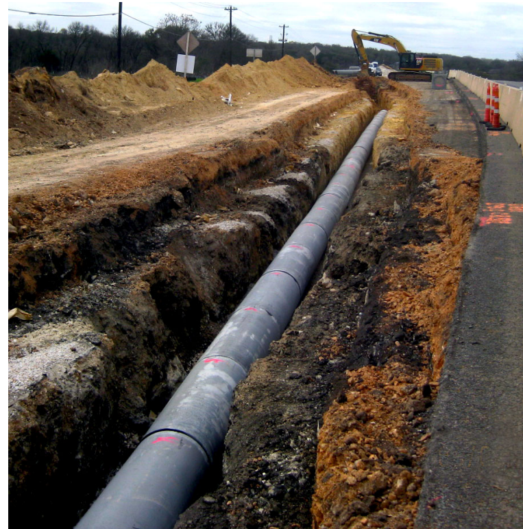
Storm Sewer Network for Water Quality Ponds
