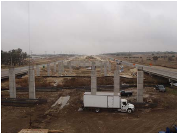
Bridge columns at RM 2243, looking south
