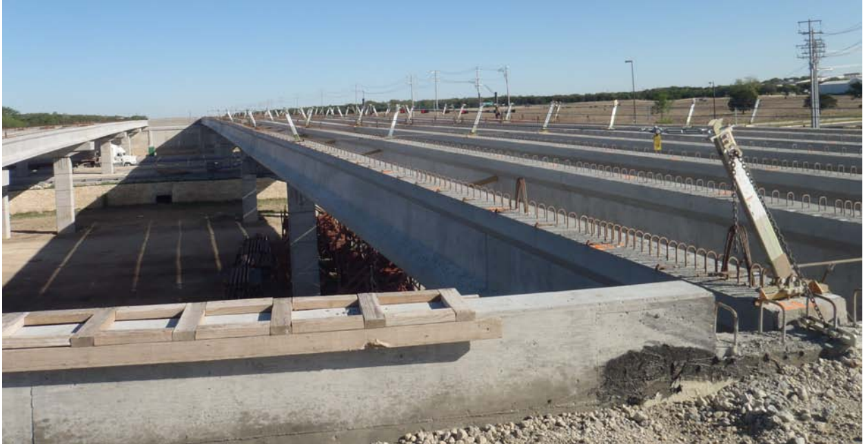
The bridge beams at Crystal Falls Parkway, facing north
