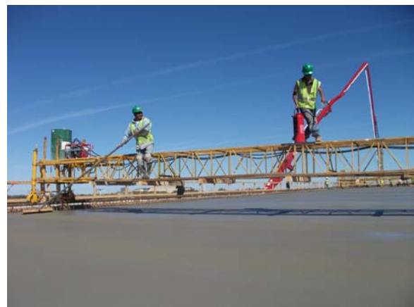
Finishing the concrete bridge deck surface with a broom
