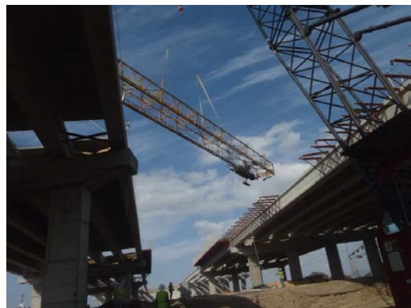
Setting up a smoothing and leveling device for freshly placed concrete
