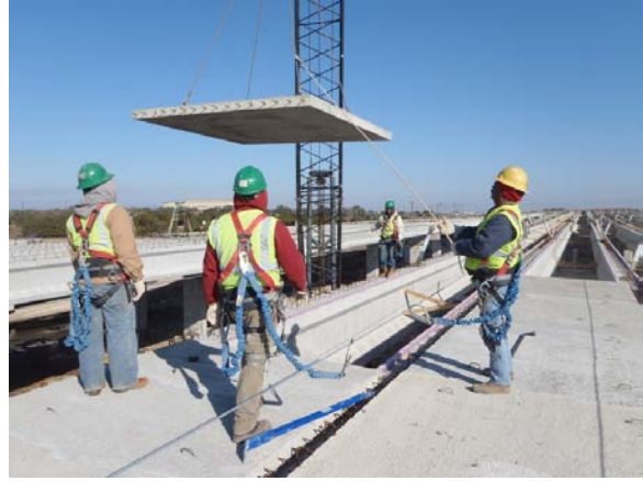
Setting deck panels at New Hope Drive
