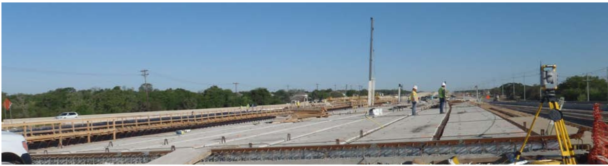
Placed deck panels at the Block House Creek Bridges
