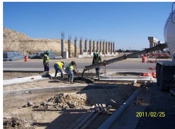
Placing concrete for the sidewalk at Hero Way
