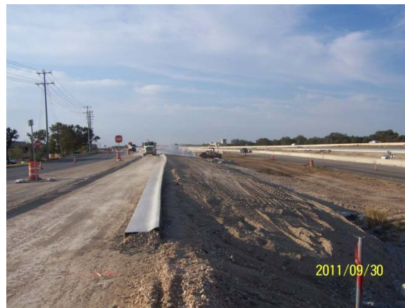
Construction of a new temporary northbound exit ramp for New Hope
