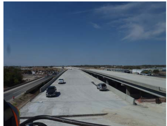
Looking north from the bridges over RM 2243
