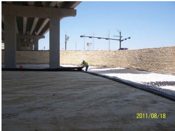
Preparing for rock lining of the stormwater detention pond south of Crystal Falls
