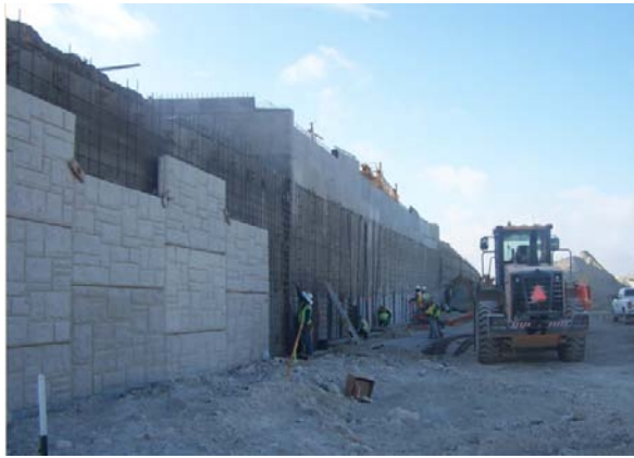
Soil nail wall construction at Scottsdale Drive
