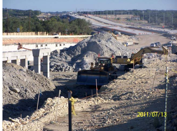
Bridge construction at Scottsdale Drive with Block House Creek beyond
