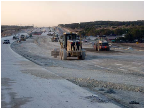
Construction of the main lanes from Hero Way to RM 2243
