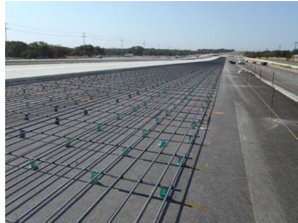
Reinforcing steel for mainlane concrete paving
