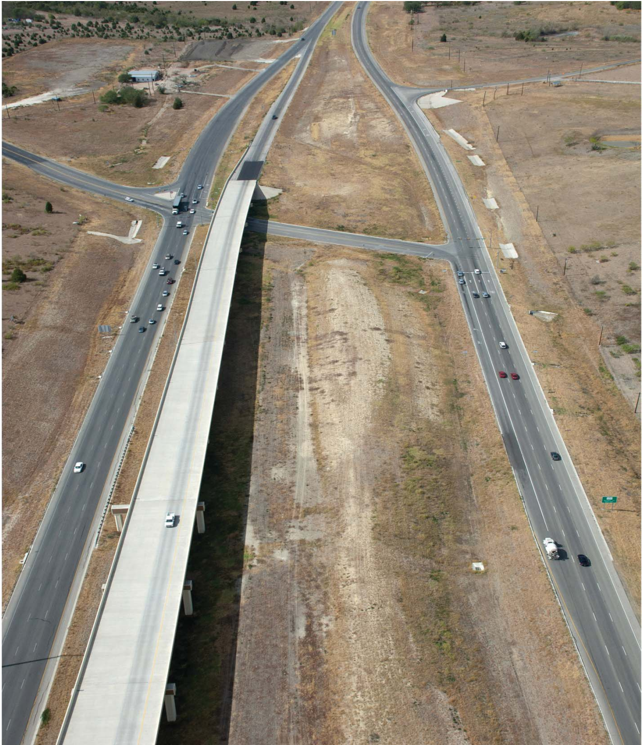
US 290 East at Decker Lane Intersection looking west (Taken 10/7/2011)
