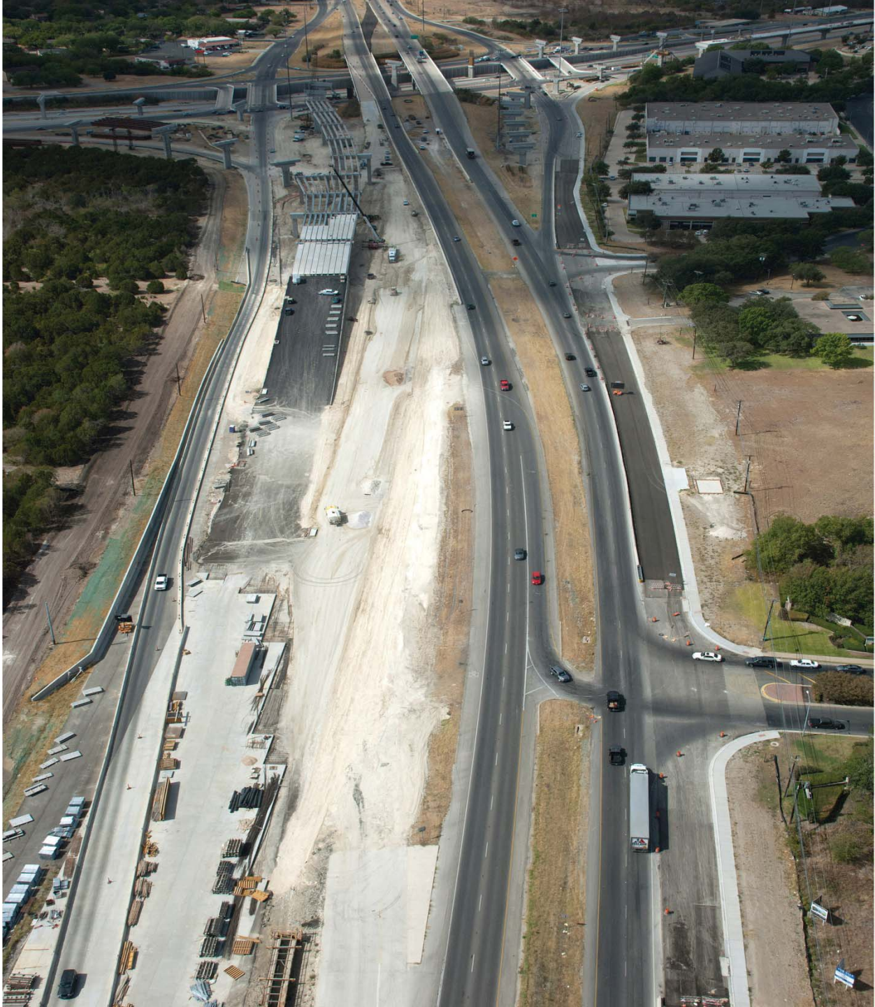
Manor Expressway Phase I Project (Looking West from US 290) (Taken 10/7/2011)
