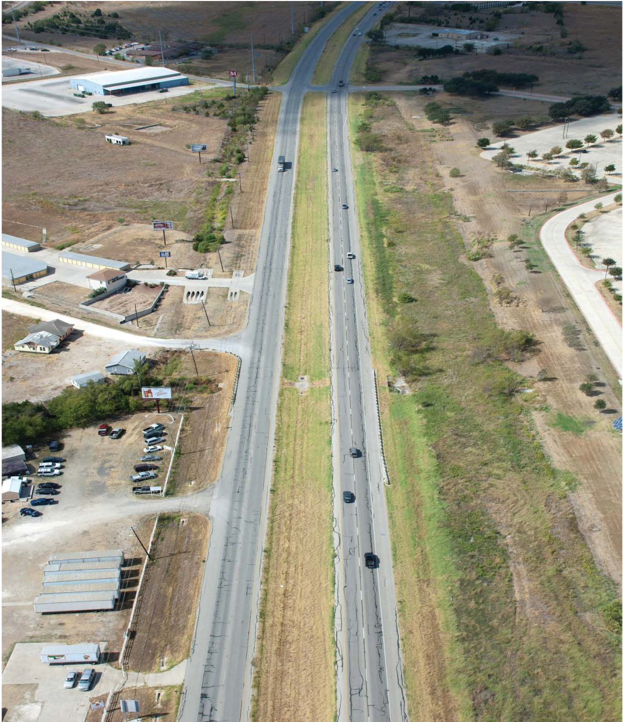
US 290 East at Crofford Lane Intersection looking west (Taken 10/7/2011)
