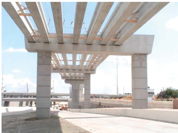
Southbound US 183 on ramp under the South to East Direct Connector (Looking South)
