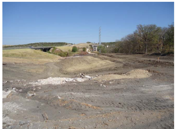
Cleared right-of-way west of MOKAN (Looking East)
