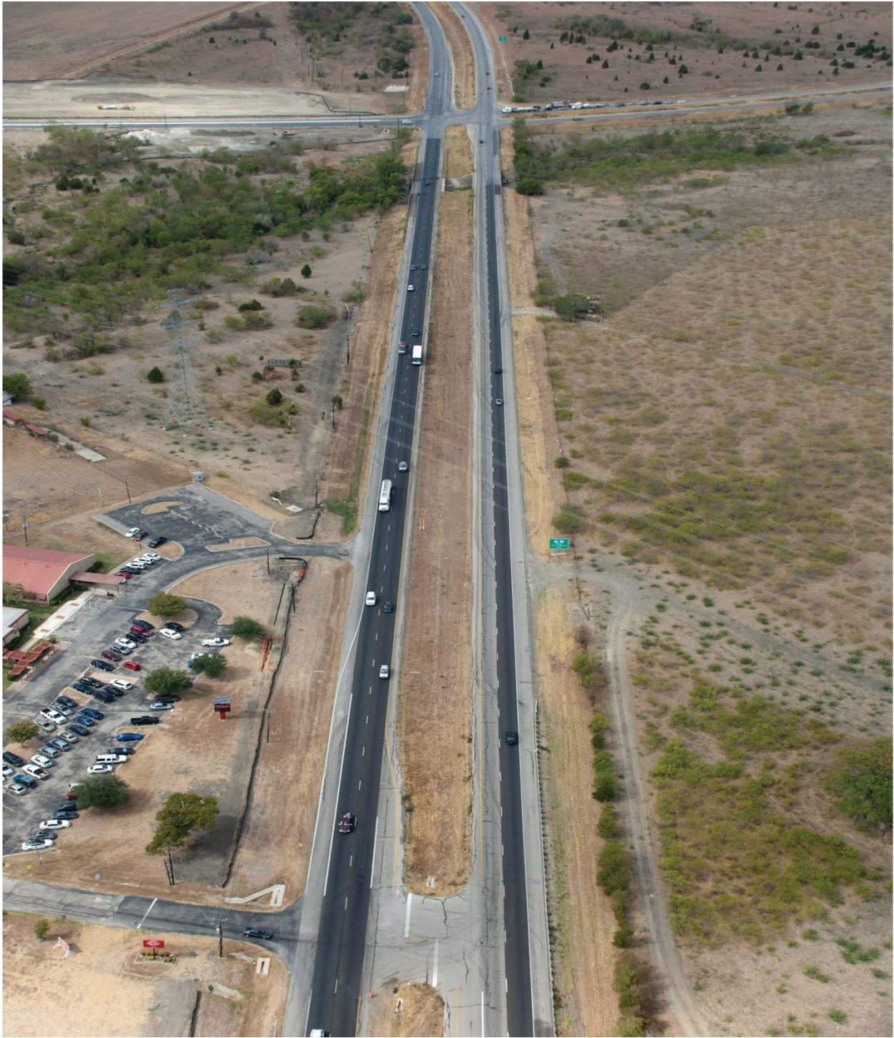
US 290 East looking west from Gilleland Creek (Taken 10/7/2011)
