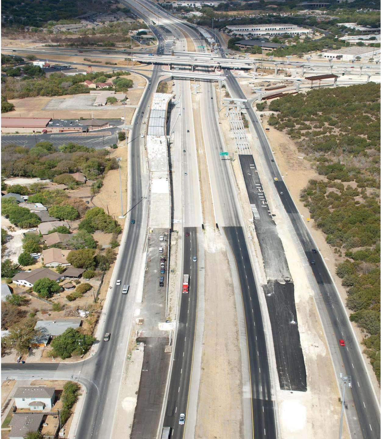
Manor Expressway Phase I Project (Looking North from US 290) (Taken 10/7/2011)
