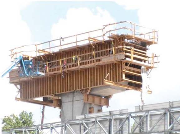
Cap formwork on the West to North Direct Connector (Looking East)
