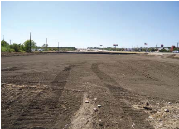
Cleared right-of-way west of Tuscan Way (Looking West)
