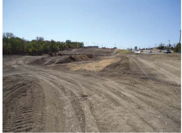
Cleared right-of-way east of Walnut Creek Trib. 5 (Looking West)
