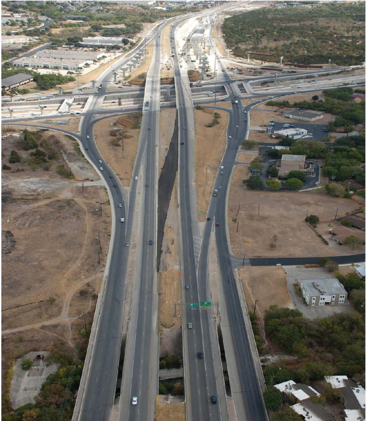
Manor Expressway Phase I Project (Looking East from US 290) (Taken 10/7/2011)
