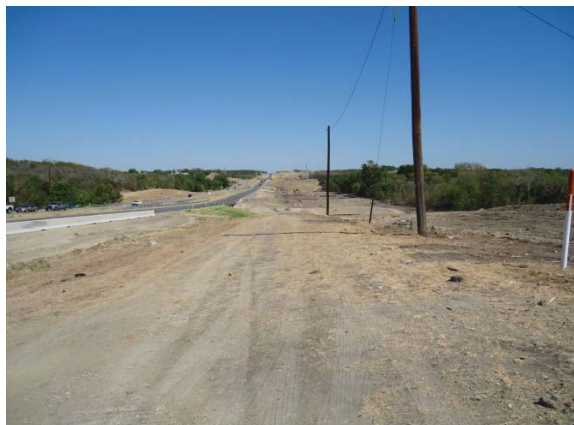
Cleared right-of-way east of Ferguson Lane (Looking East)
