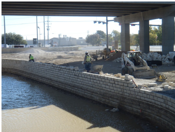
Stone masonry at storm water detention pond
