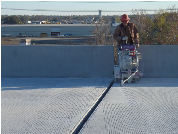
Sawcutting grooves on the bridge over RM 2243
