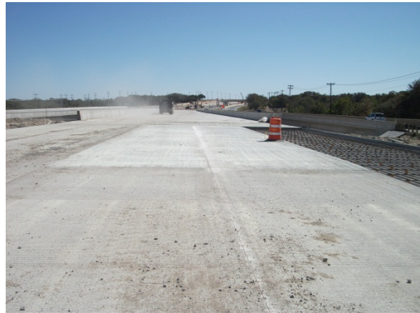
View of the southbound mainlanes at the Block House Creek bridges
