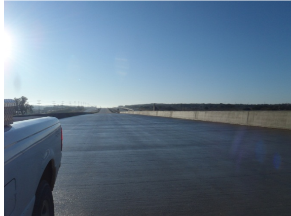
Northbound bridge over RM 2243 looking south
