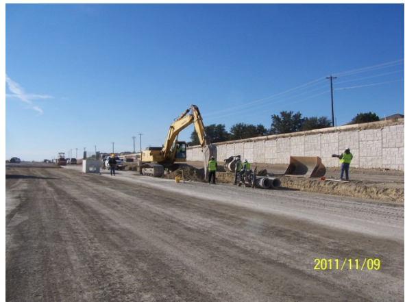
Installing the underground storm drain system south of Scottsdale Drive
