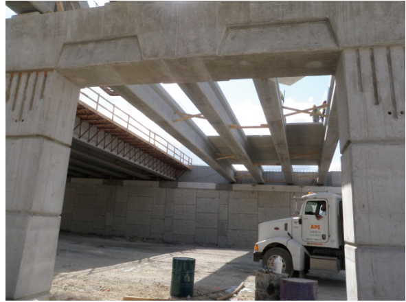
Placing precast concrete panels at a Scottsdale Drive turnaround bridge
