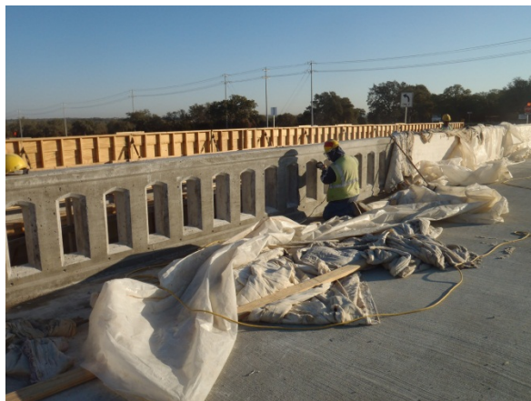
Constructing the aesthetic bridge railing at Scottsdale Drive
