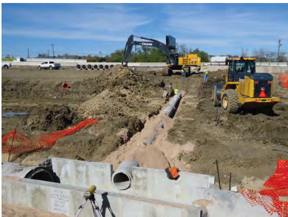
Reinforced concrete pipe installation (Looking North)
