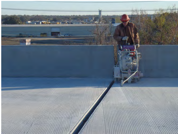
Sawcutting grooves on the bridge over RM 2243
