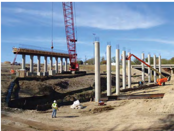
Bridges at Walnut Creek Tributary #5 (Looking North)
