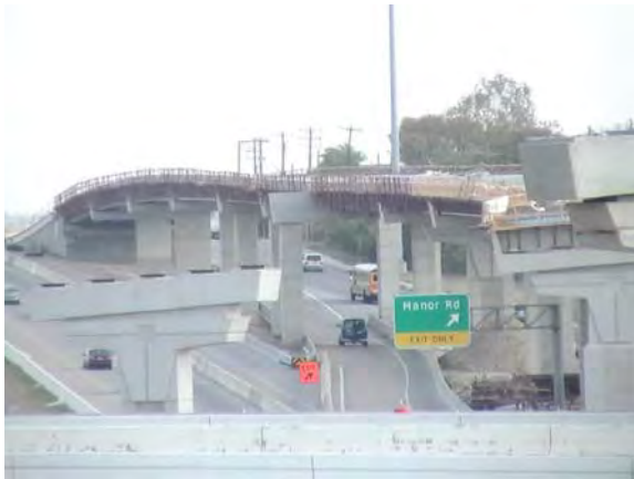
Deck construction along East to South Direct Connector (Looking South)
