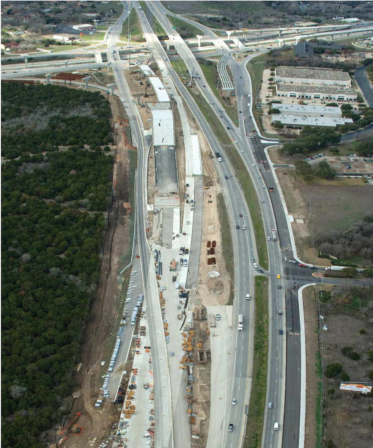
Manor Expressway Phase I Project (Looking West from US 290) (Taken 1/10/2012)
