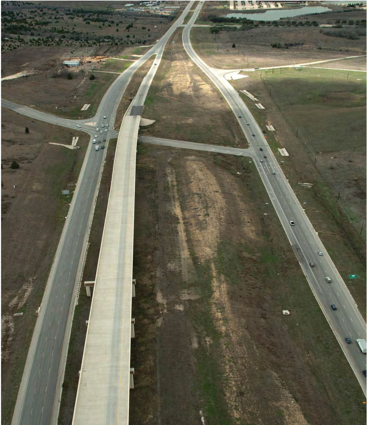
US 290 East at Decker Lane Intersection looking west (Taken 1/10/2012)
