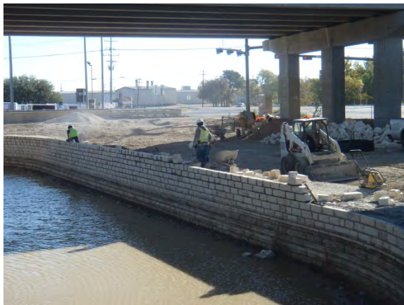
Stone masonry at storm water detention pond
