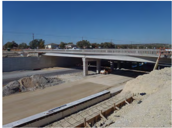
View of the Scottsdale Drive bridges and the 183A mainlanes below
