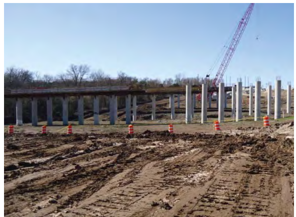
Bridges at Walnut Creek Tributary #5 (Looking East)
