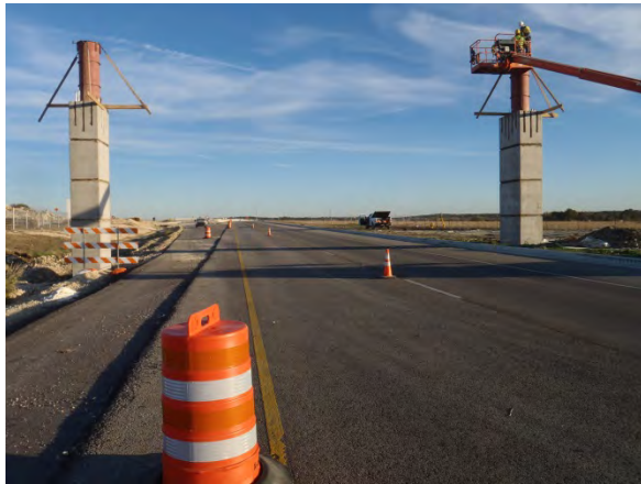
Overhead sign support columns spanning the frontage roads at the project's northern end
