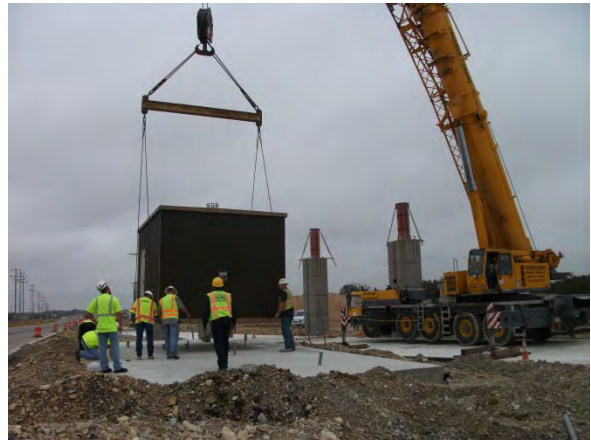
Precast concrete building for tolling equipment at the Crystal Falls on ramp
