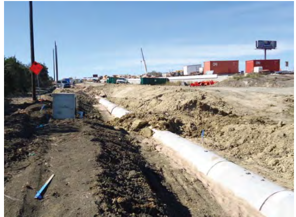
Reinforced concrete pipe installation (Looking East)
