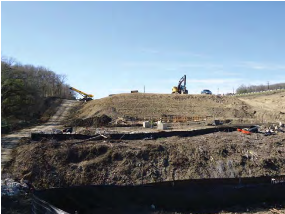
Earthwork embankment west of MOKAN (Looking East)
