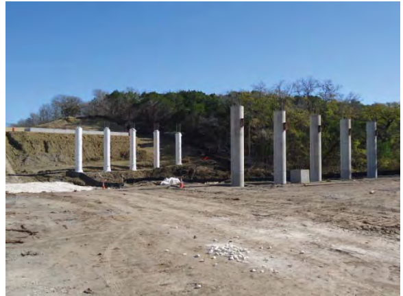
Drilled shaft extensions for bridge at Walnut Creek (Looking West)
