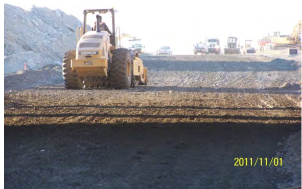
Compacting the final lift of soil on the 183A mainlanes south of Scottsdale Drive
