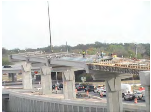
Beams constructed on South to East Direct Connector (Looking South)
