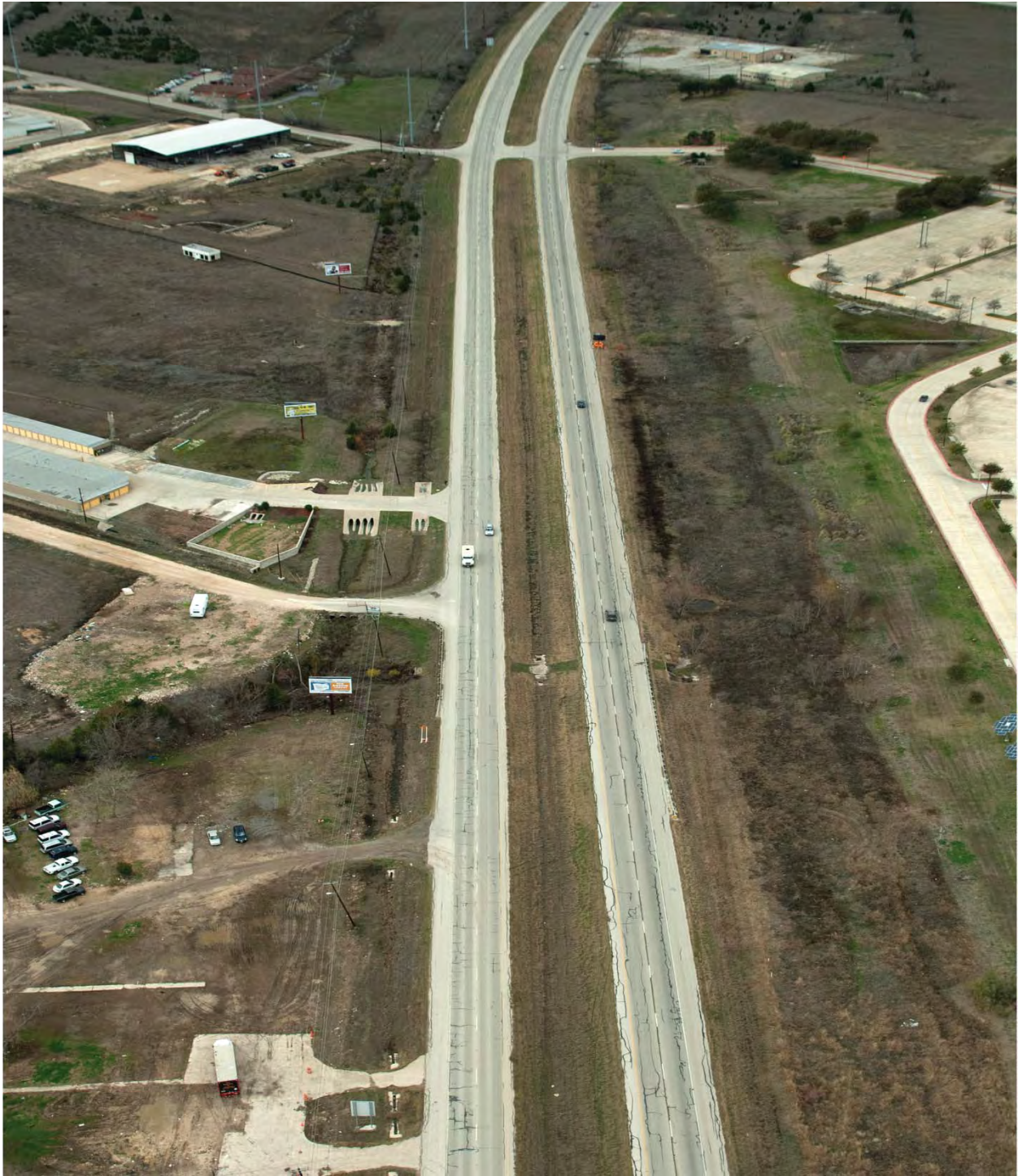
US 290 East at Crofford Lane Intersection looking west (Taken 1/10/2012)
