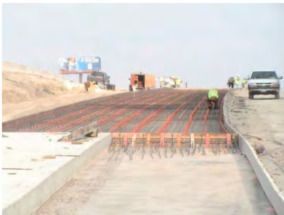
Eastbound main lane roadway construction (Looking East)
