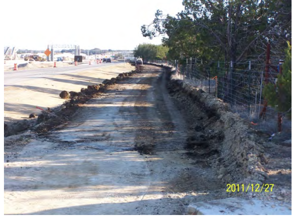
Construction of the Phase II Shared Use Path
