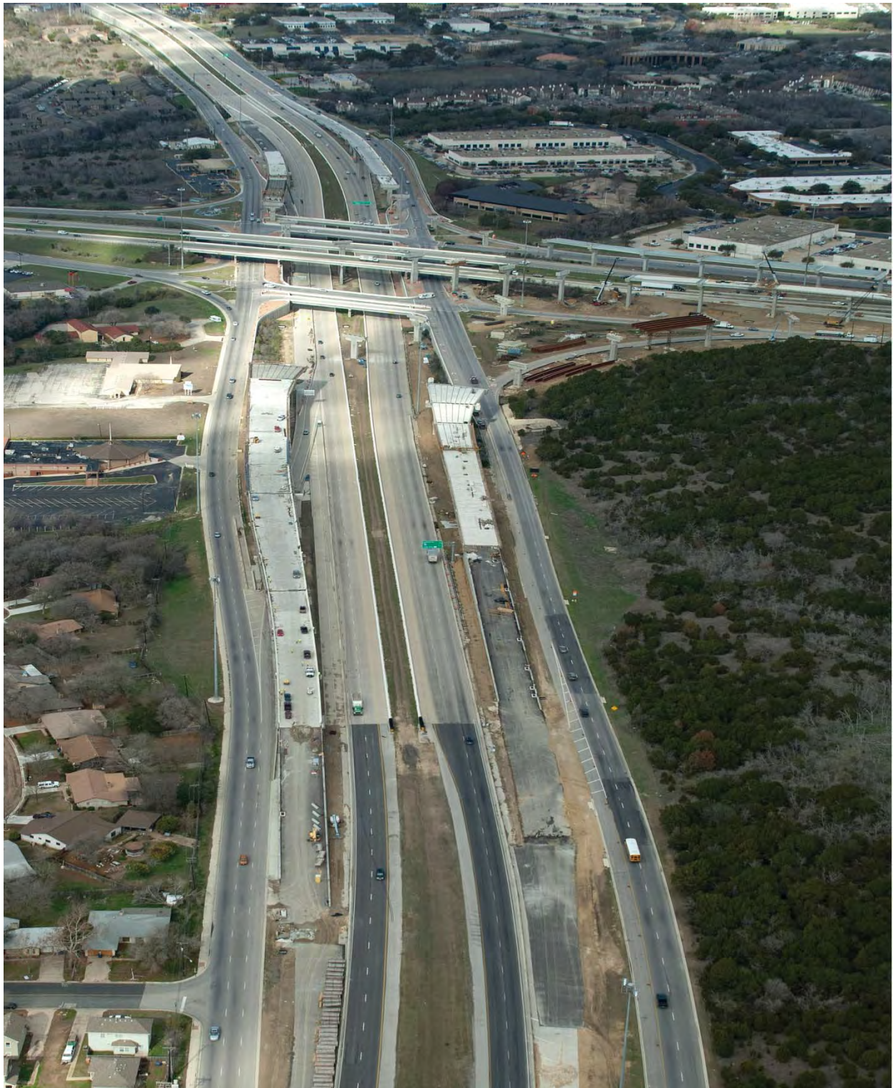
Manor Expressway Phase I Project (Looking North from US 183) (Taken 1/10/2012)
