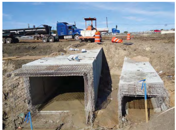
Box culverts "B1" & "B2" under construction (Looking North)
