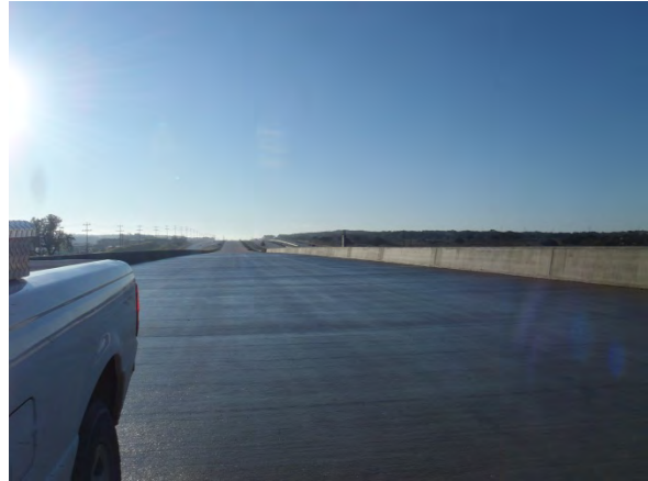
Northbound bridge over RM 2243 looking south
