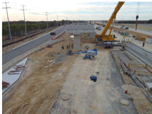
View from end of future bridge of braided ramp north of New Hope Drive
