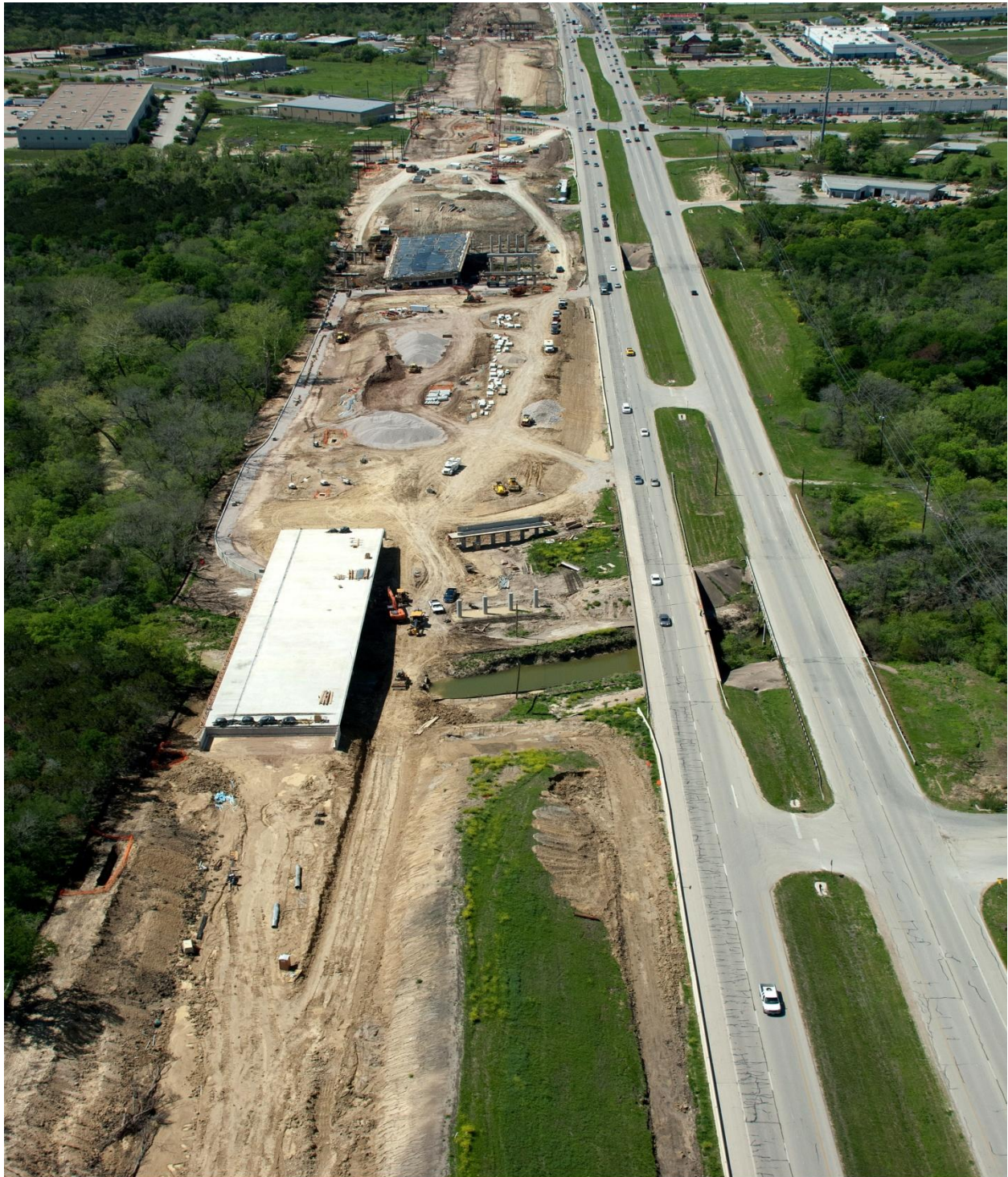
US 290 East at Chimney Hill Blvd looking west (Taken 3/02/2012)
