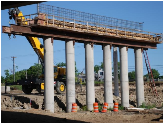
Construction of abutment at Trib #5 eastbound mainlane bridge (Looking West)
