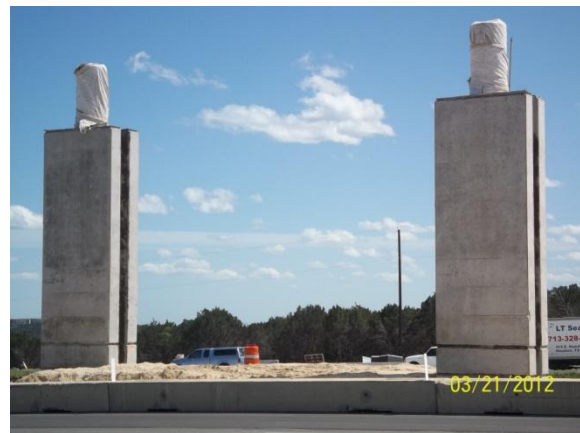
West to North Toll Gantry Columns (Looking South)
