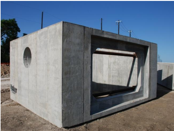
Manhole for Line D prior to installation (Looking West)
