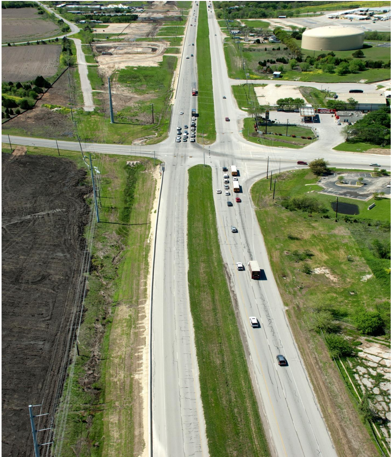
US 290 East at Giles Road Intersection looking west (Taken 3/02/2012)
