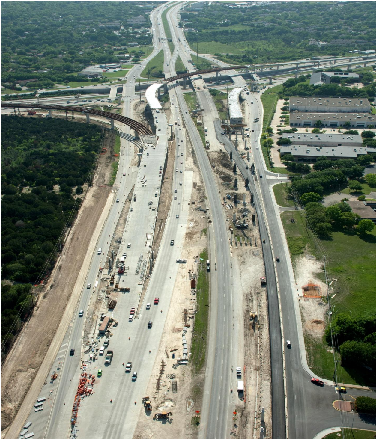
Manor Expressway Phase I Project (Looking West from US 290) (Taken 4/05/2012)
