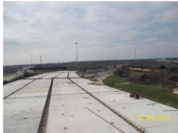
Bridge Deck Construction along West to North Direct Connector (Looking West)
