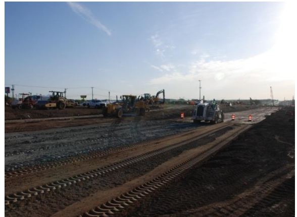
Placing cement-treated embankment for the eastbound frontage road (Looking East)
