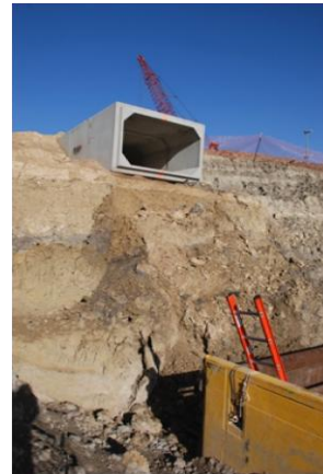
Installation of Culvert D near large manhole (Looking West)
