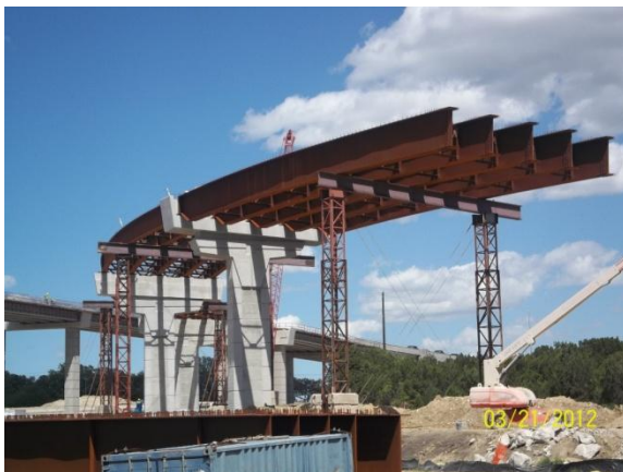
Steel Erection on the North to East Direct Connector (Looking East)
