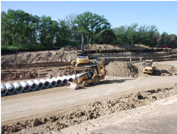
Eastbound frontage road storm sewer, Line I (Looking South)
