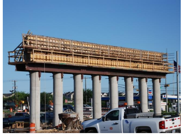
Construction of abutment at Tuscany Way eastbound mainlane bridge (Looking West)
