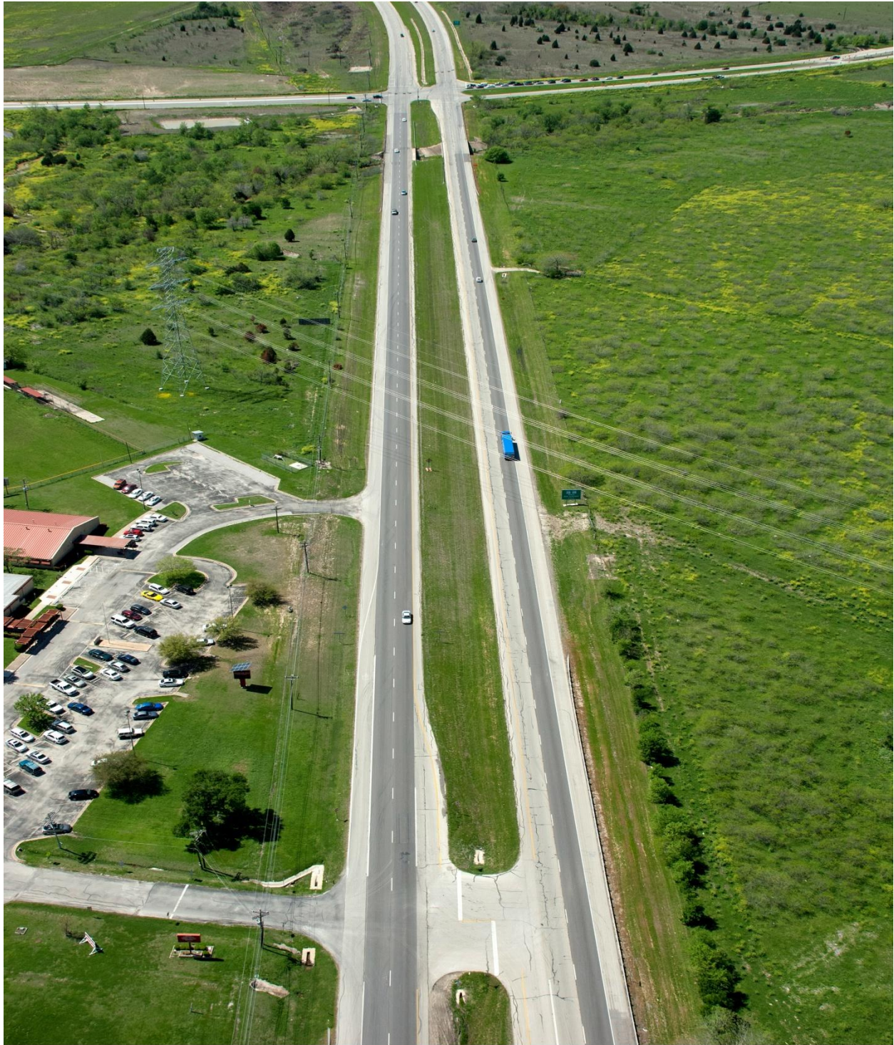
US 290 East looking west from Gilleland Creek (Taken 3/02/2012)
