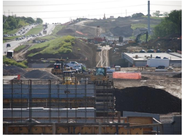
Overall view of progress from east of Ferguson Cutoff (Looking East)
