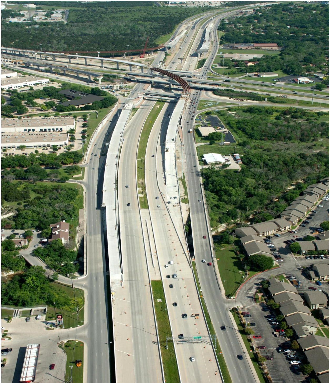
Manor Expressway Phase I Project (Looking South from US 183) (Taken 4/05/2012)
