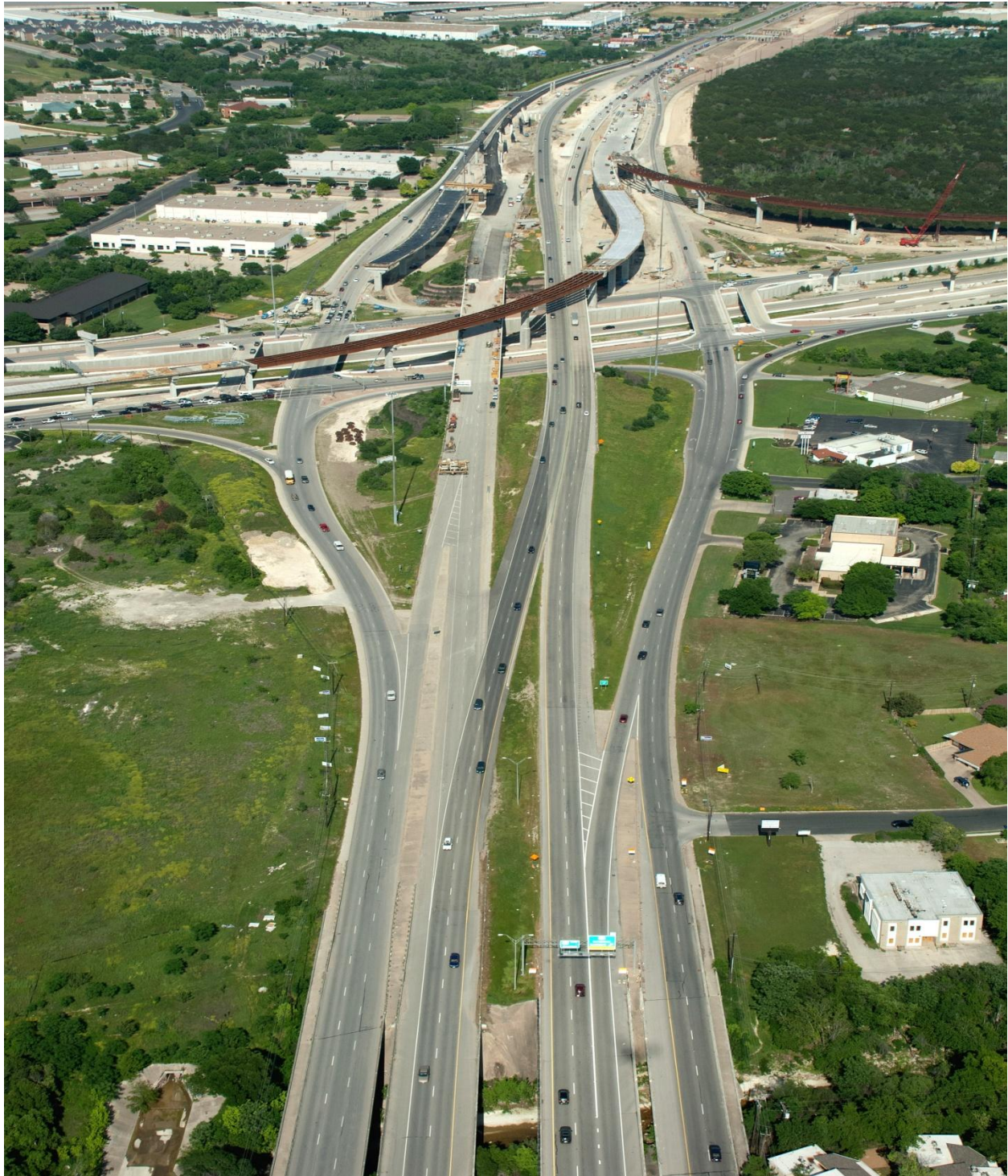
Manor Expressway Phase I Project (Looking East from US 290) (Taken 4/05/2012)
