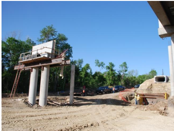
Construction of shared use path bridge at Trib #5 (Looking West)
