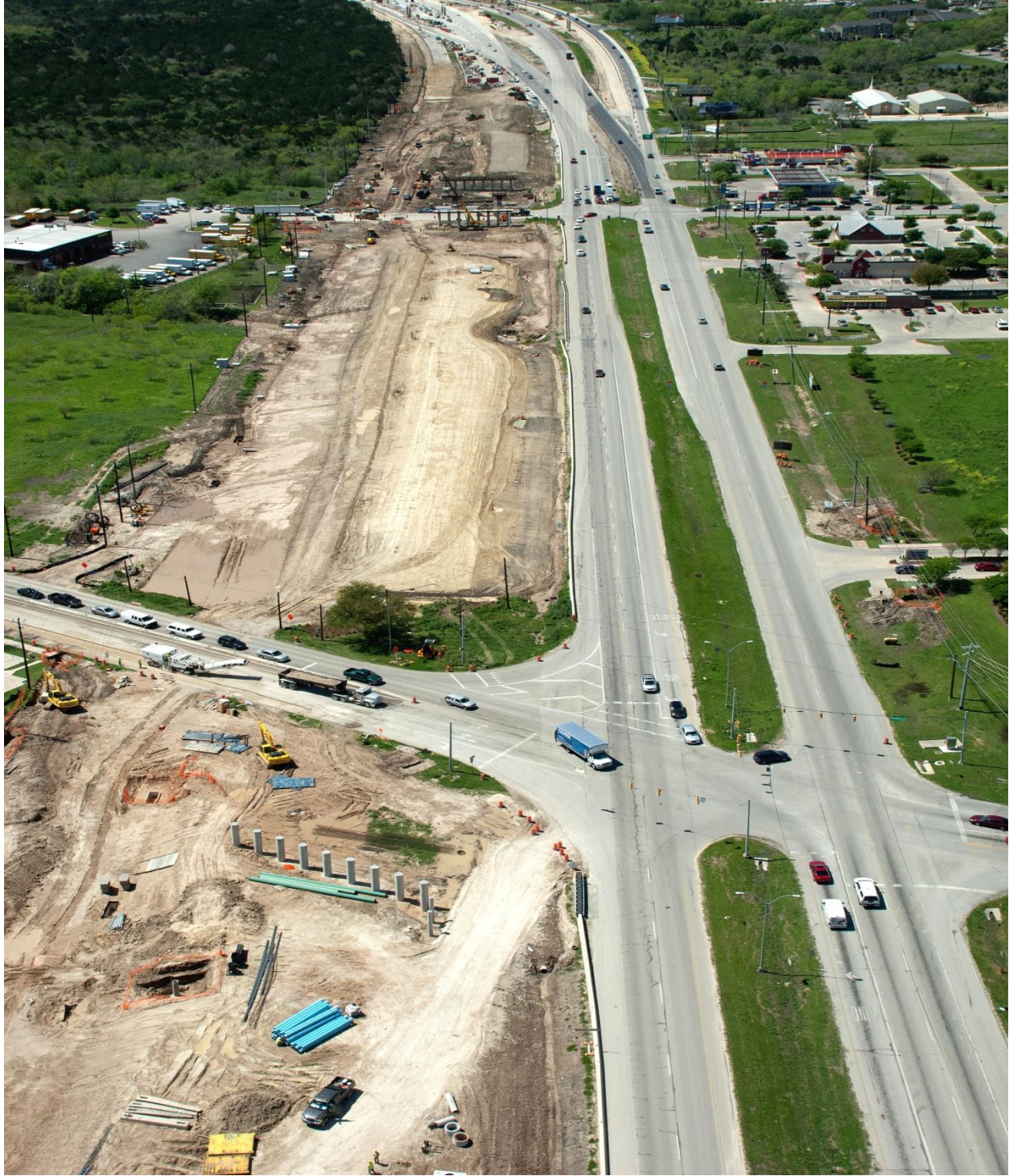
US 290 East at Springdale Road looking west (Taken 3/02/2012)
