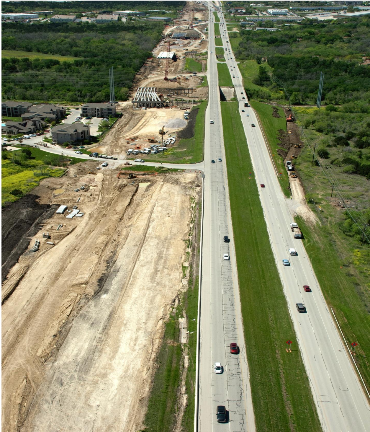
US 290 East looking west at Mokon Crossing (Taken 3/02/2012)
