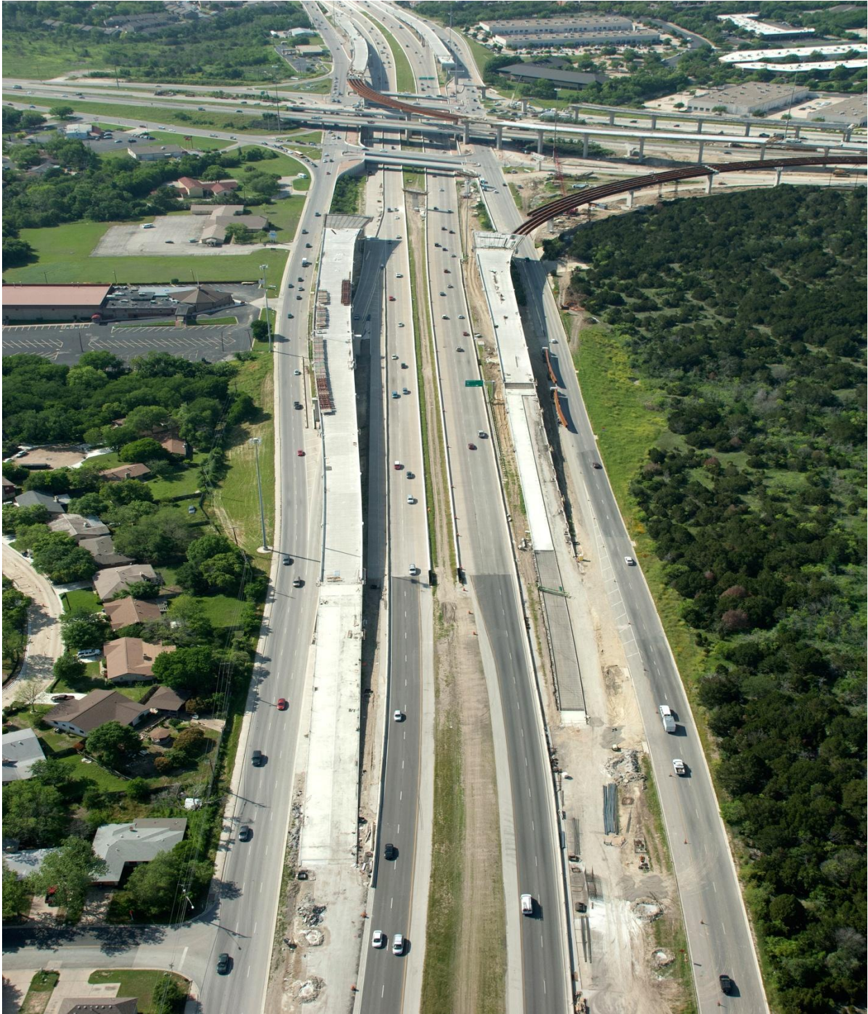
Manor Expressway Phase I Project (Looking North from US 183) (Taken 4/05/2012)
