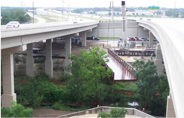
Installation of 183A Shared Use Path Pedestrian Bridge - opening September 2012
