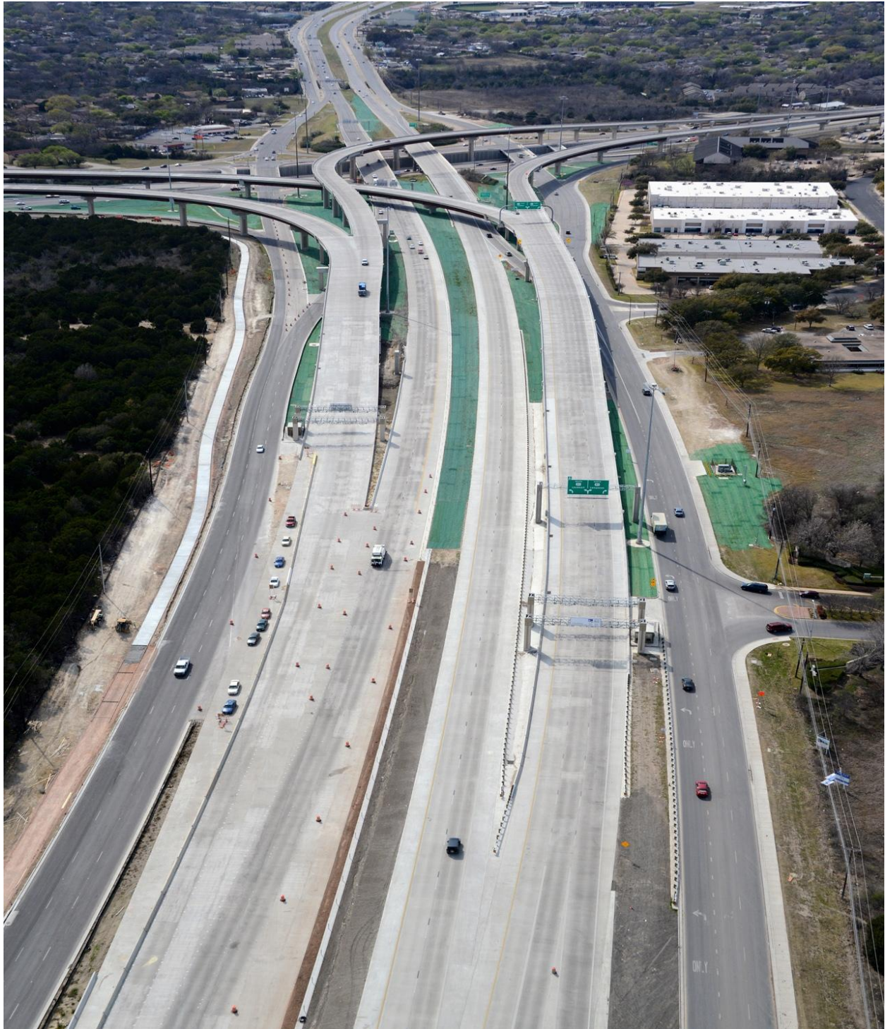
Manor Expressway Phase I Project (Looking West from US 290) (Taken 3/7/2013)
