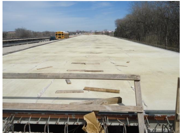
Construction of the eastbound frontage road at Gilleland Creek (Looking East)
