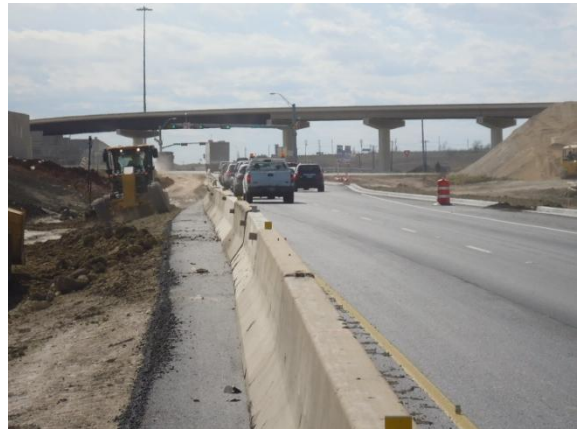
Westbound frontage road between Trib #1C and SH 130 (Looking West)
