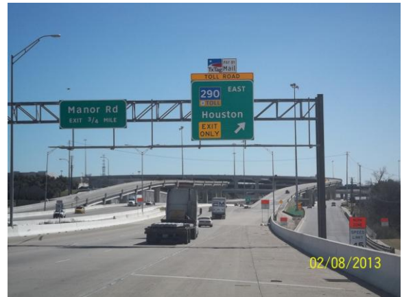
South to East Direct Connector Exit from U.S. 183 Southbound (Looking Southeast)
