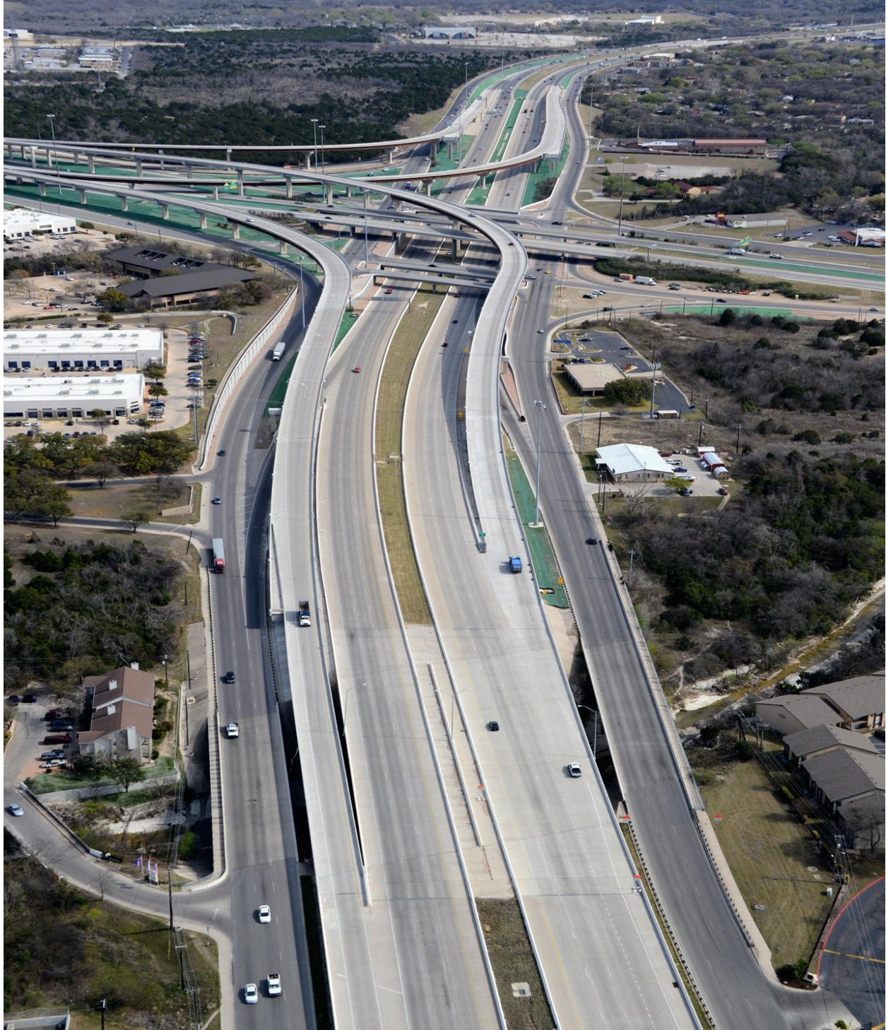
Manor Expressway Phase I Project (Looking South from US 183) (Taken 3/7/2013)
