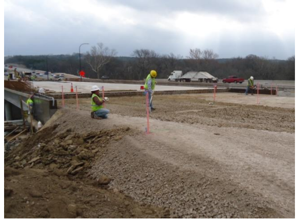
Approach slab construction for the EBML bridge at Trib #5 (Looking Southeast)
