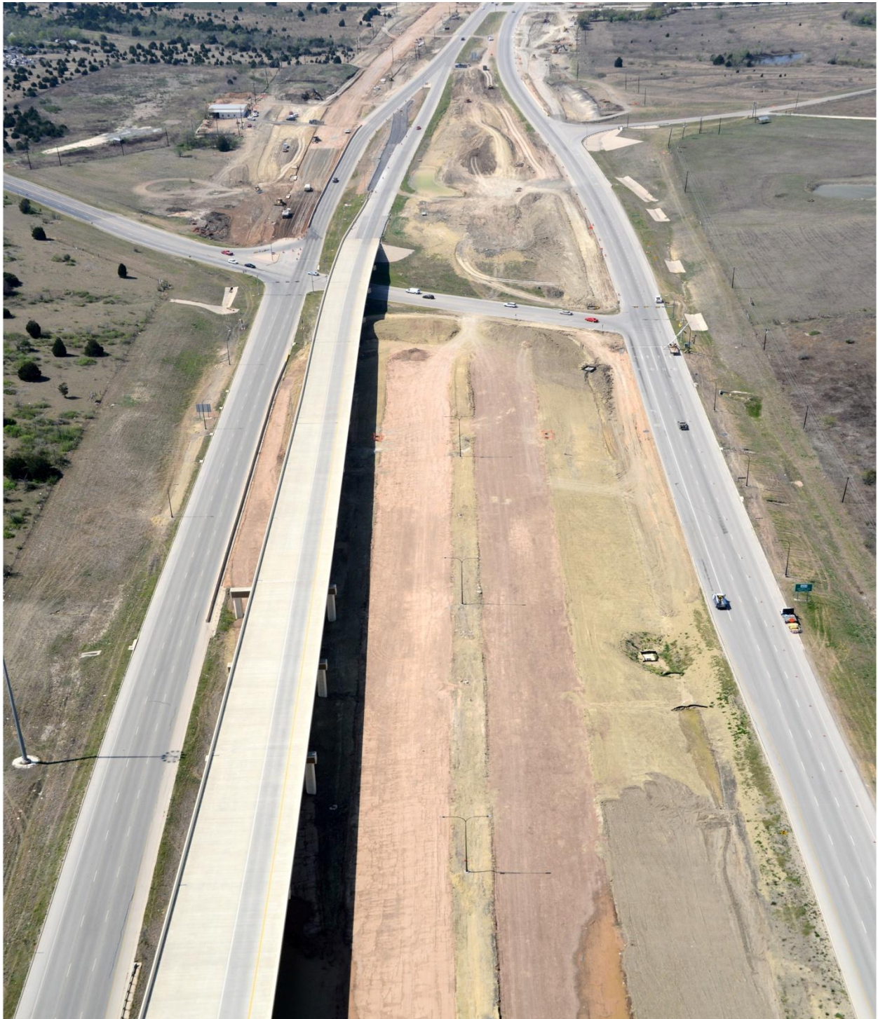
US 290 East at Decker Lane Intersection looking west (Taken 3/19/2013)
