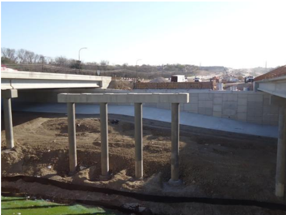
Construction of the westbound mainlane bridge at Trib #5 (Looking East)
