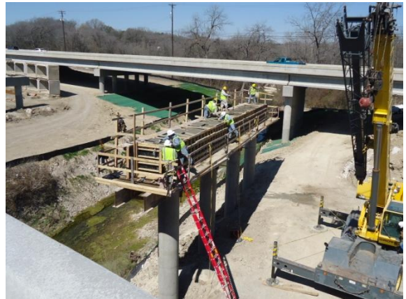
Construction of the westbound mainlane bridge at Walnut Creek (Looking Northwest)
