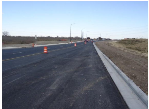
Westbound frontage road east of SH 130 (Looking East)
