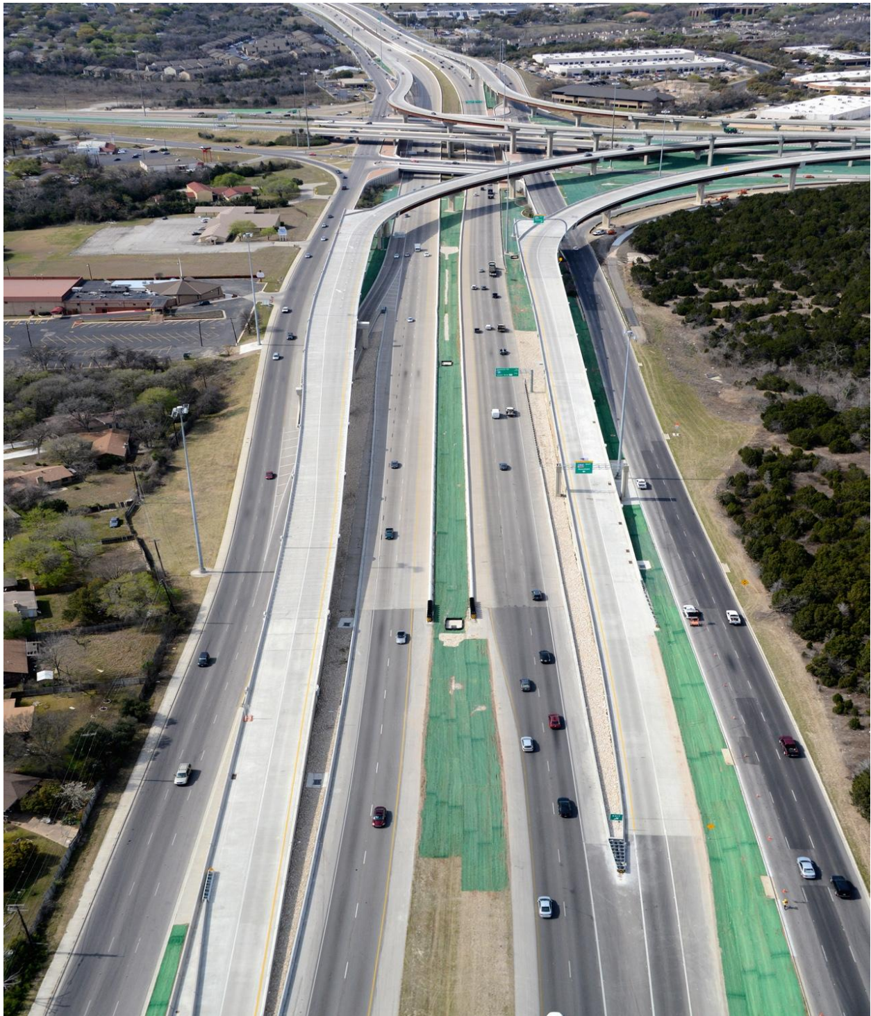
Manor Expressway Phase I Project (Looking North from US 183) (Taken 3/7/2013)
