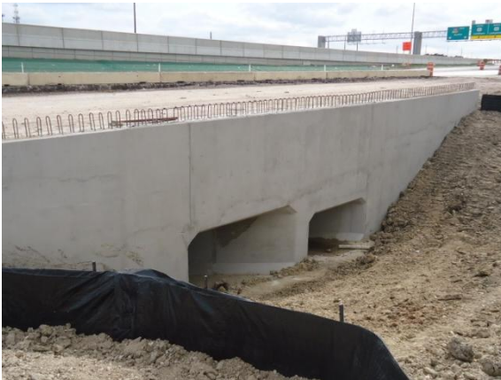
Culvert A & A1 Headwall for the Westbound Frontage Road (Looking Southwest)
