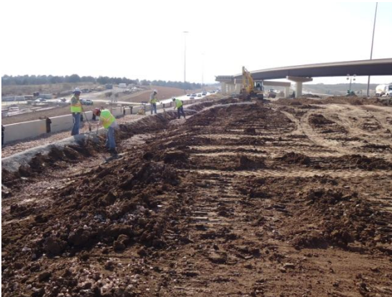
Embankment operations on the eastbound mainlanes at SH 130 (Looking West)
