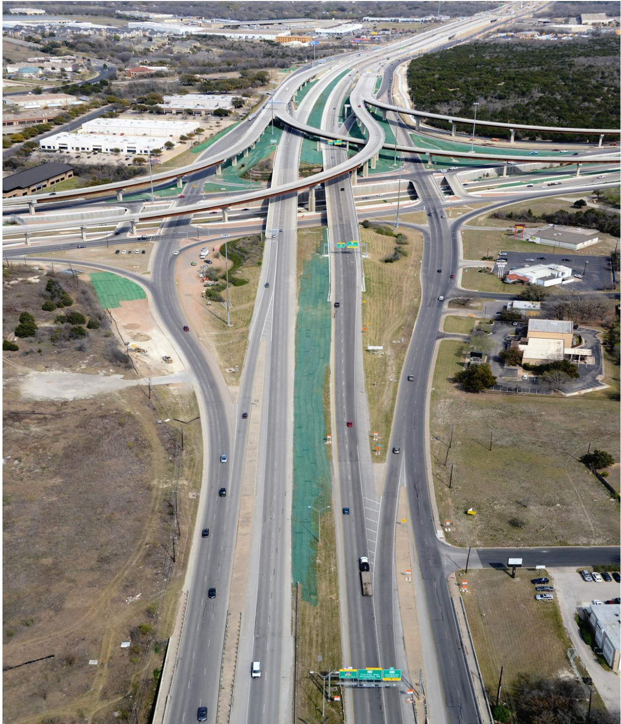
Manor Expressway Phase I Project (Looking East from US 290) (Taken 3/7/2013)
