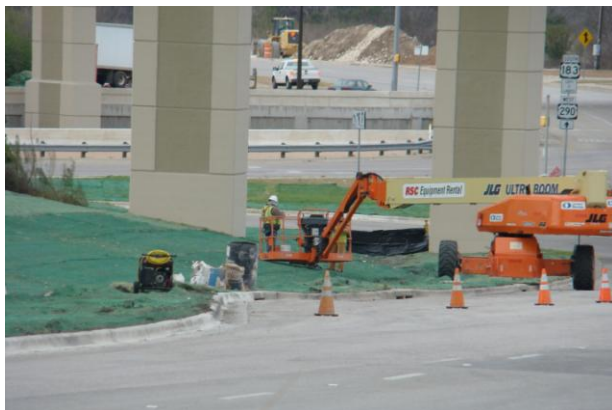
Repair of minor aesthetic blemishes on the West to South direct connector (Looking West)
