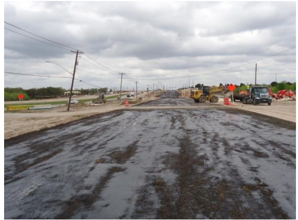
Placement of prime coat on the cement-treated base (Looking East)
