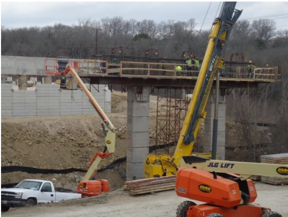
Construction of the westbound frontage road bridge at MOKAN (Looking Northwest)
