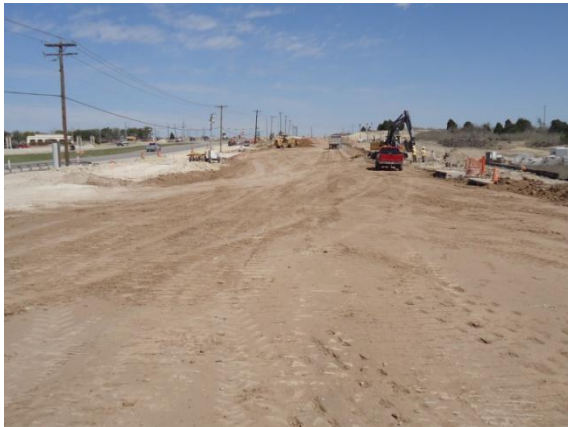
Embankment for the eastbound frontage road near Harris Branch Pkwy (Looking East)
