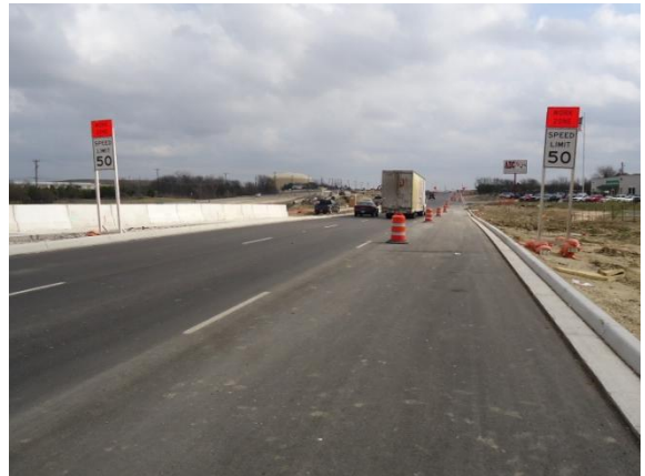
Eastbound frontage road opened to traffic near Arterial "A" (Looking East)
