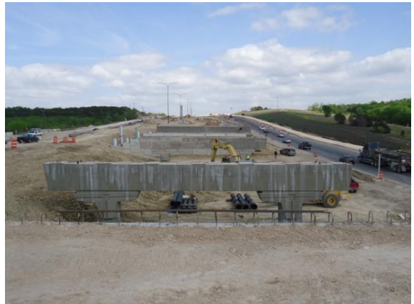
Construction of the eastbound mainlane bridge at Arterial "A" (Looking East)
