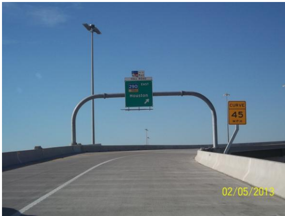
Completed North to East Direct Connector (Looking Northwest)
