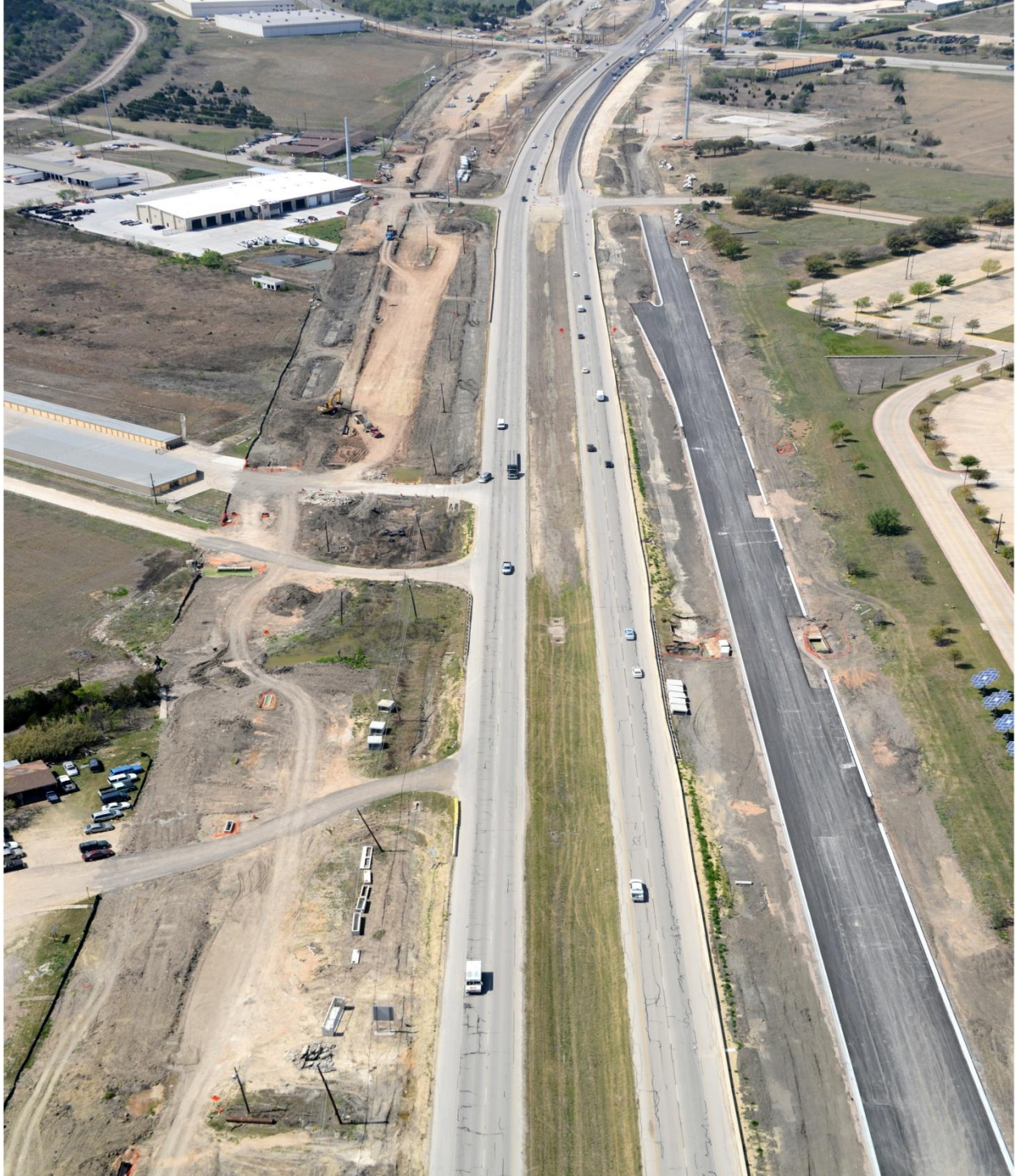
US 290 East at Crofford Lane Intersection looking west (Taken 3/19/2013)
