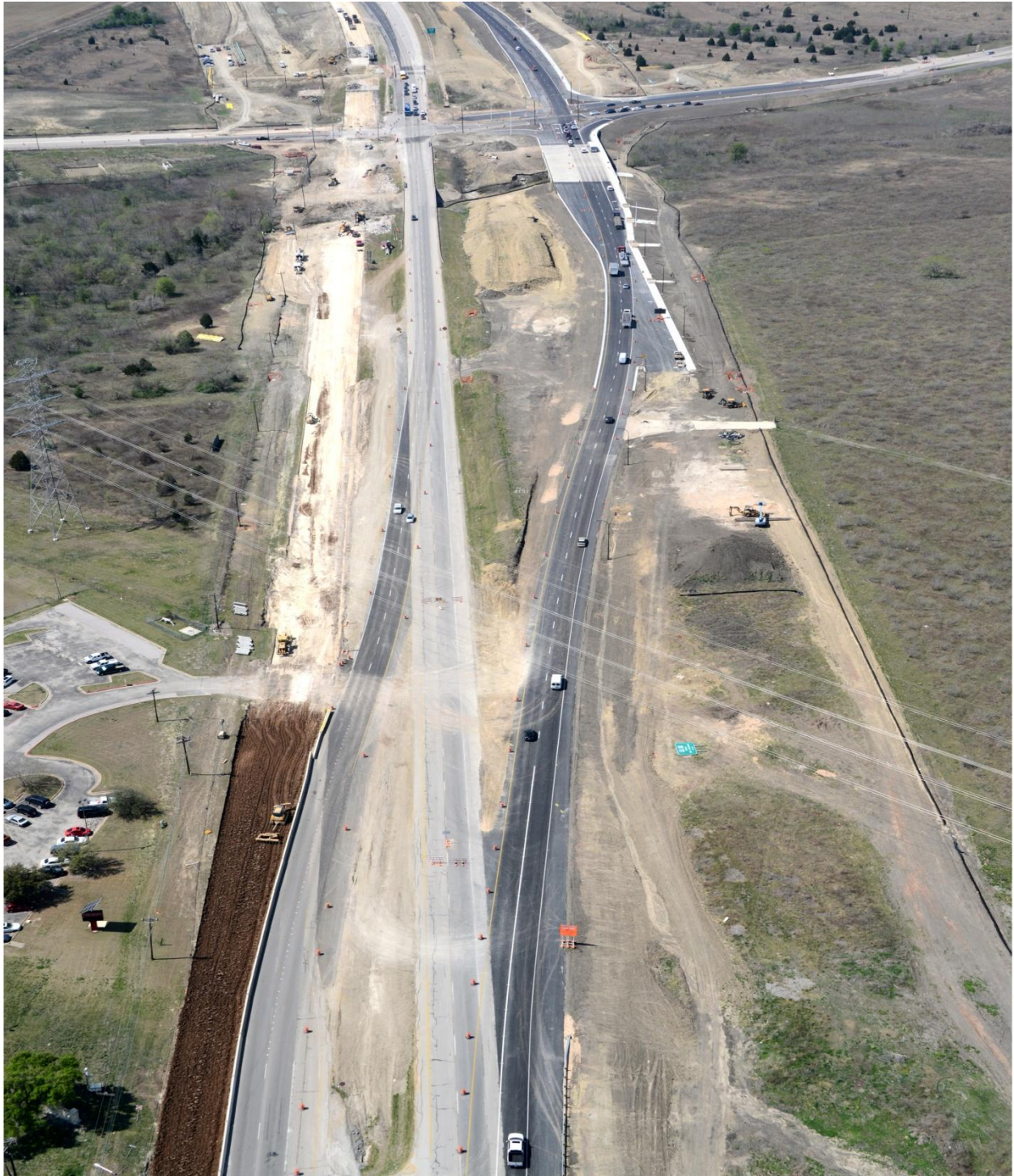
US 290 East looking west from Gilleland Creek (Taken 3/19/2013)
