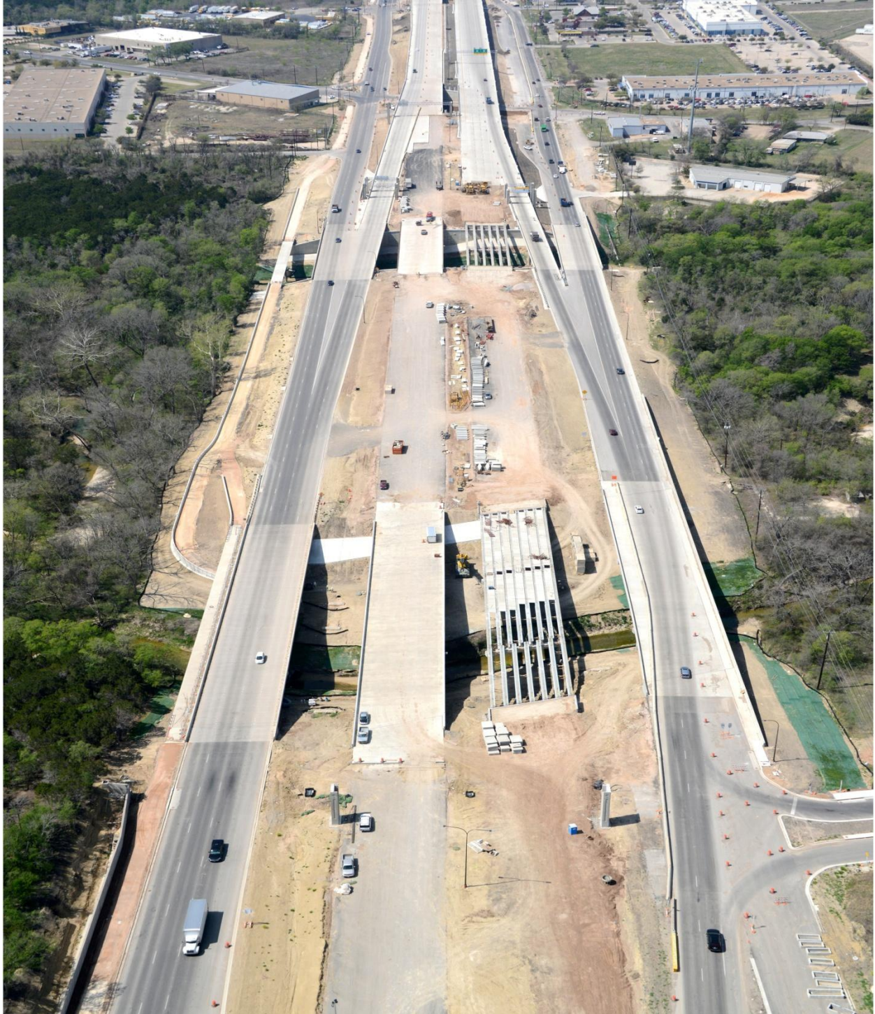
US 290 East at Chimney Hill Blvd looking west (Taken 3/19/2013)
