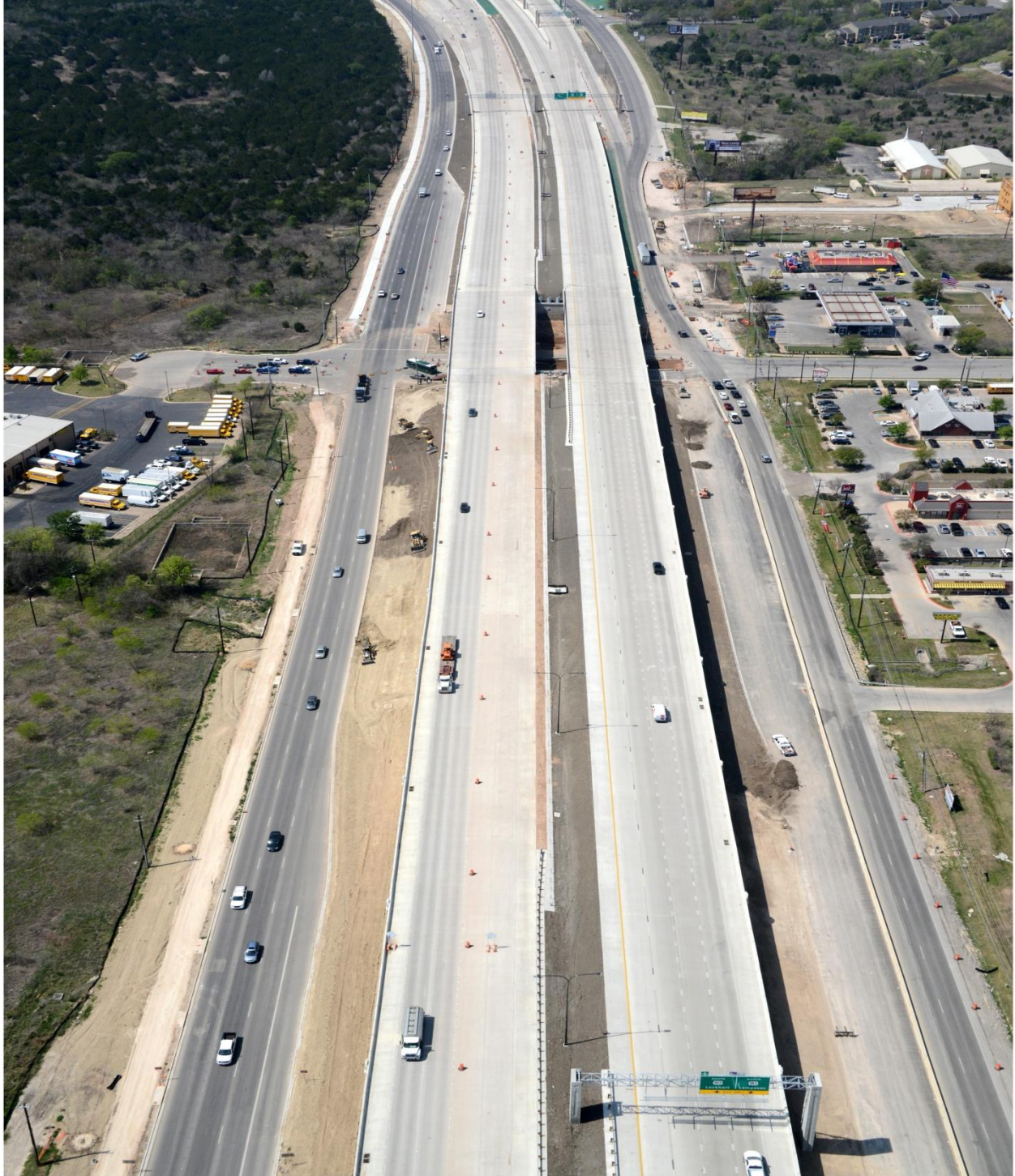
US 290 East at Springdale Road looking west (Taken 3/19/2013)
