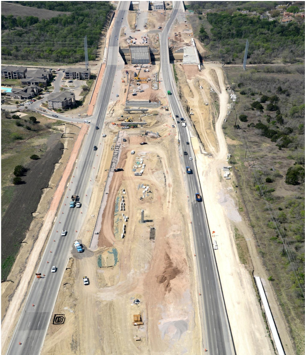
US 290 East looking west at Mokon Crossing (Taken 3/19/2013)
