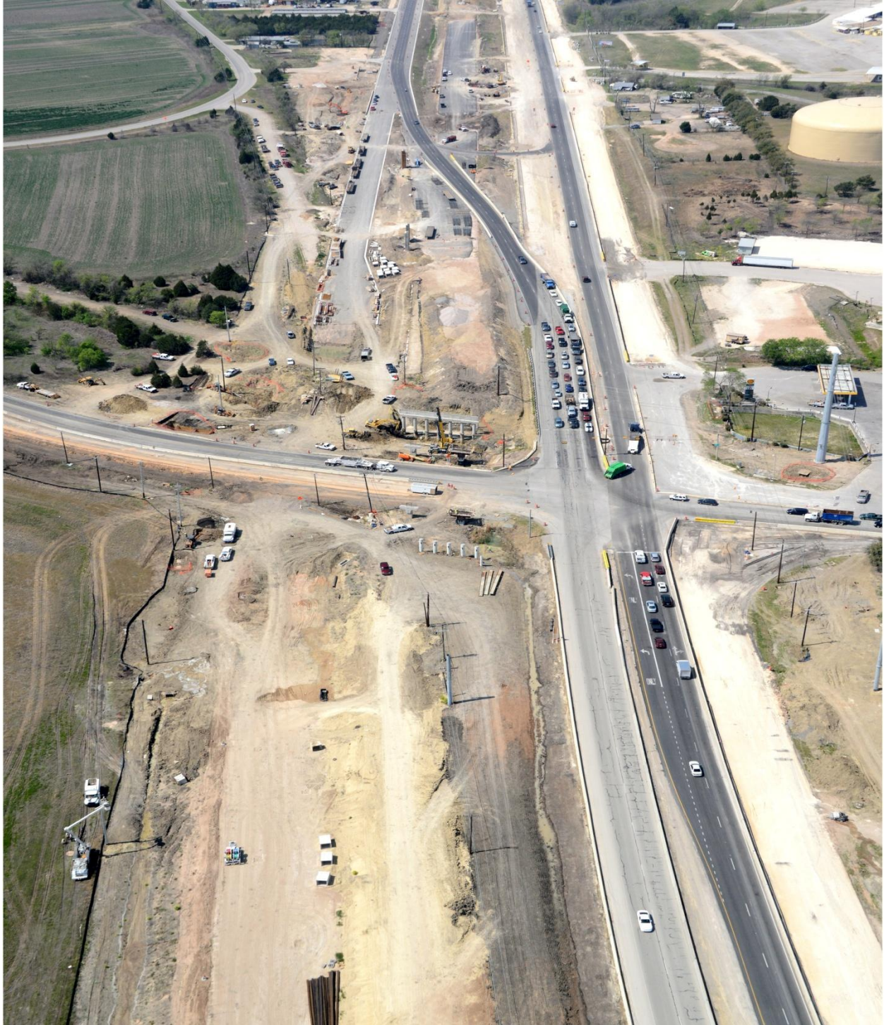
US 290 East at Giles Road Intersection looking west (Taken 3/19/2013)
