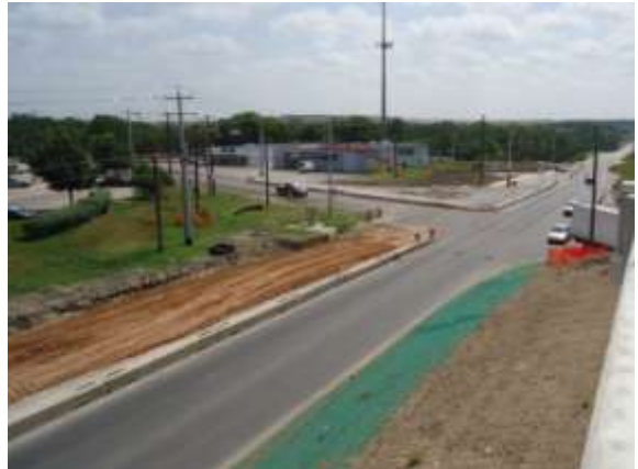
Westbound frontage road construction at Springdale Road (Looking Northeast)
