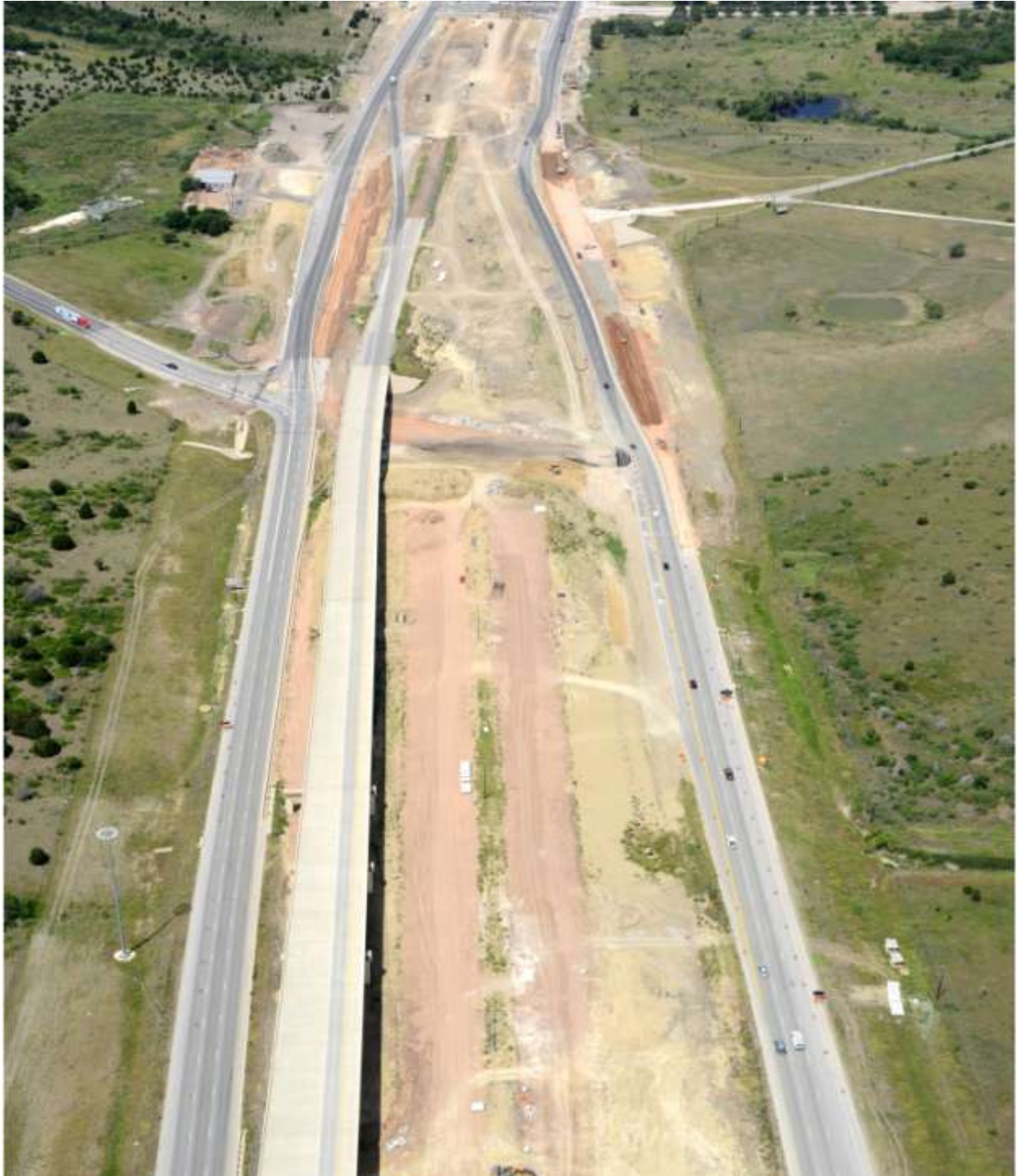
US 290 East at Decker Lane Intersection looking west (Taken 6/24/2013)
