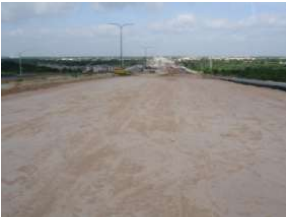
Subgrade for the westbound mainlanes east of Arterial "A" (Looking West)
