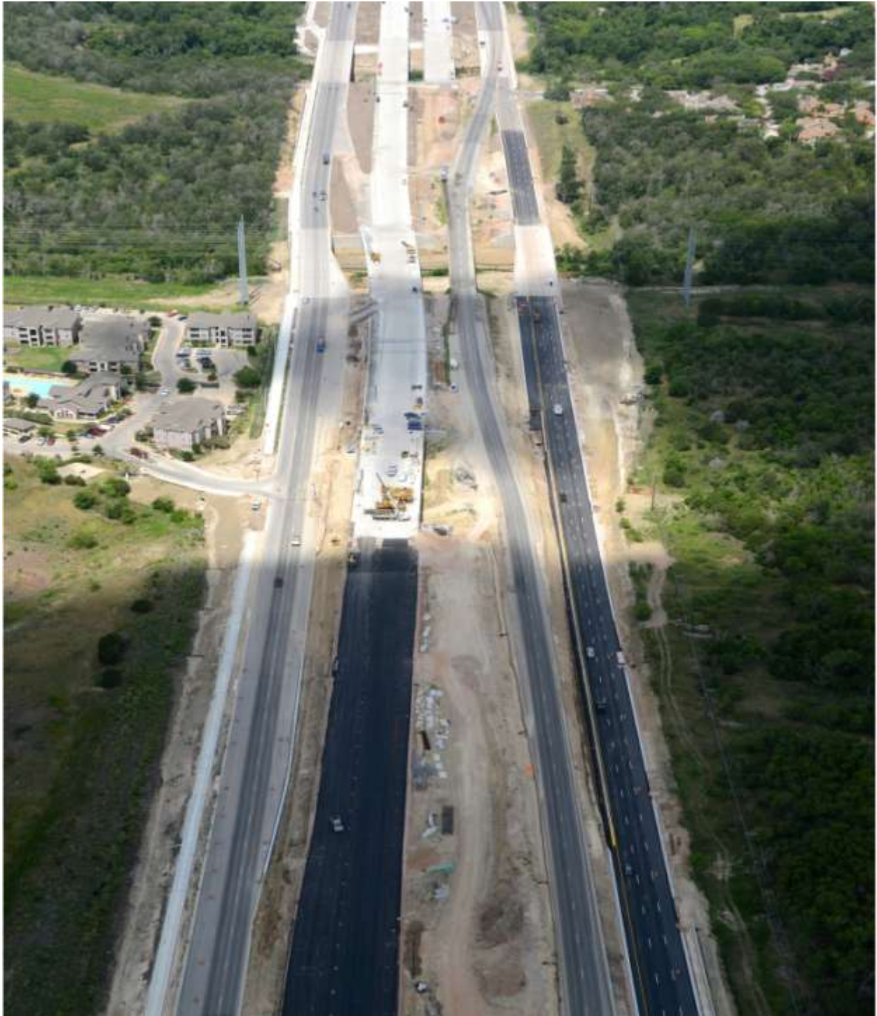
US 290 East looking west at Mokan Crossing (Taken 6/24/2013)
