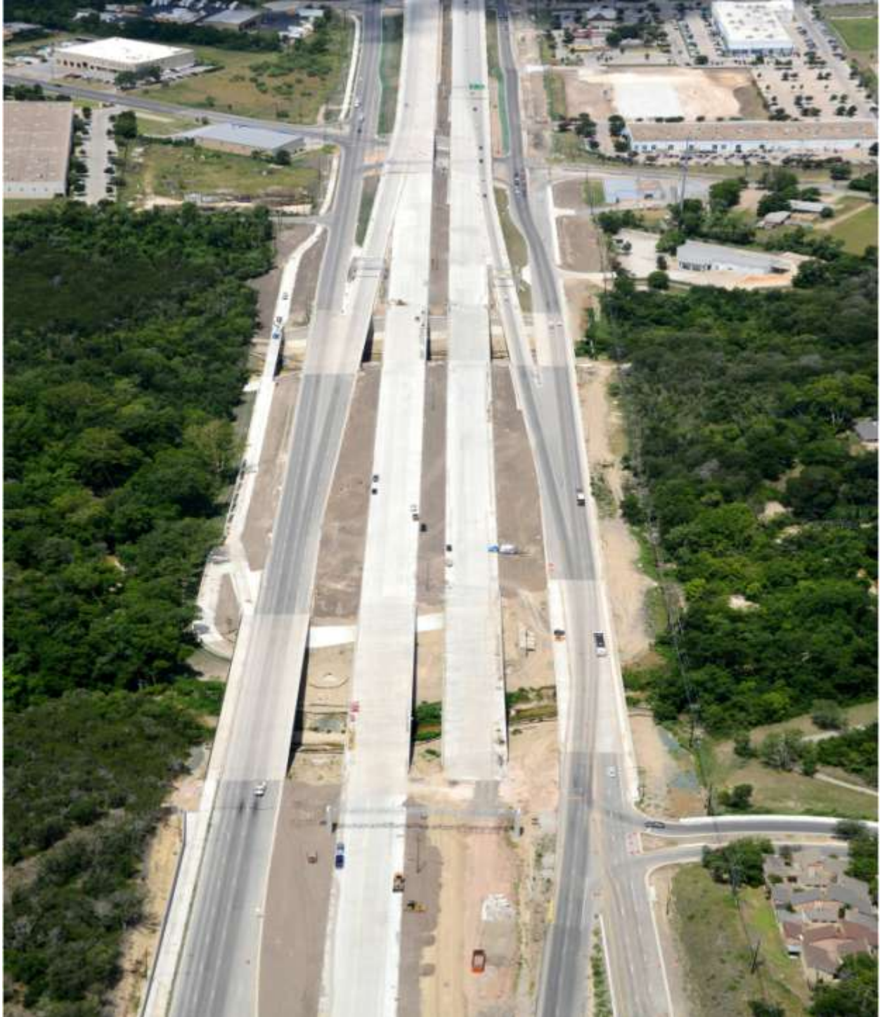
US 290 East at Chimney Hill Blvd looking west (Taken 6/24/2013)
