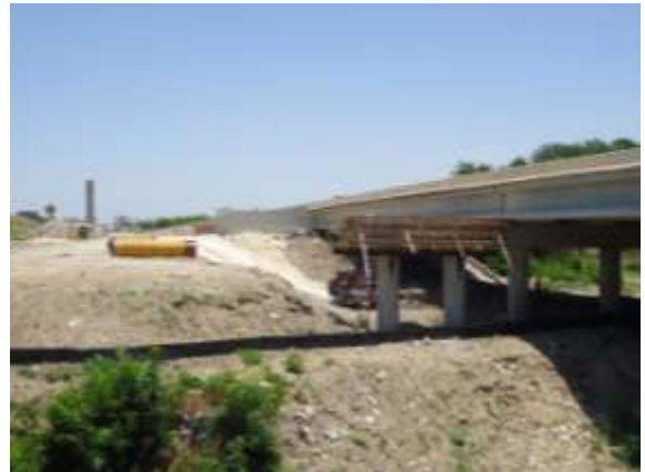
Construction of eastbound frontage road bridge at Gilleland Creek (Looking East)
