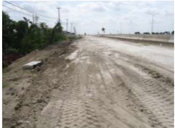
Westbound frontage road construction between Arterial "A" and Giles Road
