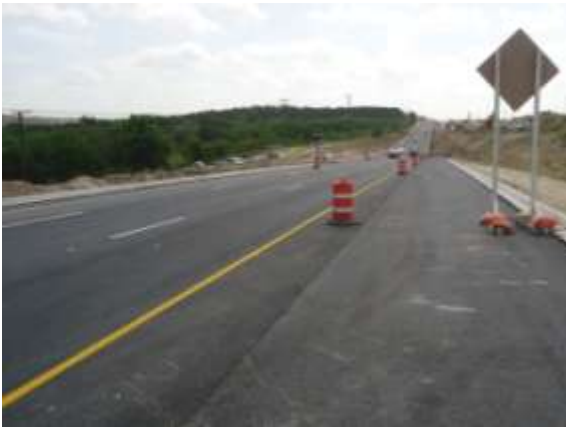
Westbound frontage road construction near the Arterial "A" intersection (Looking East)
