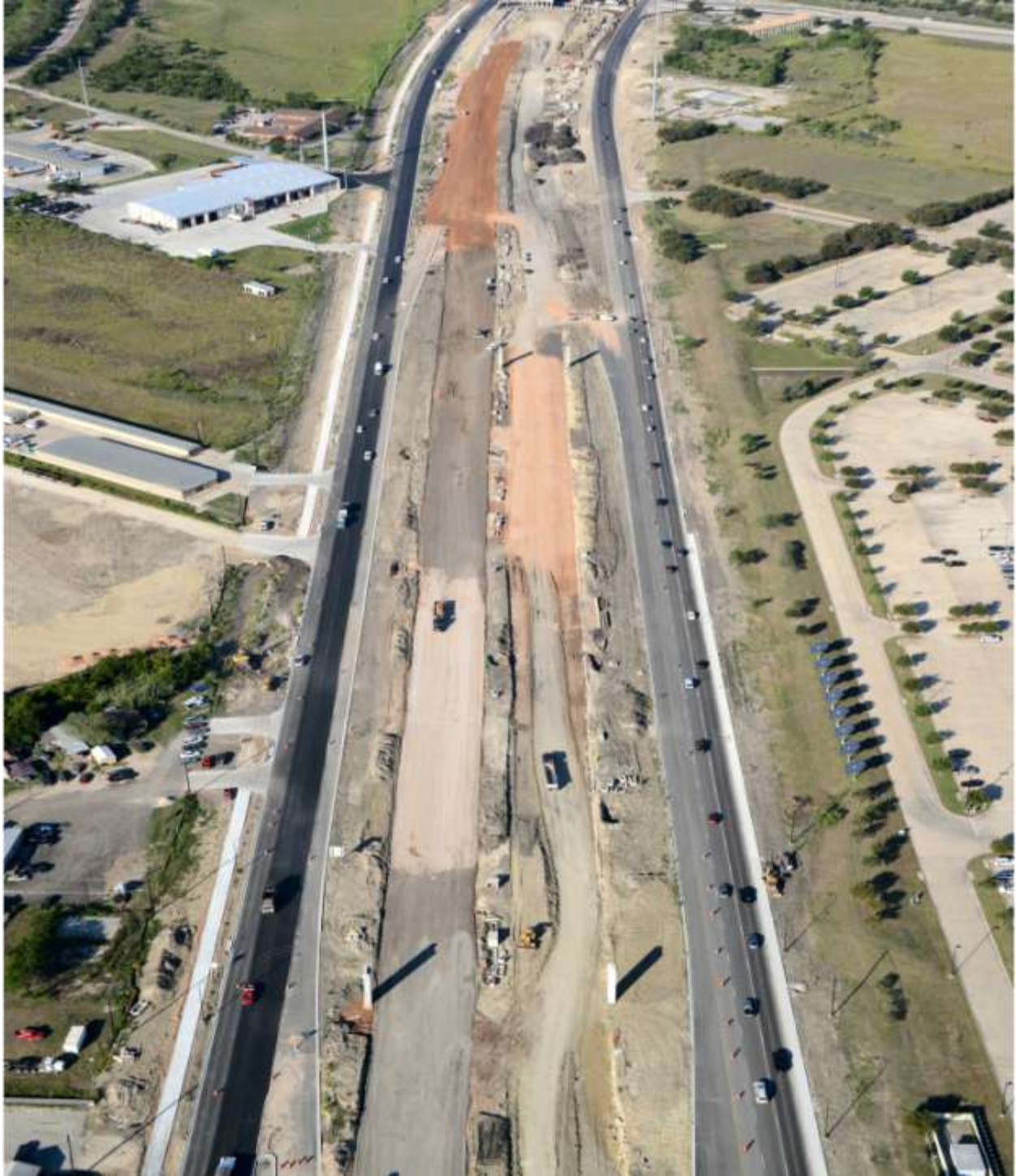
US 290 East at Crofford Lane Intersection looking west (Taken 9/25/2013)
