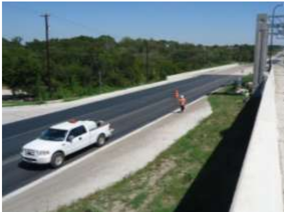
Completed westbound frontage road west of Tributary #5 (Looking Northeast)
