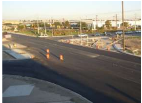
SMA has been placed east of Springdale Road intersection (Looking Northwest)
