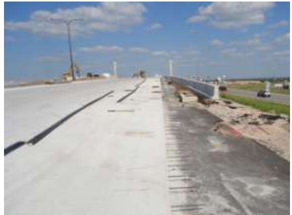
Concrete paving poured on the eastbound mainlanes near SH 130 (Looking East)
