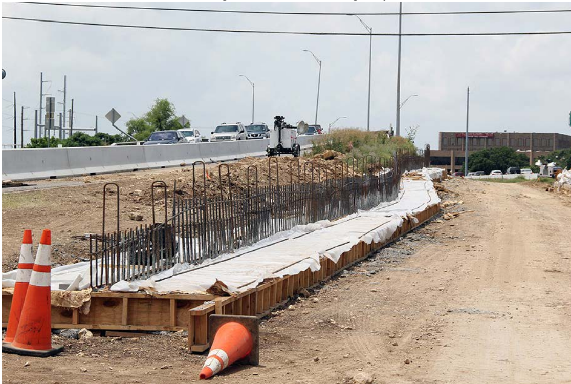
Retaining Wall Construction in Median at RM 2222 – June 2014
