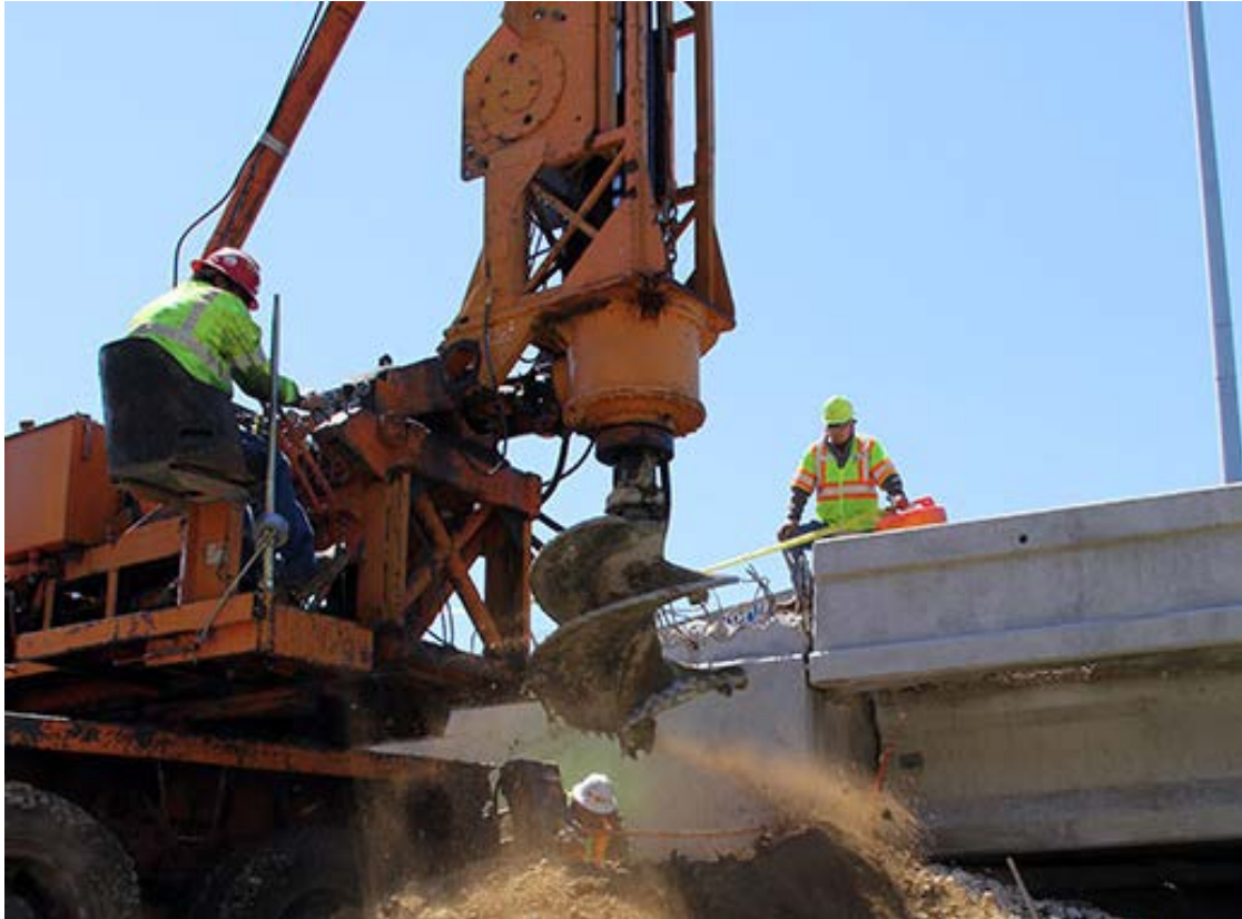
RM 2222 Bridge Foundation Drilling – April 2014
