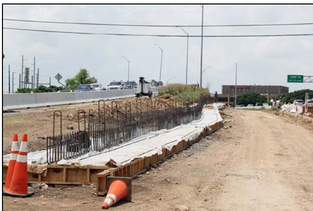
Retaining Wall Construction in Median at RM 2222
