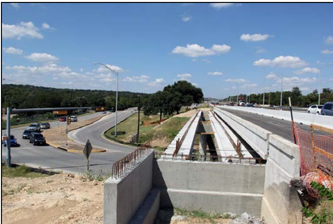
Bridge Beams on Southbound MoPac at 45th Street - September 9, 2014
