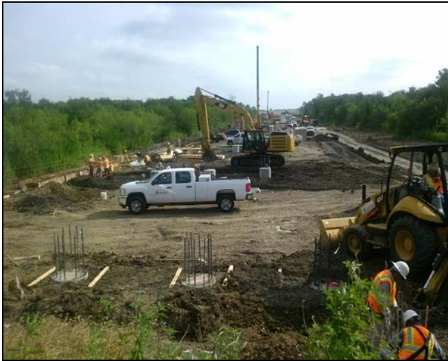
Maha Loop Construction
