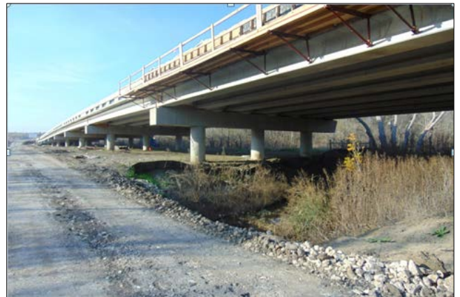
Maha Loop South Bridge Construction
