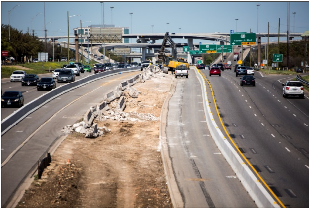
MoPac Improvement Project Construction
