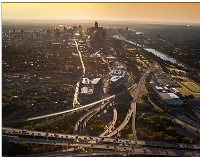
Downtown Austin and the MoPac Blvd Interchange
