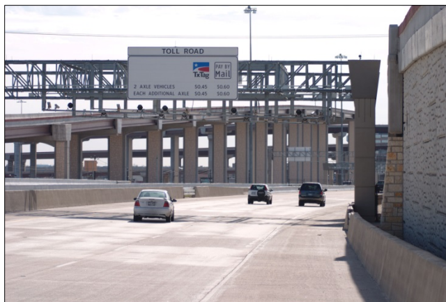
183A Toll Gantry
