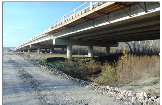
Maha Loop South Bridge Construction
