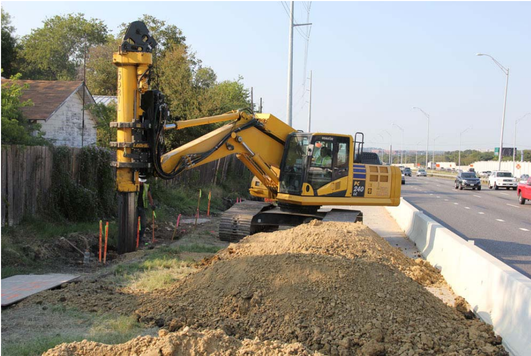
Drilling Foundations for Sound Walls north of Enfield Road
