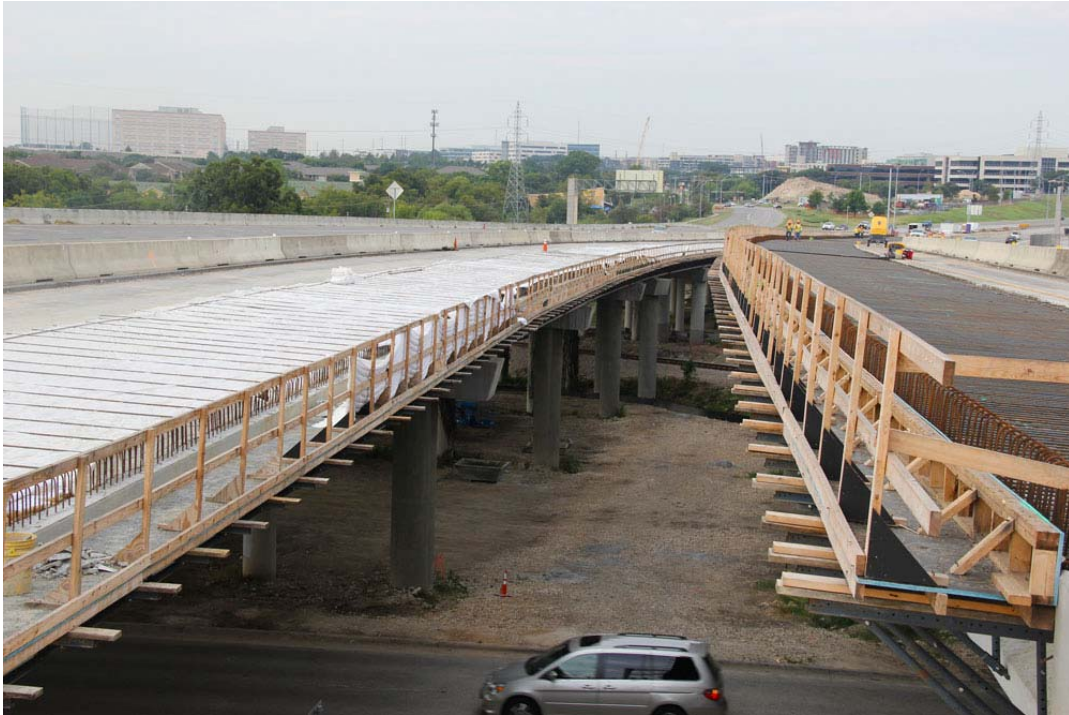
Bridge Widening at Park Bend Drive/Waters Park Drive
