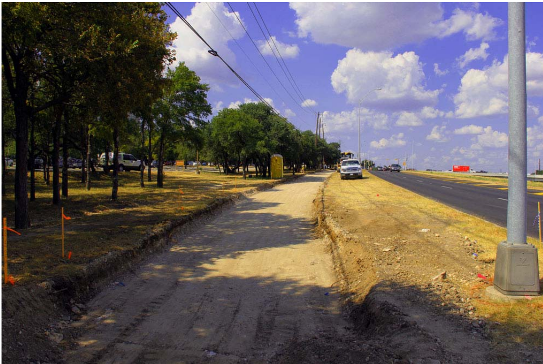
Shared Use Path Construction along southbound MoPac Frontage Road near Loop 360
