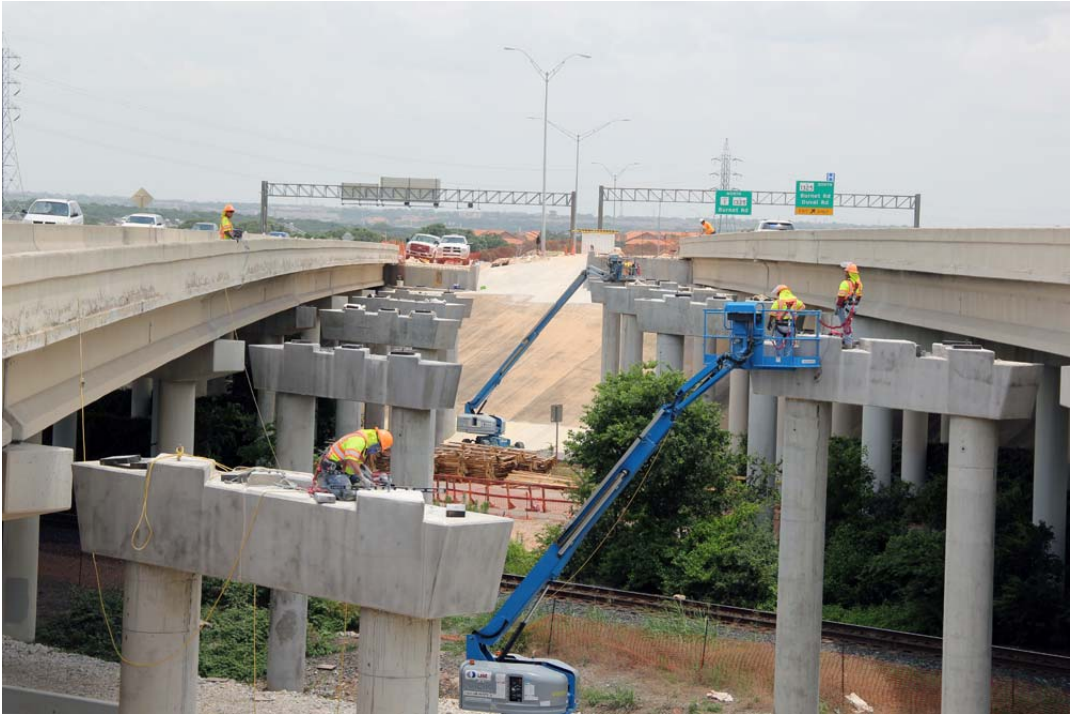
Bridge Bent Construction at Union Pacific Rail Crossing
