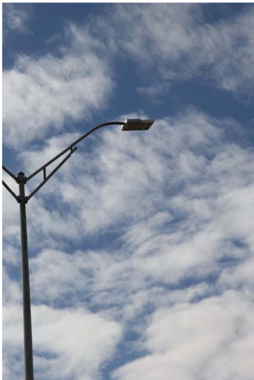
New energy efficient LED highway lights are being installed on MoPac
