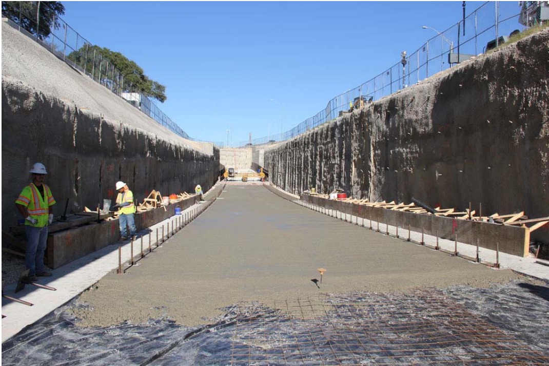
Southbound Undercrossing Construction – December 2015
