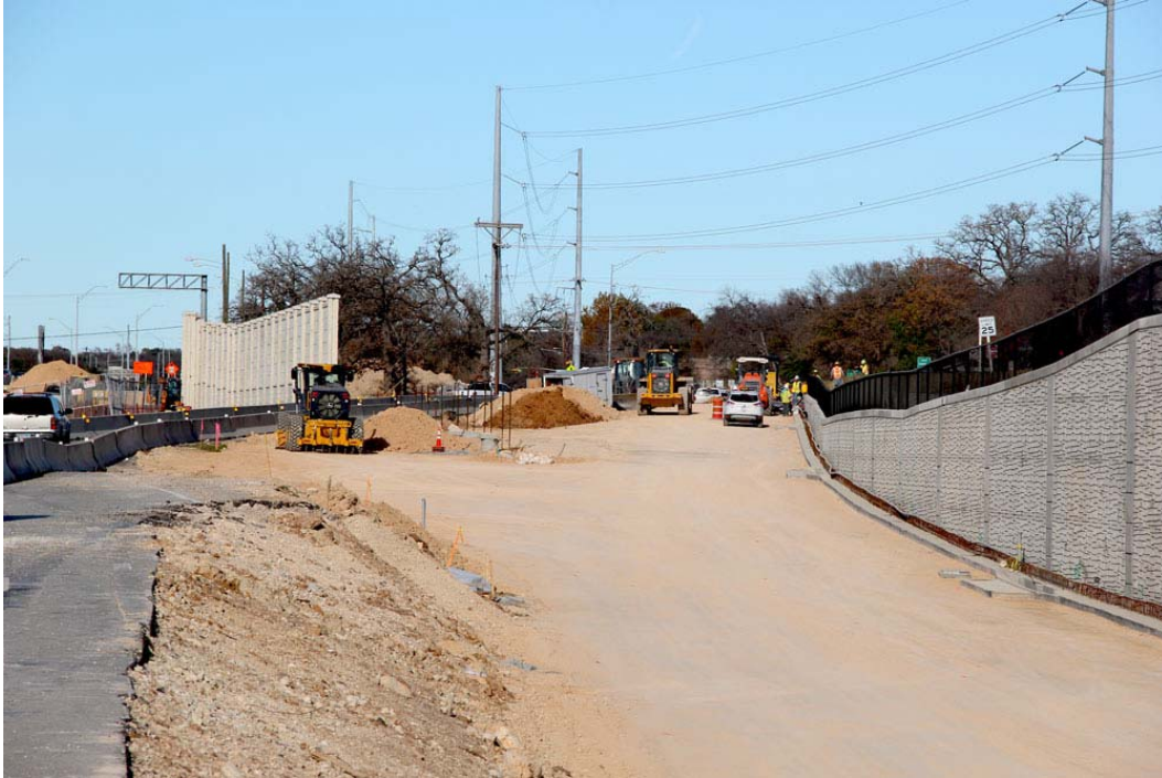
Roadway Construction for Northbound Traffic Shift – December 2015
