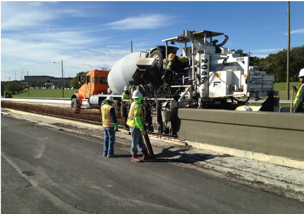
Install of Slip Formed Median Rail – November 2015
