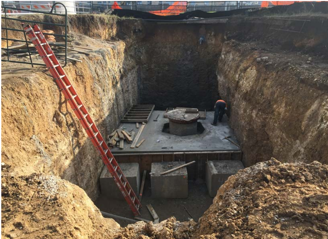
Boring for 42" Waterline at Camp Mabry – December 2015
