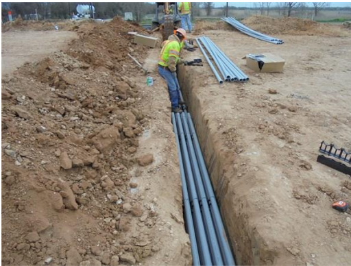
Ductbank being placed
