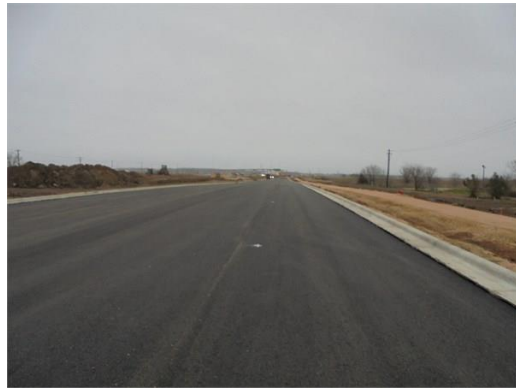
Eastbound general purpose lanes completed
