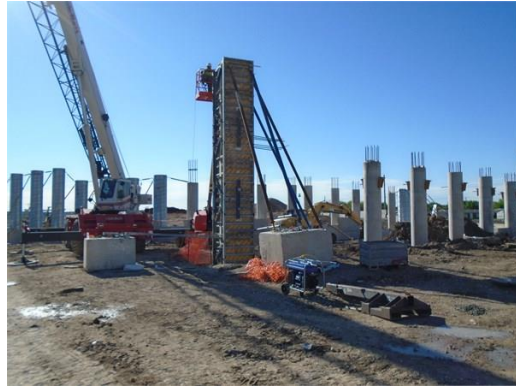
Columns for new FM 973 Overpass
