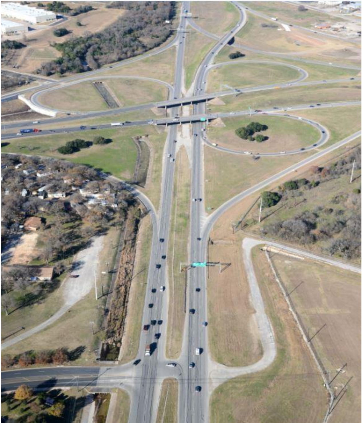
SH 71 at 183 Interchange (Looking North) [December 22, 2016]
