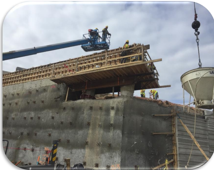
Northbound Main Lane Bridge at Manor/Springdale Road [December 20, 2016]
