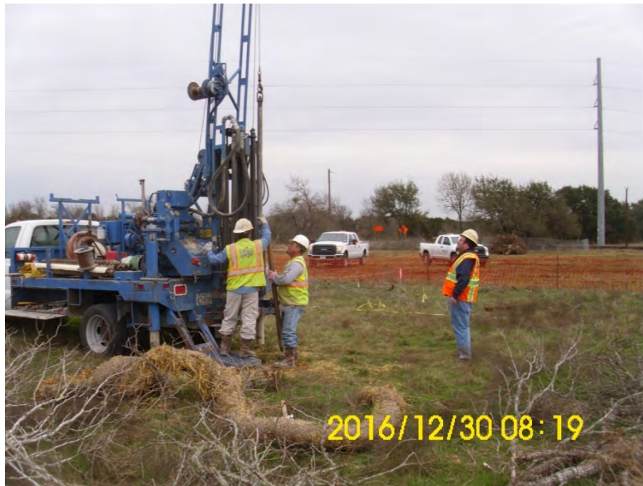
At GS1: Plug & Fill Operation of PF-001 (Borehole B-9) Feature
