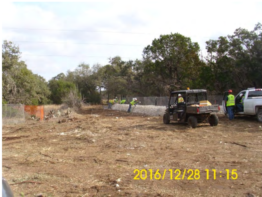
At GS2: Placing Rock Filter Dam at Sensitive Feature F29D
