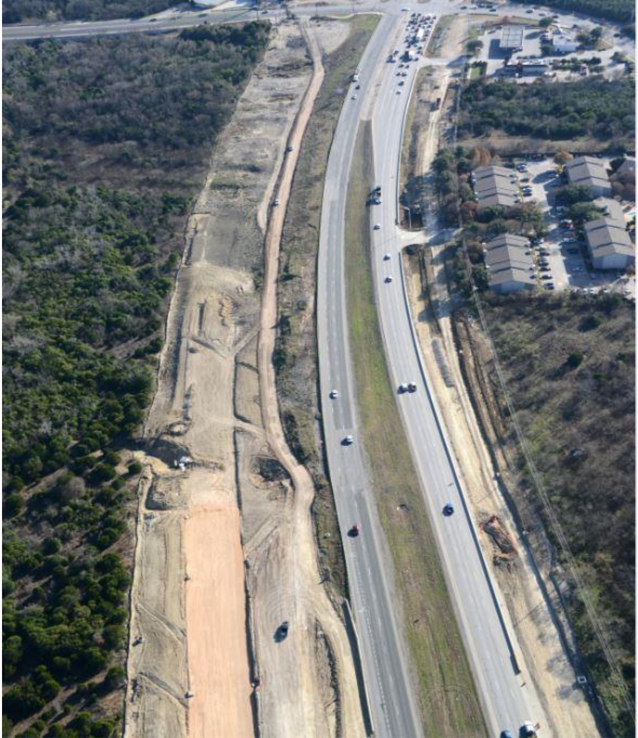
183 North of Loyola Ln (Looking South)
