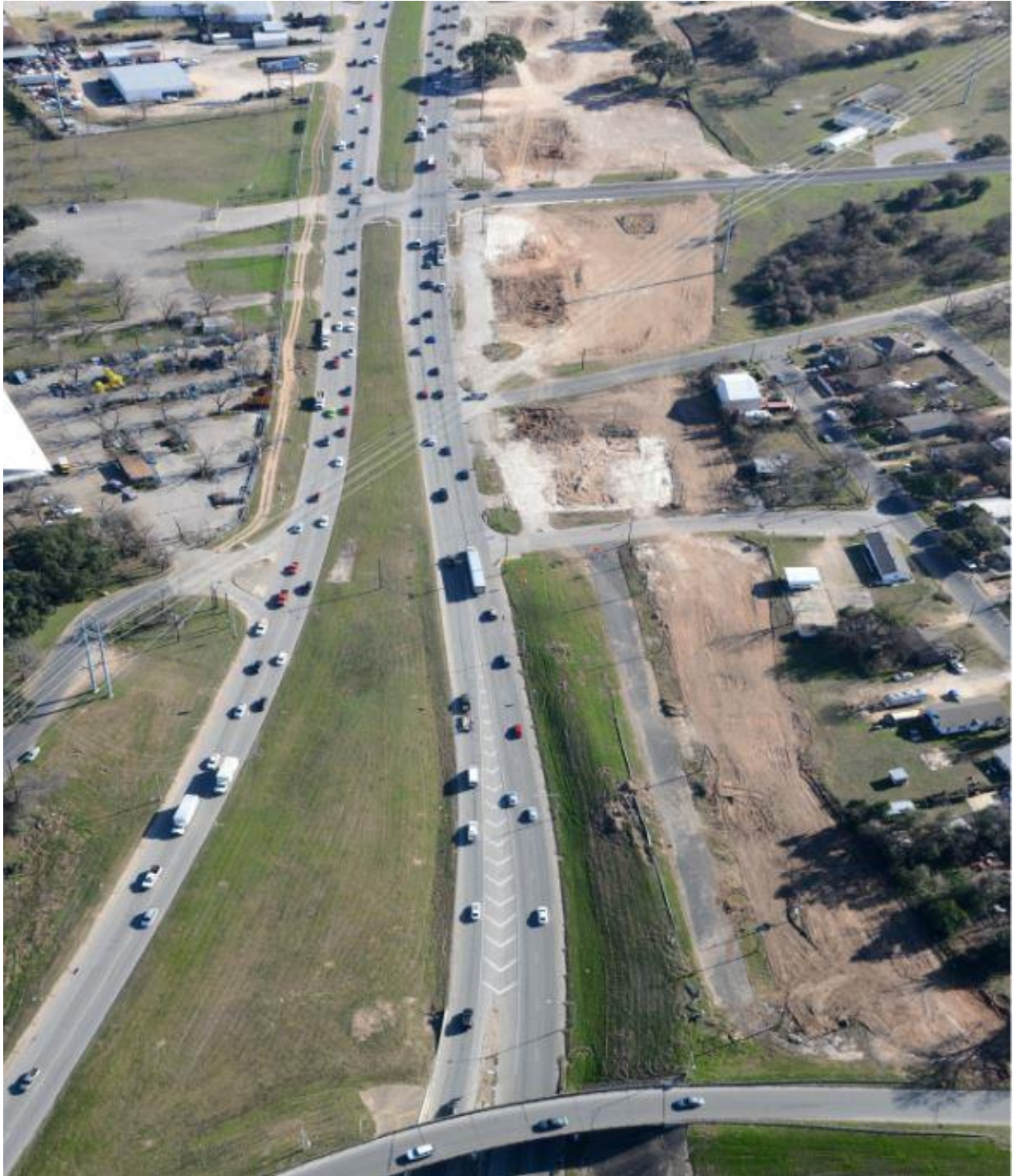
183 Near Vargas Rd (Looking South)
