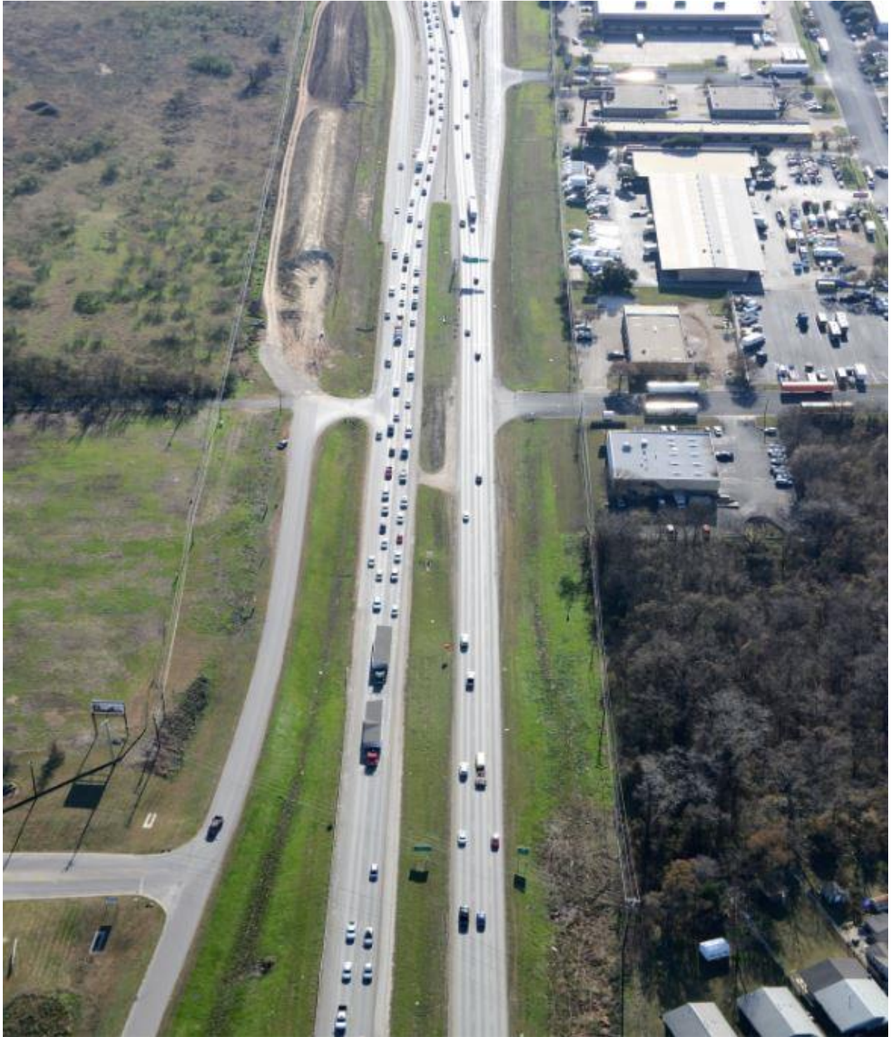
183 Between Boggy Creek and Bolm Rd (Looking South) [December 22, 2016]
