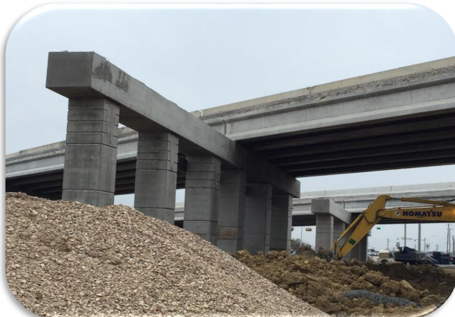
Northbound Mainlane Bridge Construction at Manor/Springdale Road Interchange
