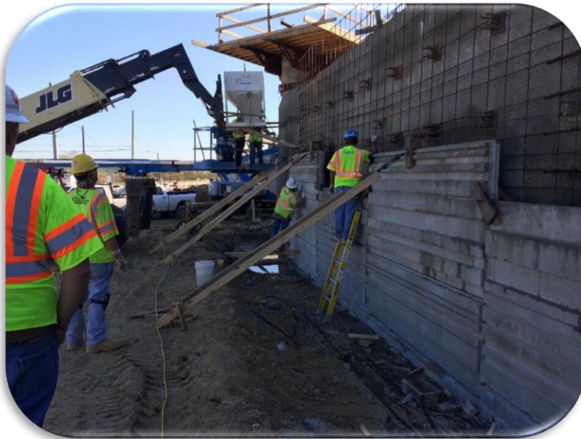
Northbound General Purpose Mainline Wall Construction – Near Manor/ Springdale Road [December 12, 2016]
