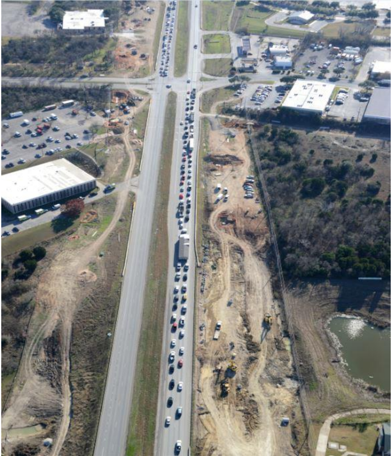
183 at Techni Center Dr (Looking South) [December 22, 2016]
