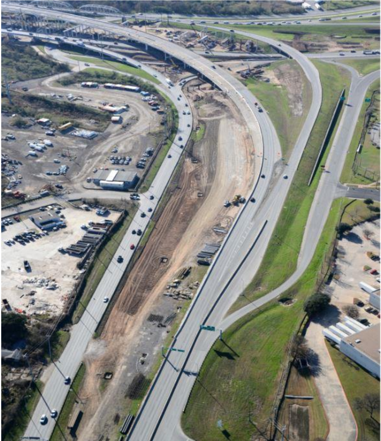
183 at Colorado River Bridge (Looking Southwest) [December 22, 2016]
