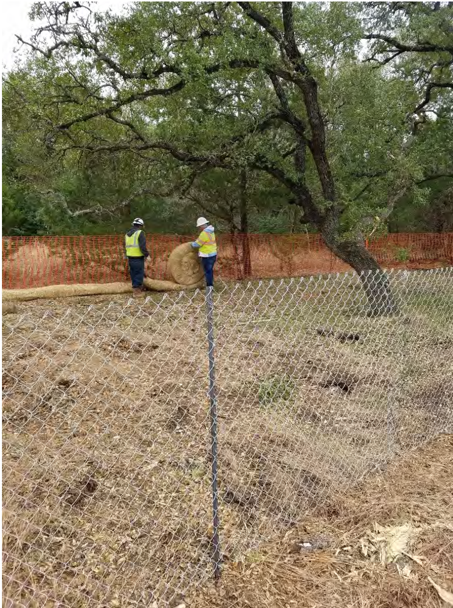
At GS2: Placing Biodegradable Erosion Control Logs
