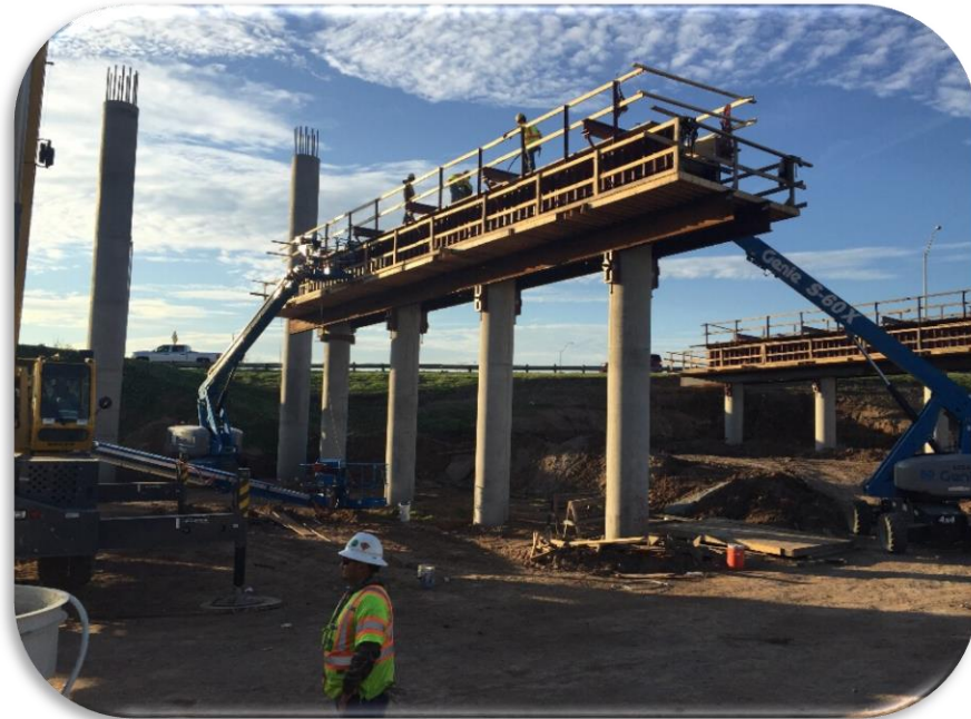
Cesar Chavez Street Bridge Construction at Southbound 183 [December 21, 2016]
