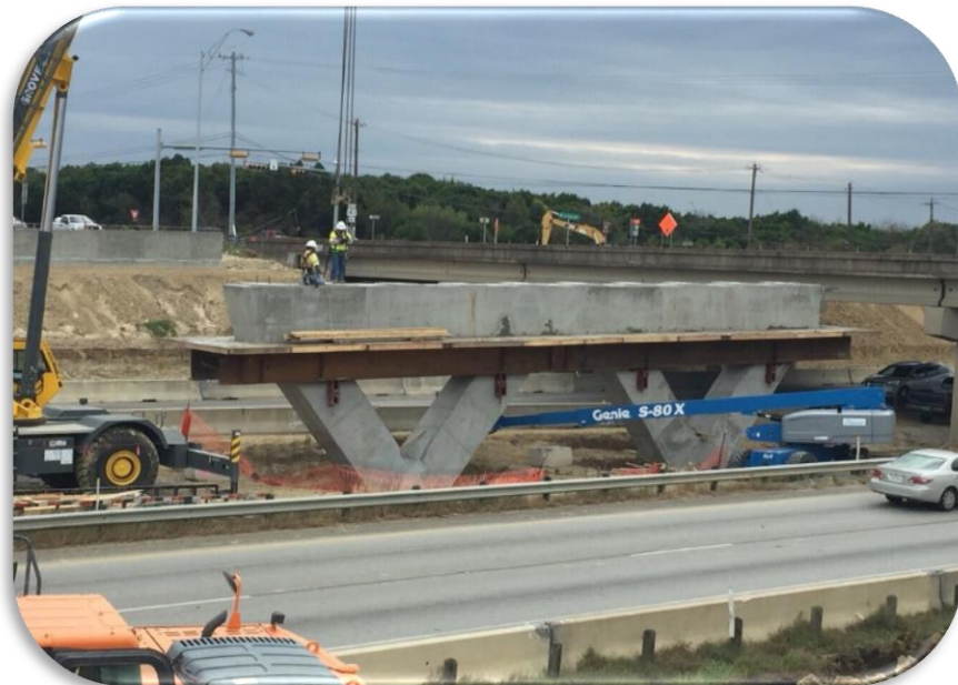
MLK Blvd U-Turn Bridge Construction [December 2, 2016]
