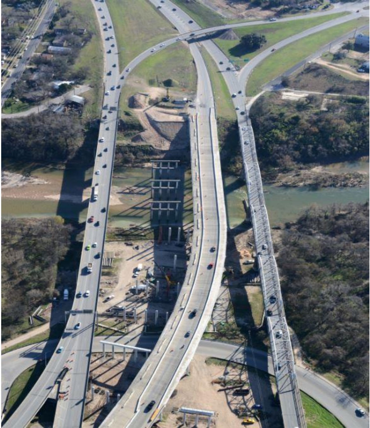
183 near Colorado River Bridge (Looking West)
