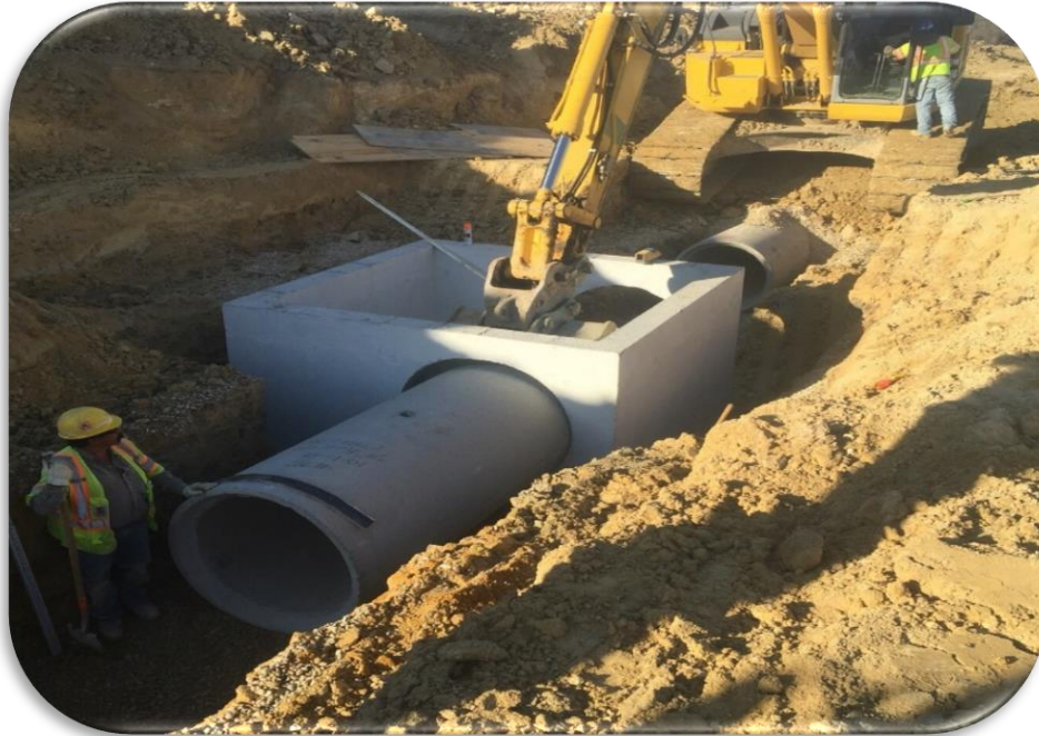
Drainage Construction at Little Walnut Creek
