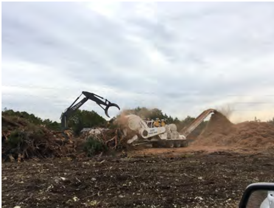
At GS1: Mulching Operation
