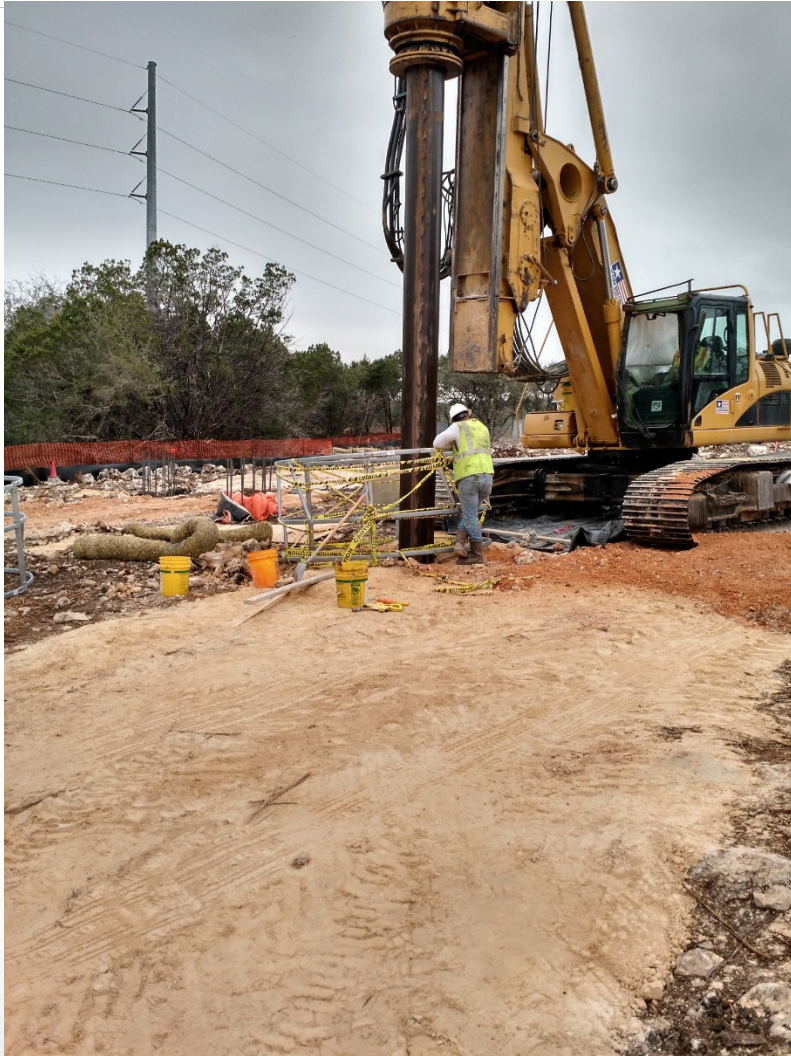
Foundation Drilling and Video Inspection at Bear Creek Bridge
