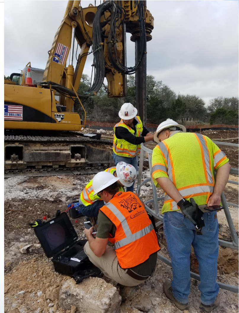
Foundation Drilling and Video Inspection at Bear Creek Bridge
