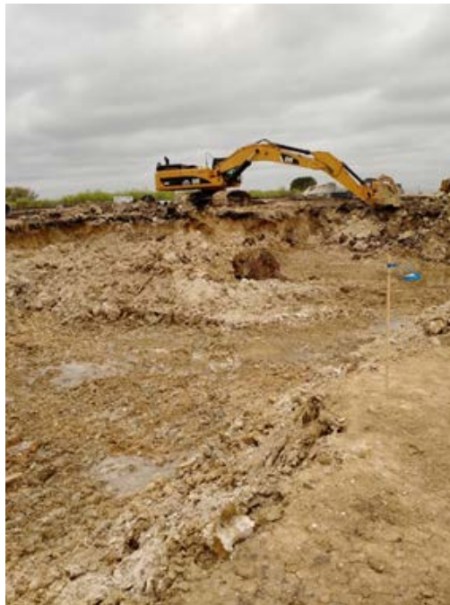
At GS1: Pond A Excavation
