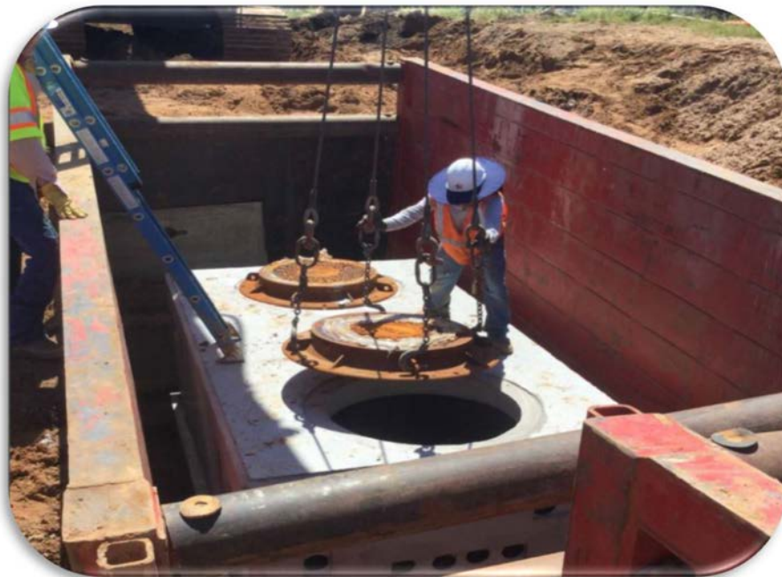
Joint Trench Utilities
