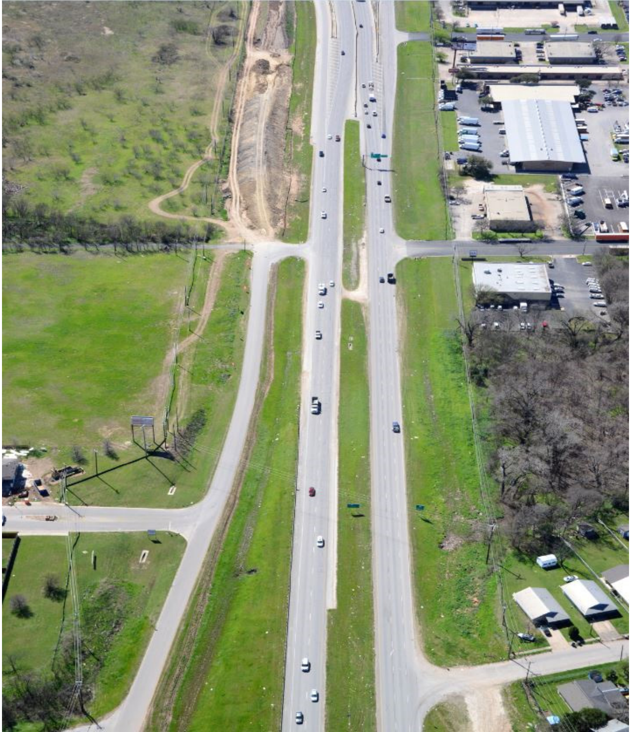
183 Between Boggy Creek and Bolm Rd (Looking South) [February 24, 2017]
