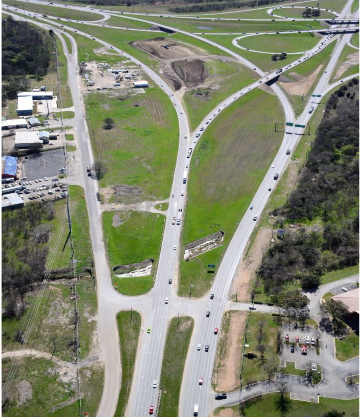
Old Bastrop Rd – SH 71 – 183 N Ramp (Looking Southeast)
