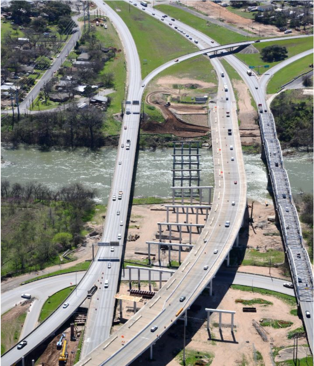
183 near Colorado River Bridge (Looking West)
