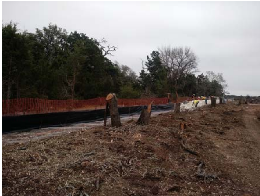
At GS2: Installing Rock Filter Dam
