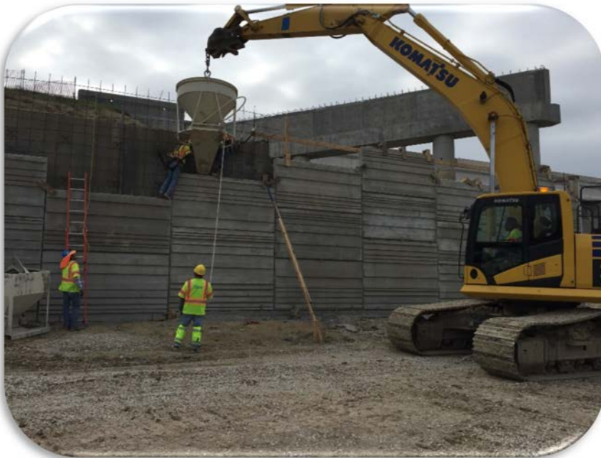
Tie Additional Steel on Soil Nail Wall (Northbound) [March 7, 2017]
