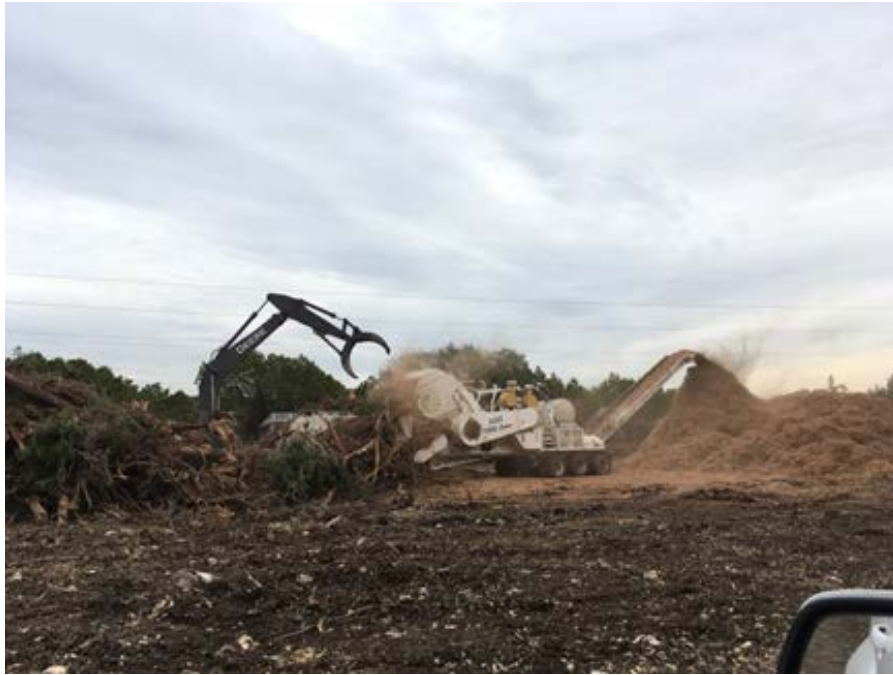
At GS1: Mulching Operation
