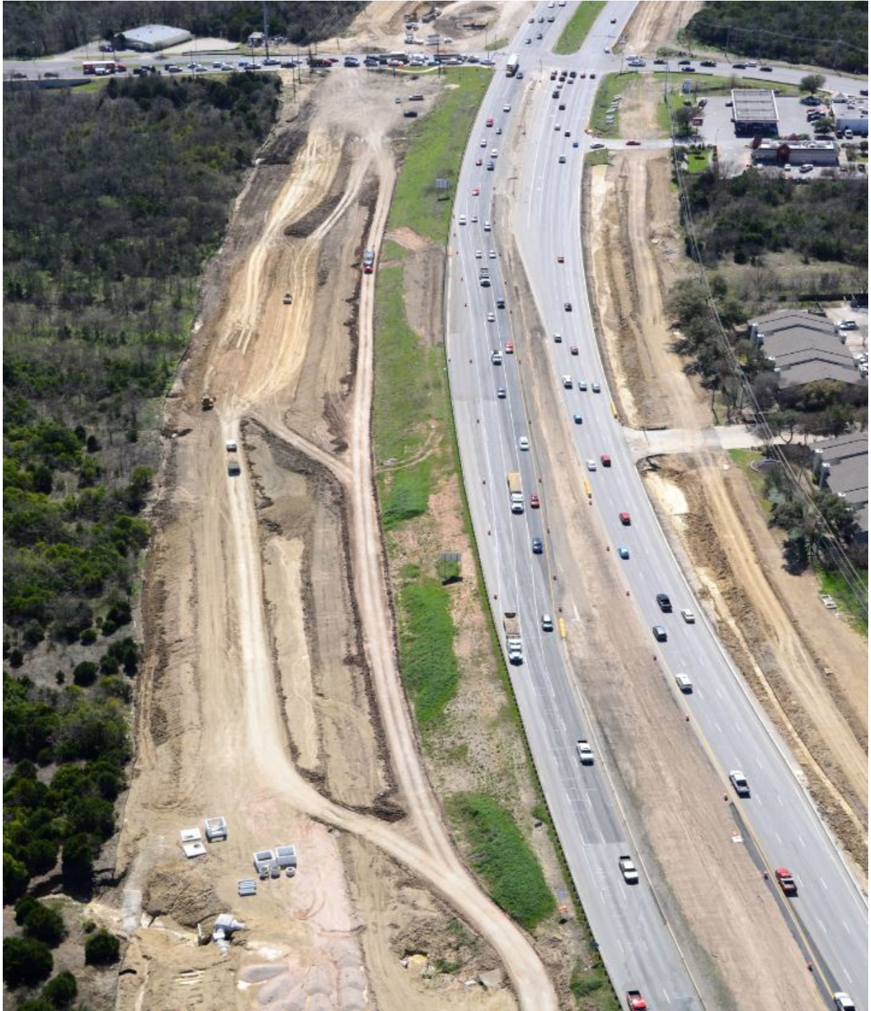
183 North of Loyola Ln (Looking South)
