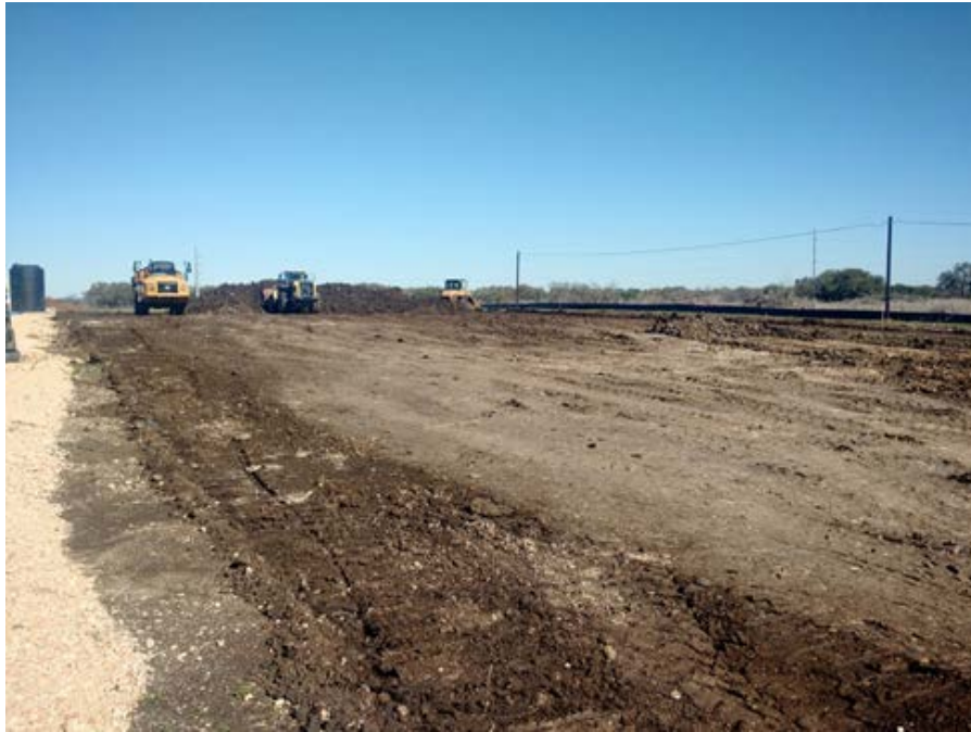
At GS1: Stripping Topsoil
