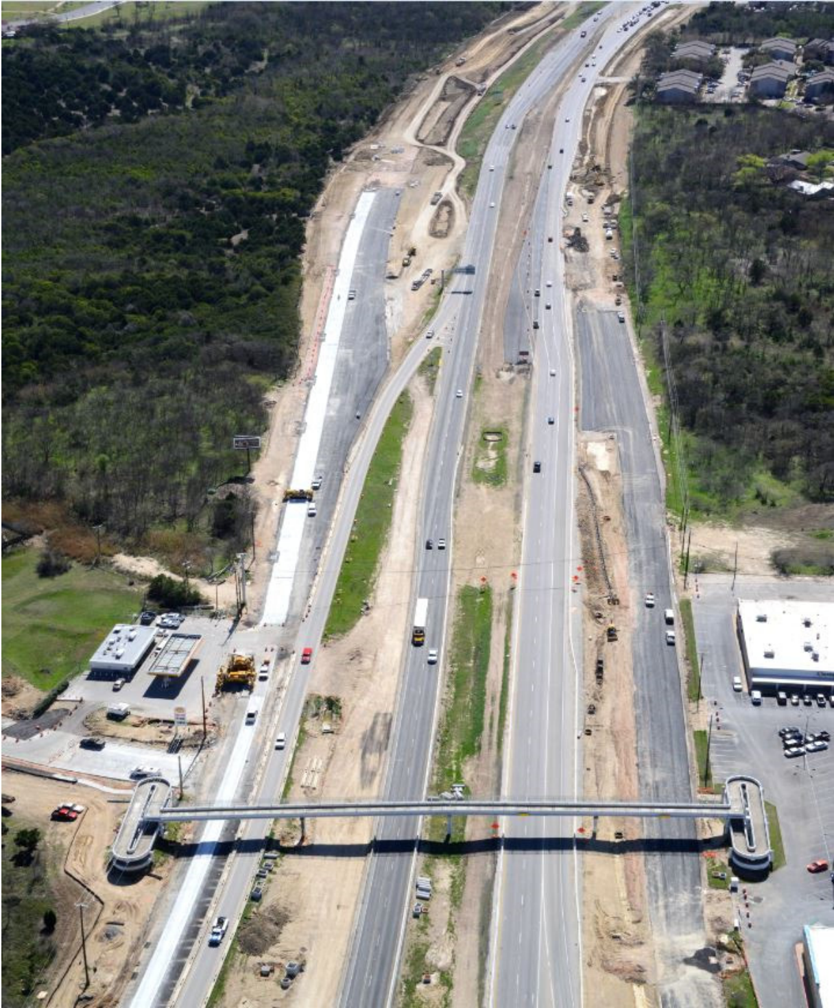
183 at Purple Sage Pedestrian Bridge (Looking South)
