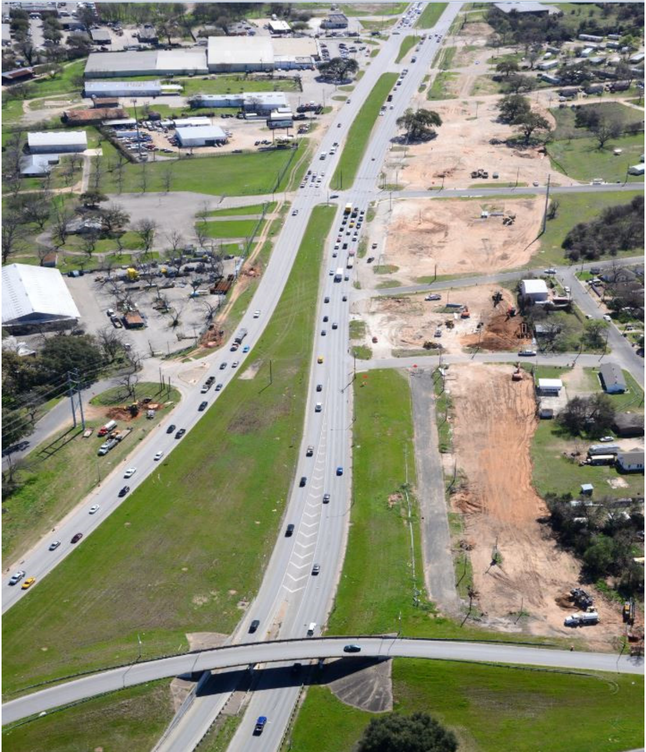
183 Near Vargas Rd (Looking South)
