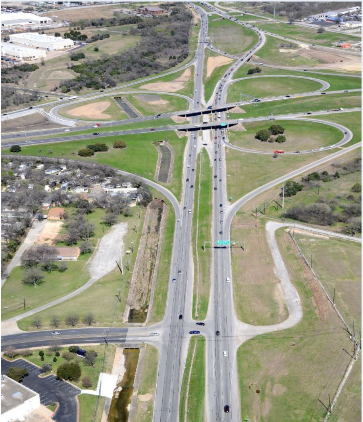
SH 71 at 183 Interchange (Looking North)
