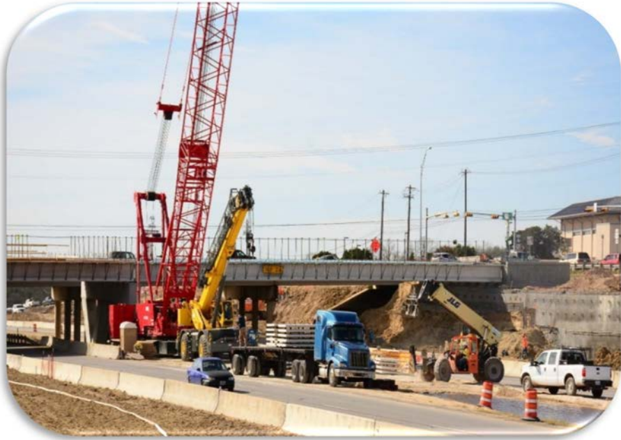
Bridge Construction near MLK Boulevard [January 25, 2017]
