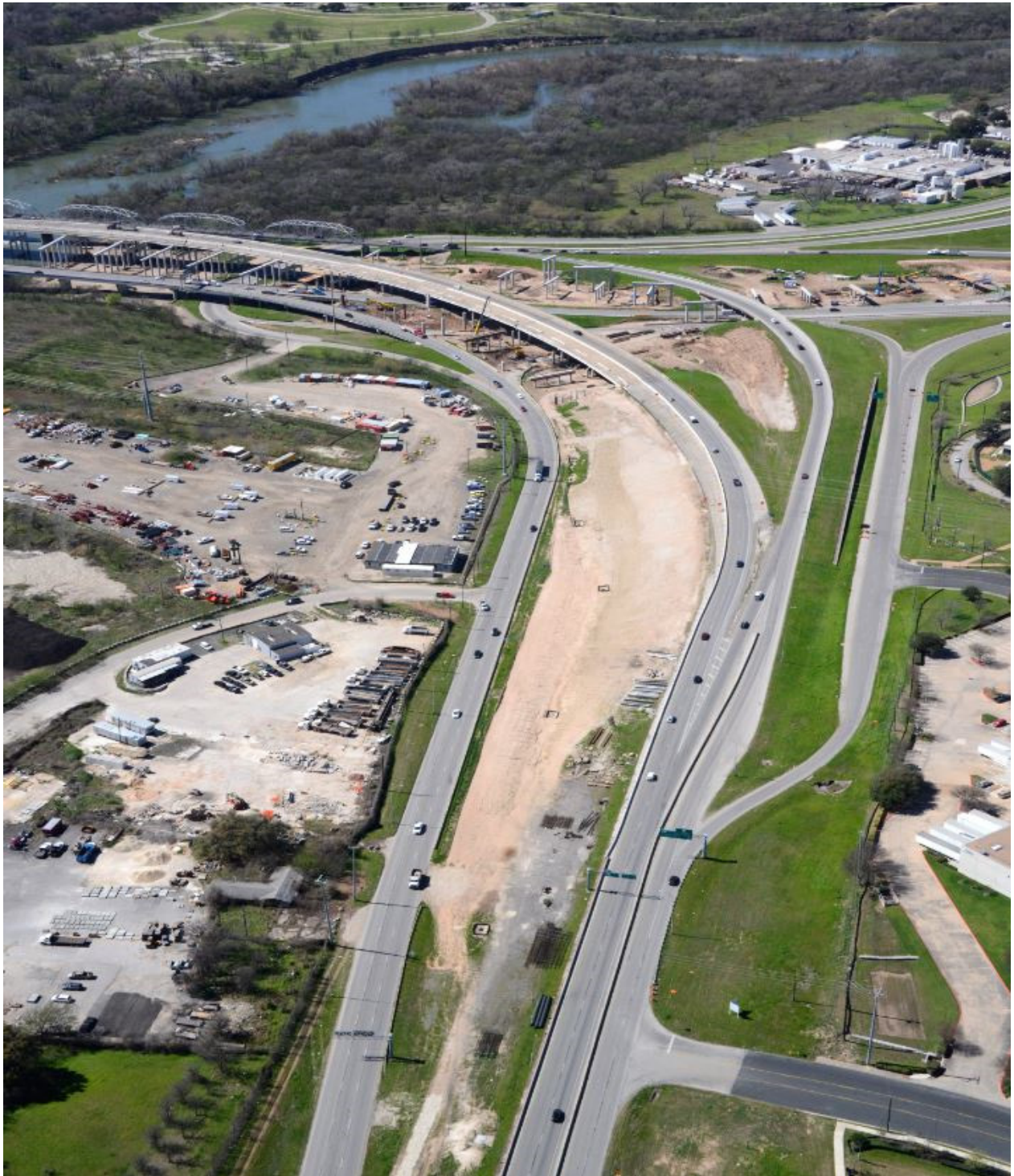
183 at Colorado River Bridge (Looking Southwest)
