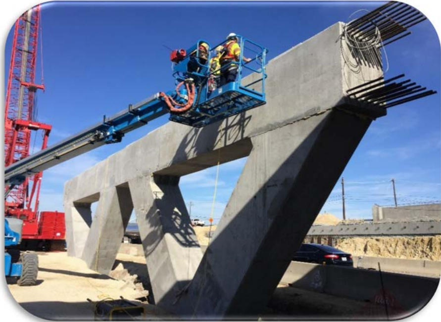
Bridge Cap Construction near MLK Boulevard [January 10, 2017]
