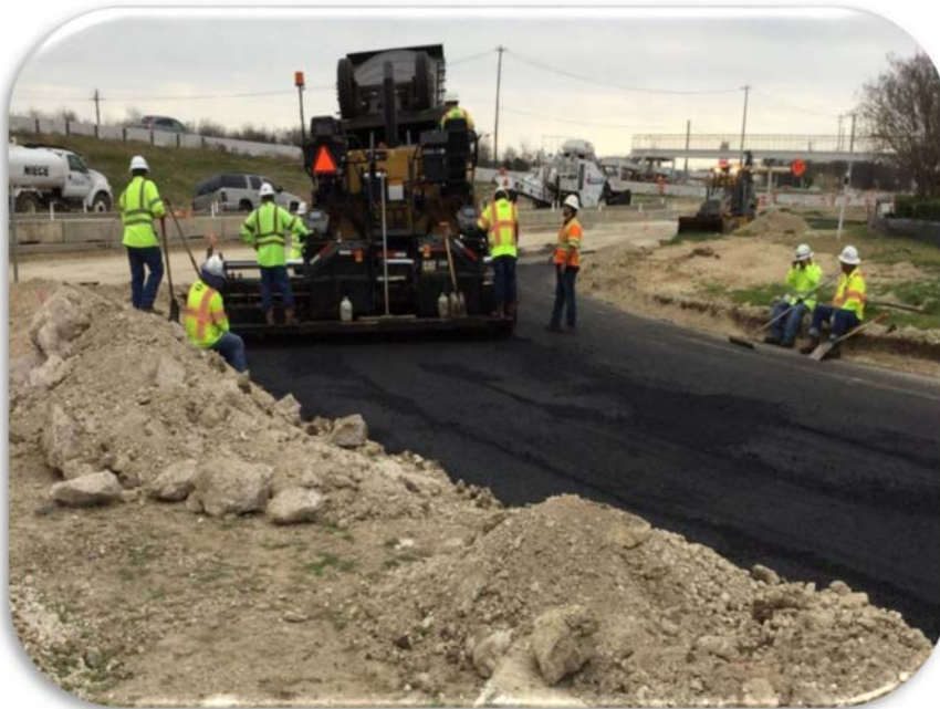
Hot Mix Asphalt near Manor/Springdale Road
