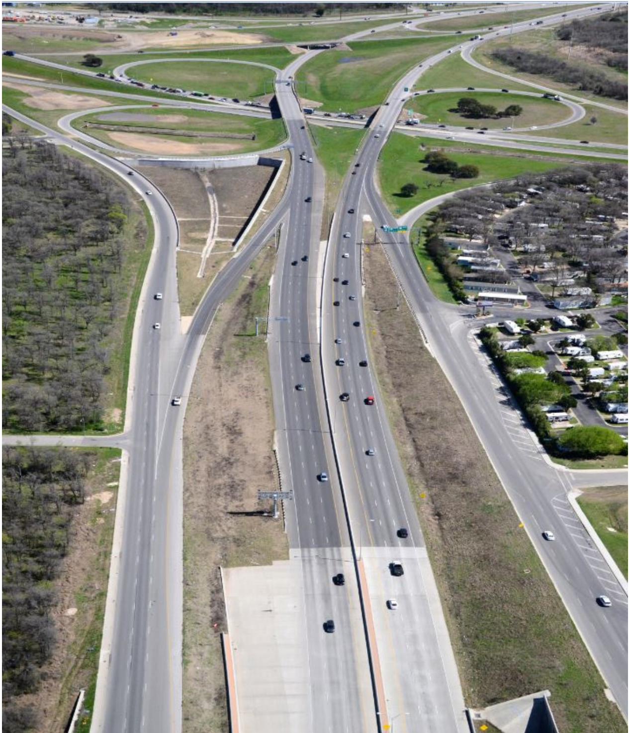
WB/EB SH 71 at 183 Interchange (Looking East)
