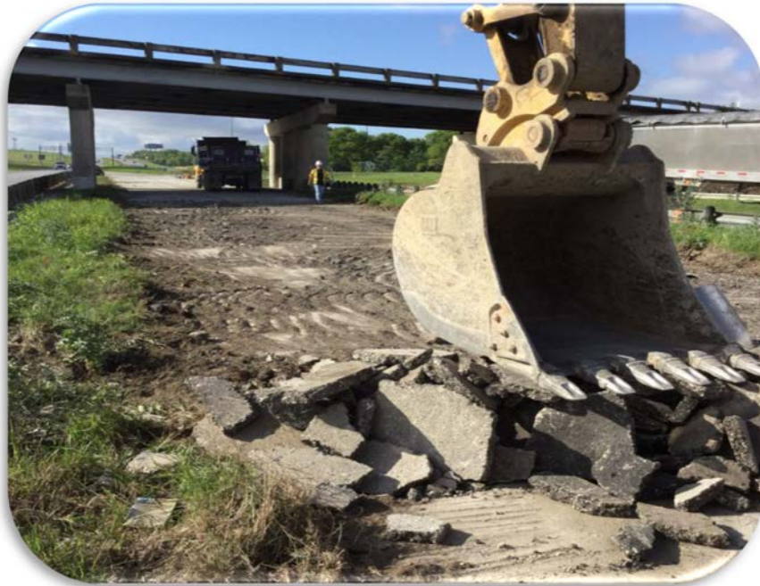
Excavating & Demo for Drill Shaft Rig
