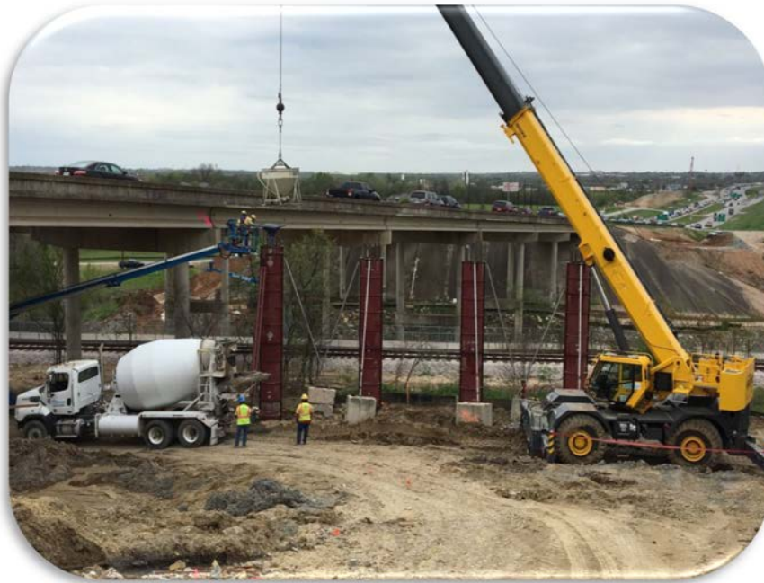
Southbound Bridge Columns at Boggy Creek
