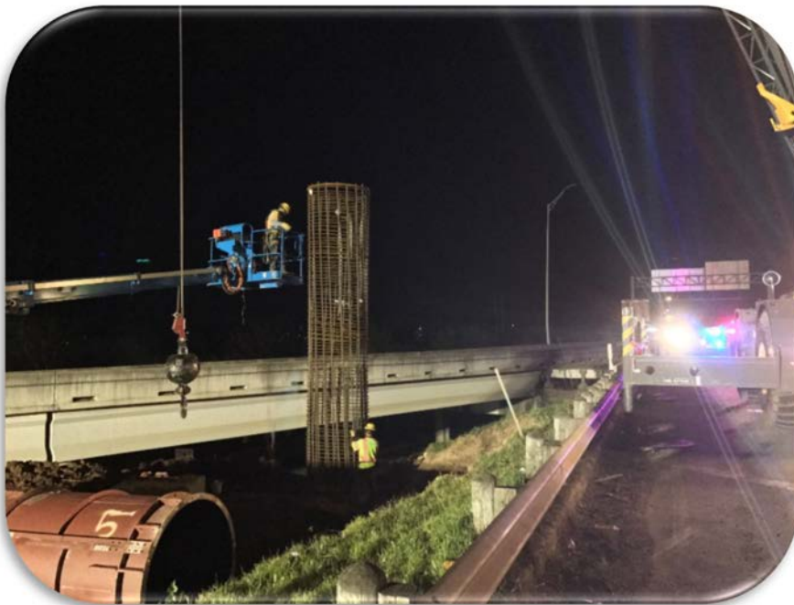
Bridge Columns at Colorado Bridge
