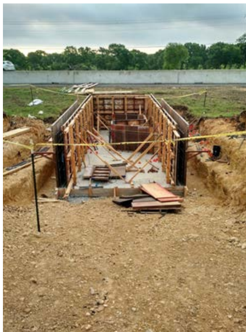
At GS1: Splitter Structure at Pond A
