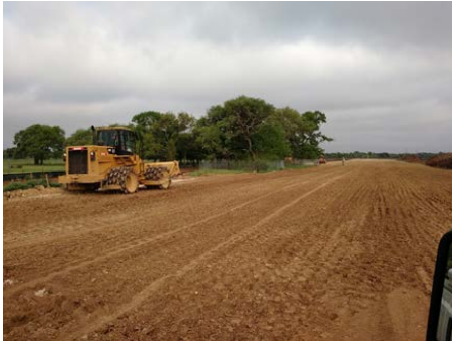
At GS1: Compacting Embankment along the Eastbound Mainlane
