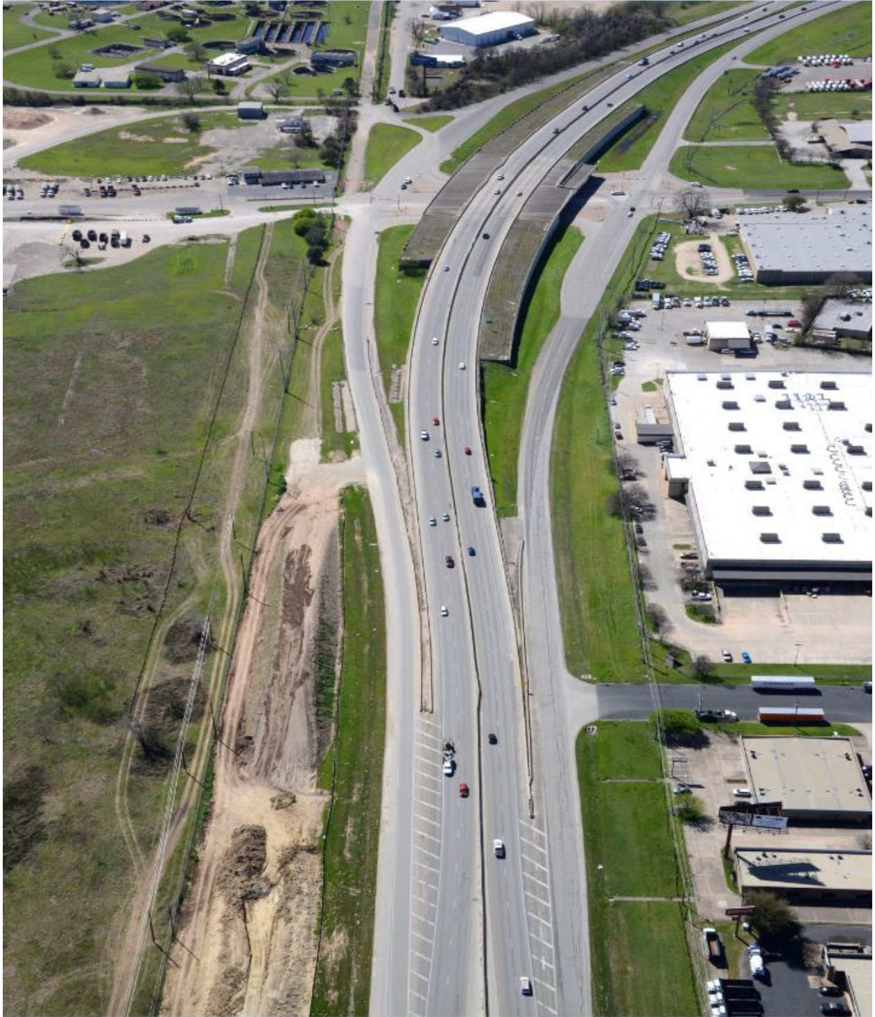
183 at Bolm Rd (Looking South) [February 24, 2017]
