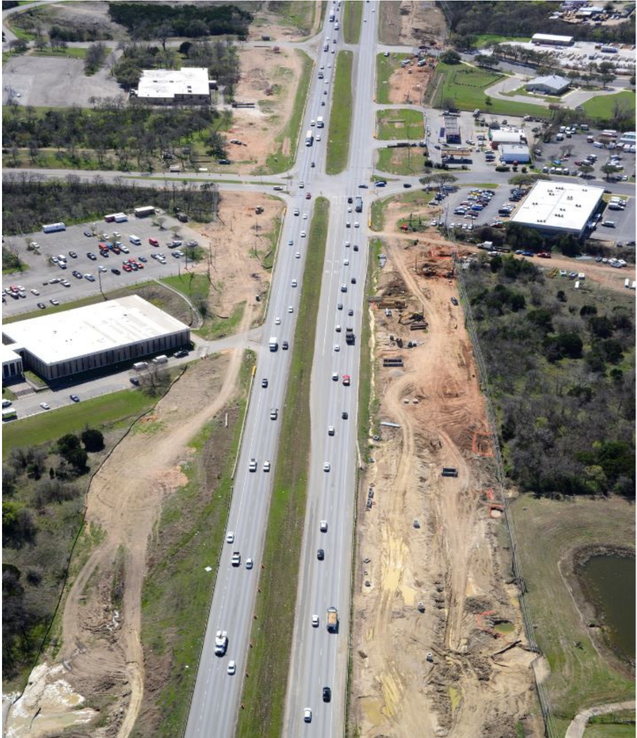
183 at Techni Center Dr (Looking South) [February 24, 2017]
