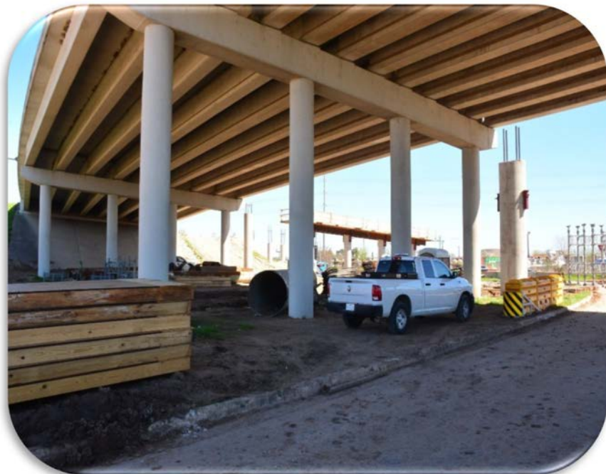
Bridge Cladding near Airport Boulevard & Leander Loop
