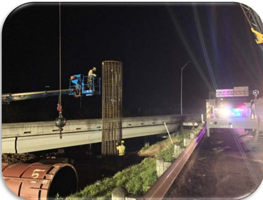
Bridge Columns at Colorado Bridge
