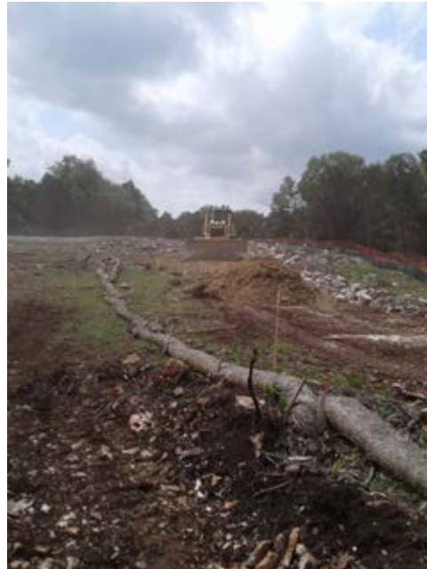
At GS1: Embankment Placement of Haul Road South of Bear Creek
