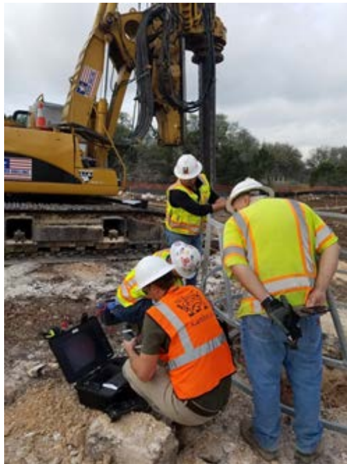
At GS1: Video Monitoring of Bear Creek Bridge Bent 3 Shaft C
