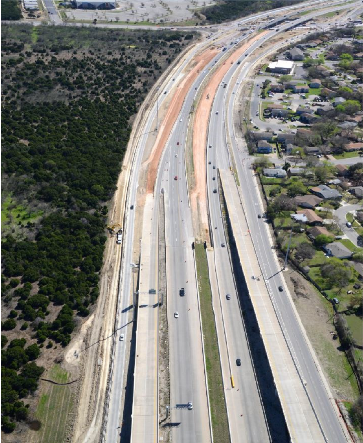
183 south of US 290 (Looking South)
