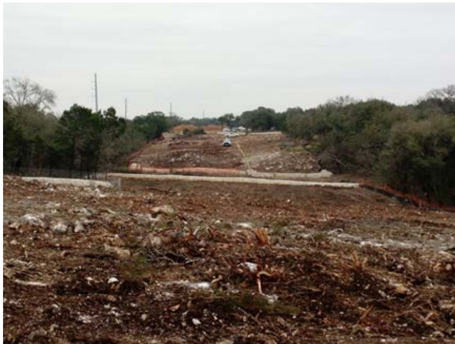
At GS1: Bear Creek Looking North
