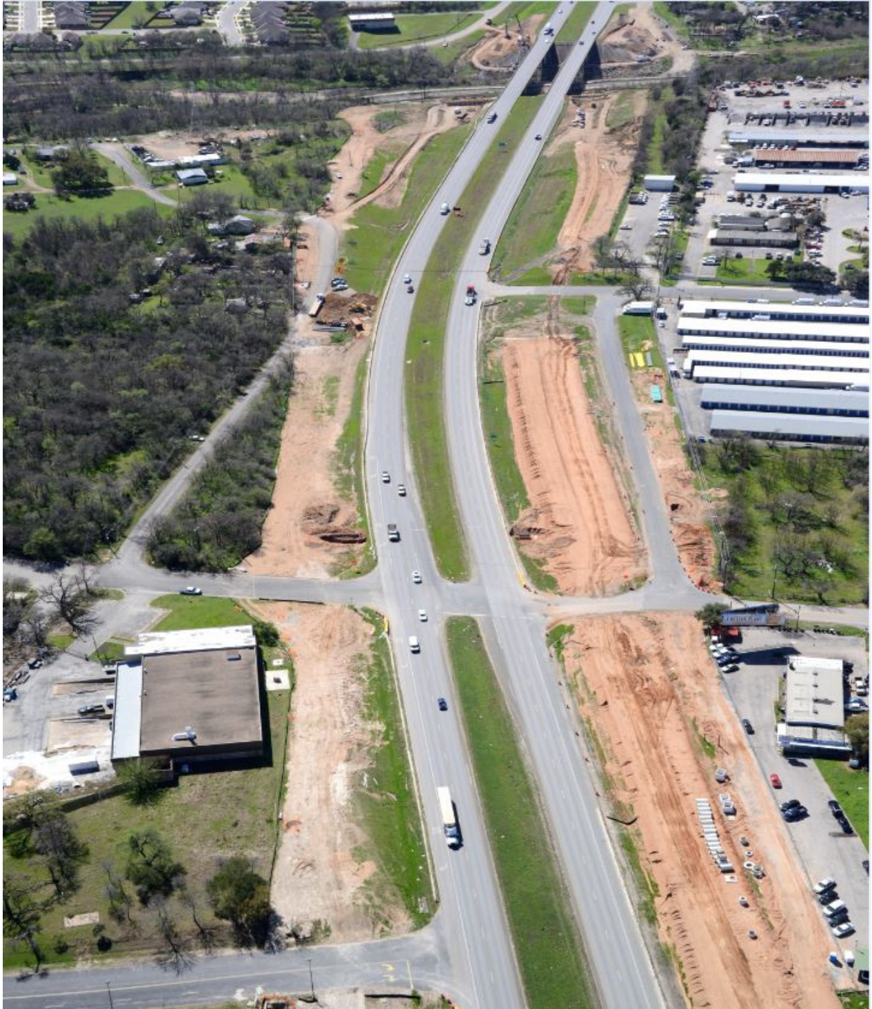
183 at Hudson St and Harold Ct (Looking South) [February 24, 2017]
