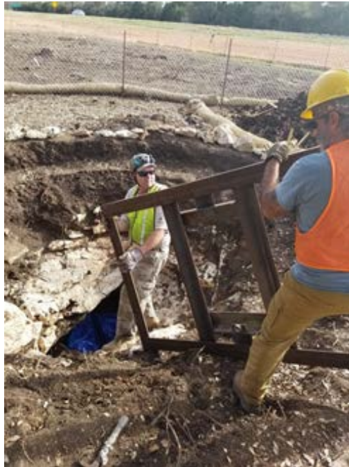
At Interchange: Installing Grate on Sensitive Feature PF04
