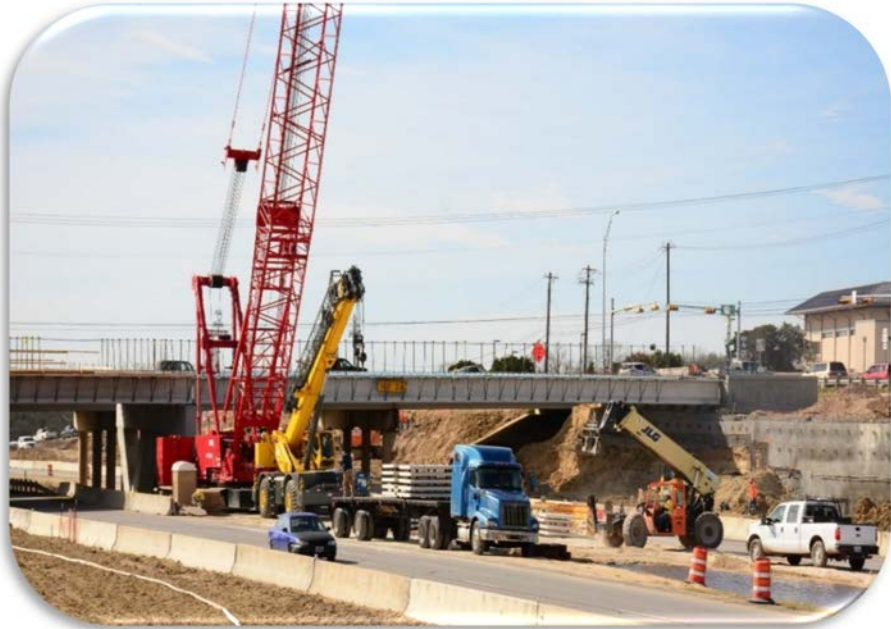
Bridge Construction near MLK Boulevard [January 25, 2017]
