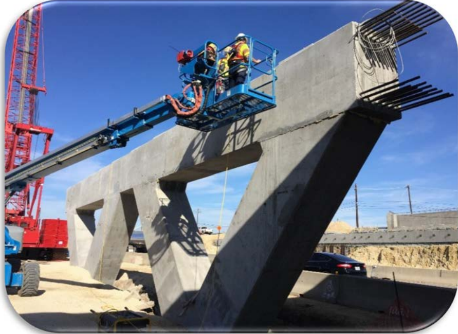
Bridge Cap Construction near MLK Boulevard [January 10, 2017]
