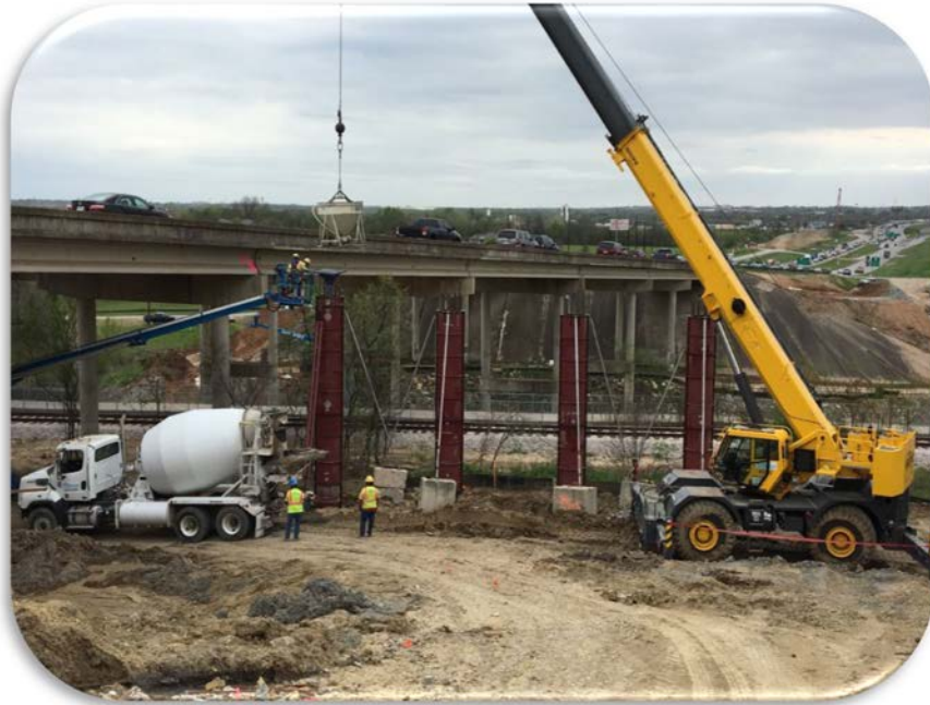
Southbound Bridge Columns at Boggy Creek
