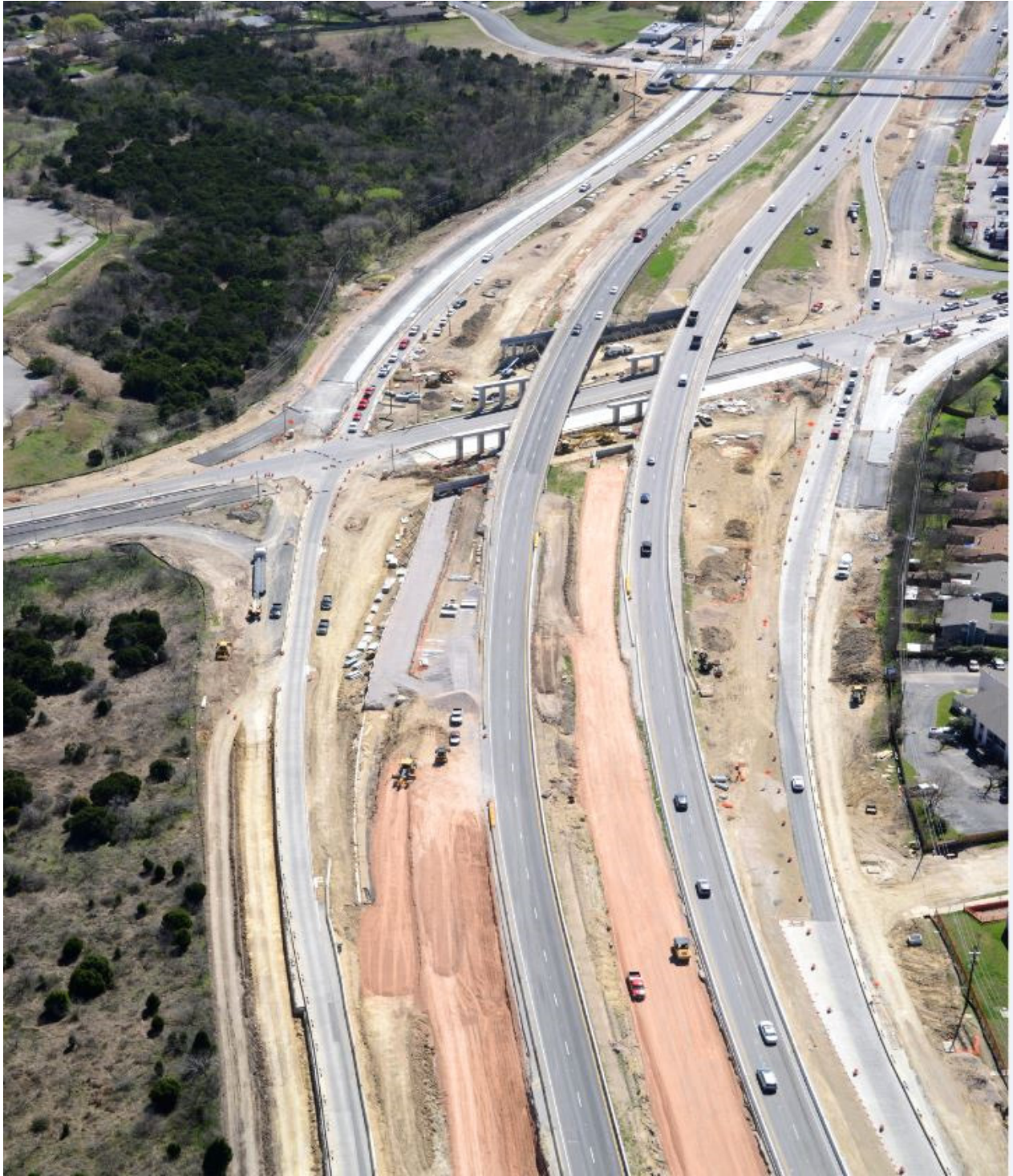
183 at Springdale/Manor Rd Interchange (Looking South) [February 24, 2017]
