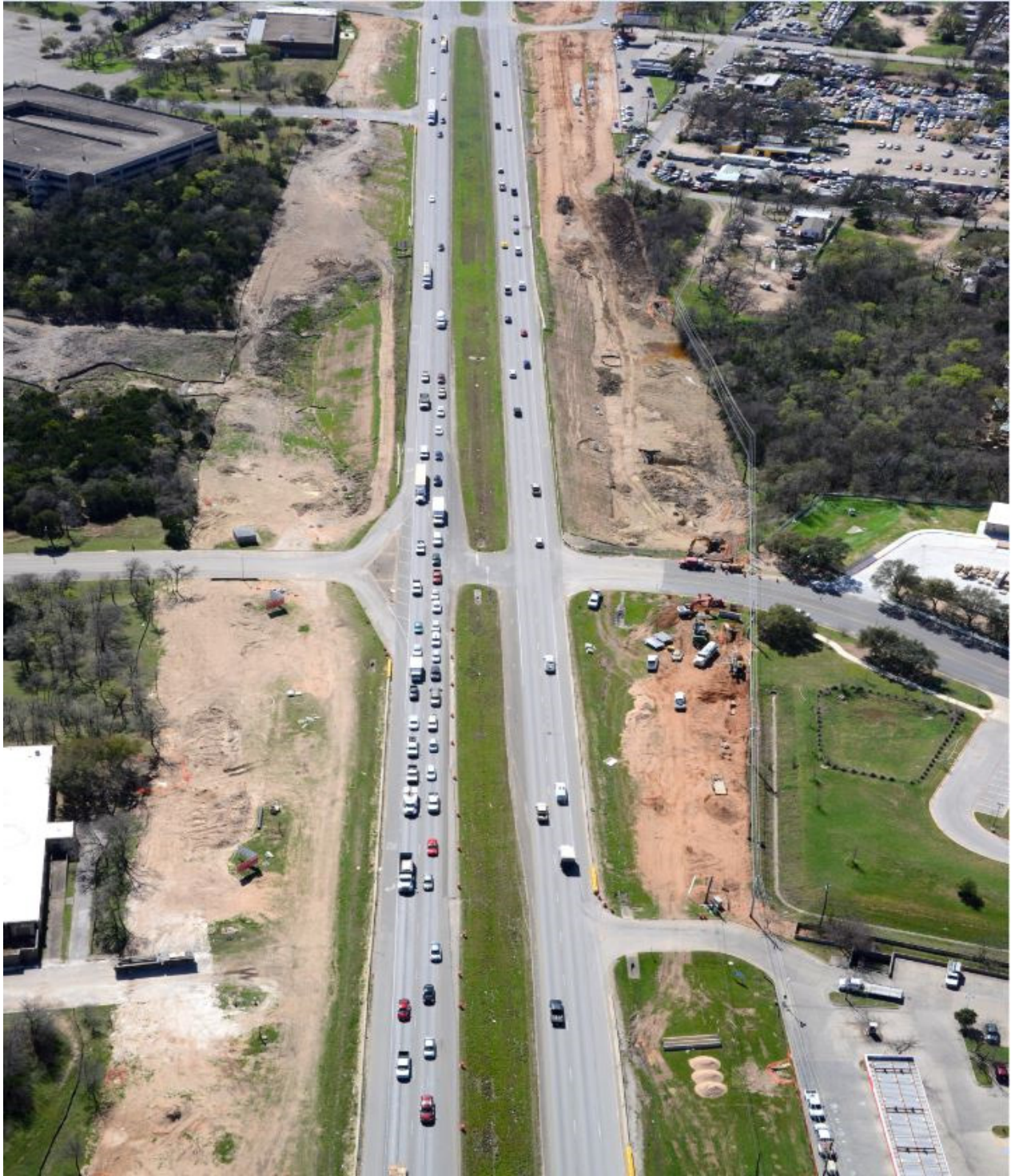
183 at Central Ave (Looking South) [February 24, 2017]
