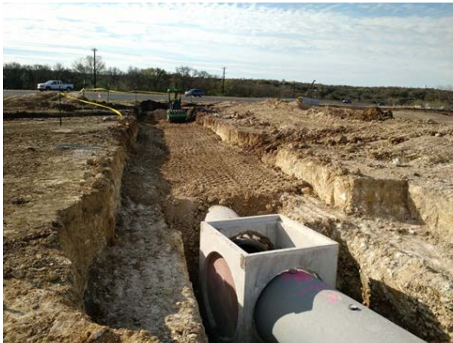
At GS1: Backfilling Operation of a Drainage Line
