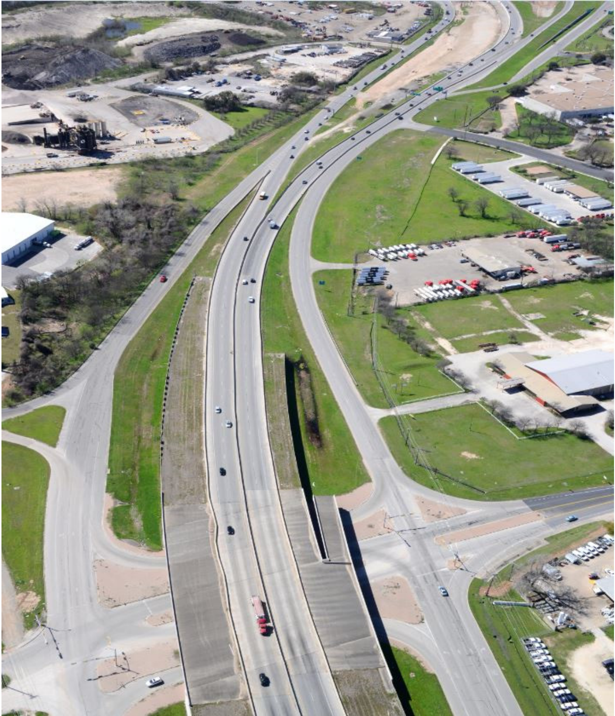
183 near Bolm Rd (Looking South)
