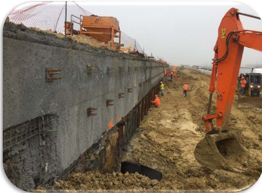
Soil Nail Wall Construction [January 23, 2017]
