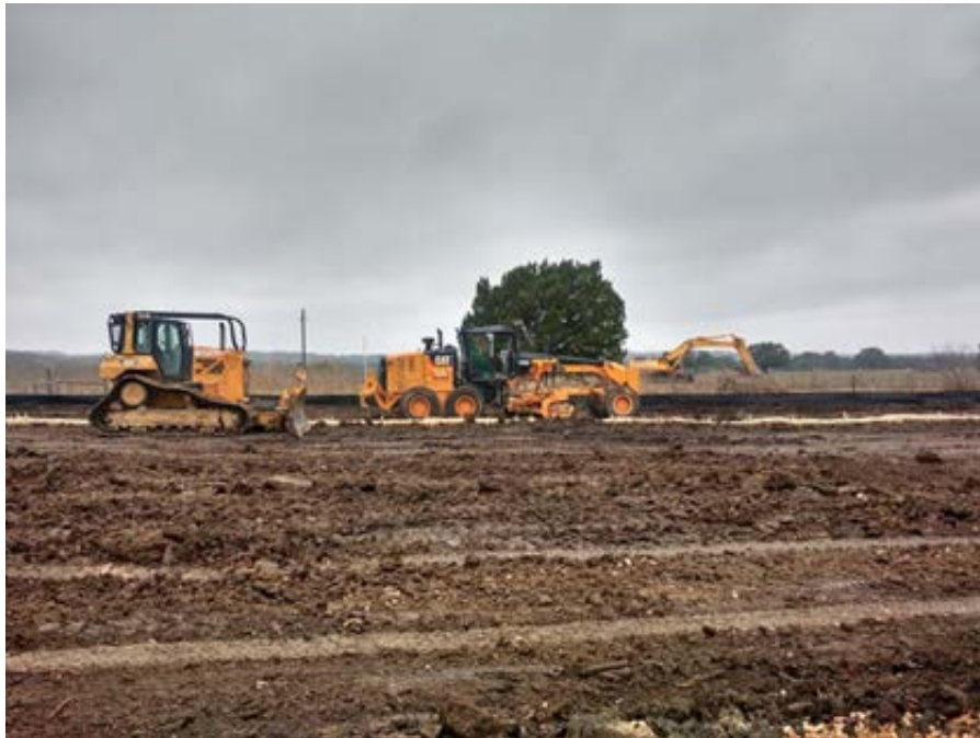
At GS1: Grading Haul Road
