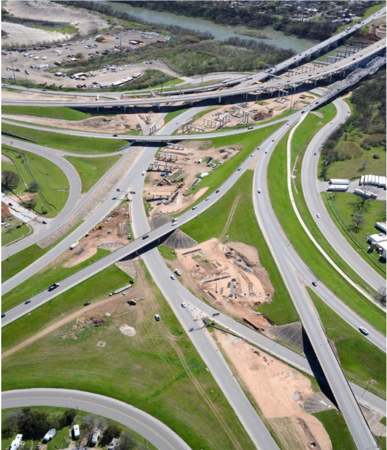
183 at Airport Blvd/7 th St/5 th St/1 st St (Looking Southeast)
