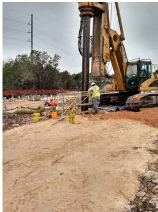
At GS1: Foundation Drilling at Bear Creek Bridge Bent 2
