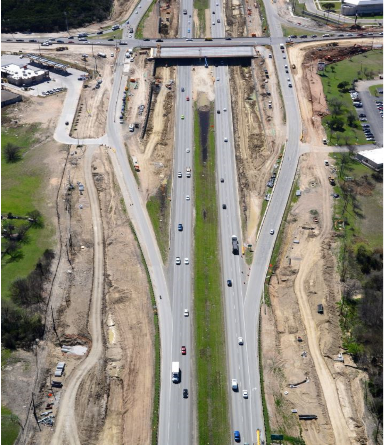
183 at FM 969/MLK Jr Blvd (Looking South)
