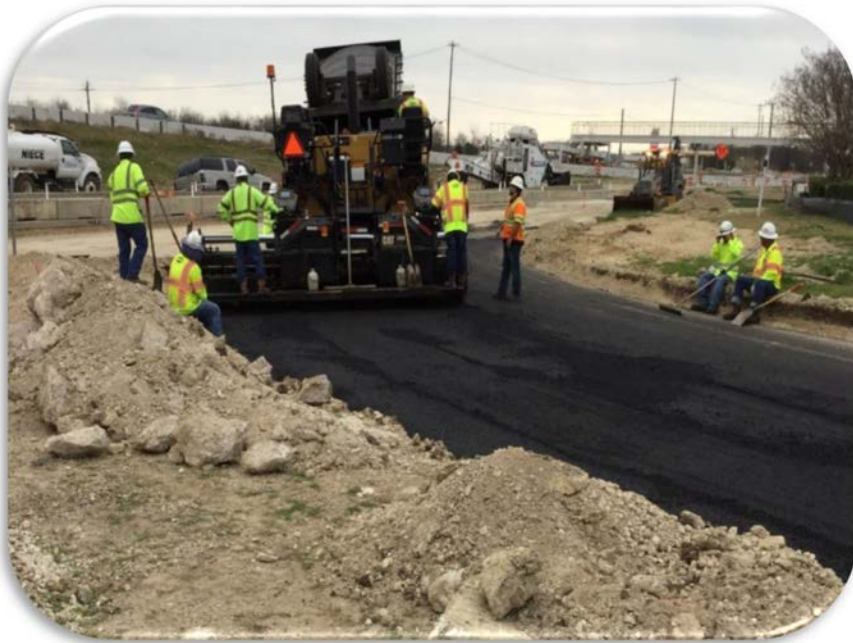
Hot Mix Asphalt near Manor/Springdale Road
