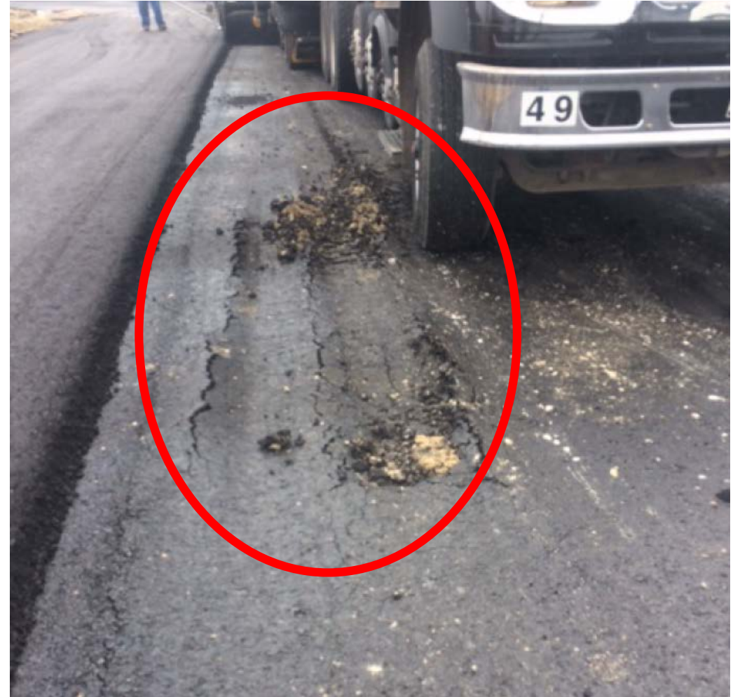
Subgrade failure
