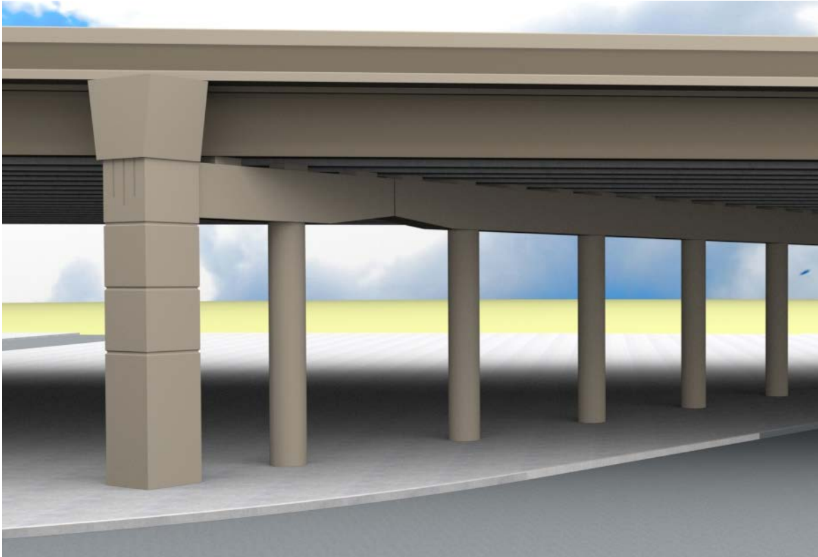
Decorative Column at Bridge with outside widening typ. Interior column cylindrical - exterior column decorative and structural connected to new cap - Skewed bent location
