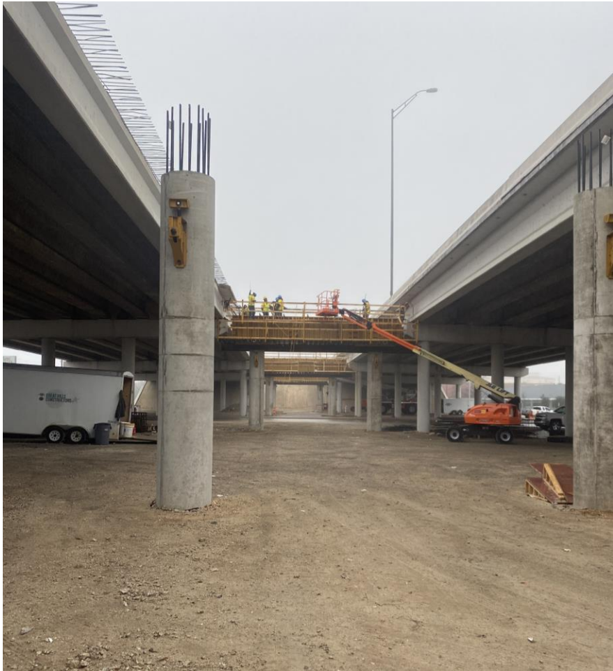
MCNEIL BRIDGE CAP
