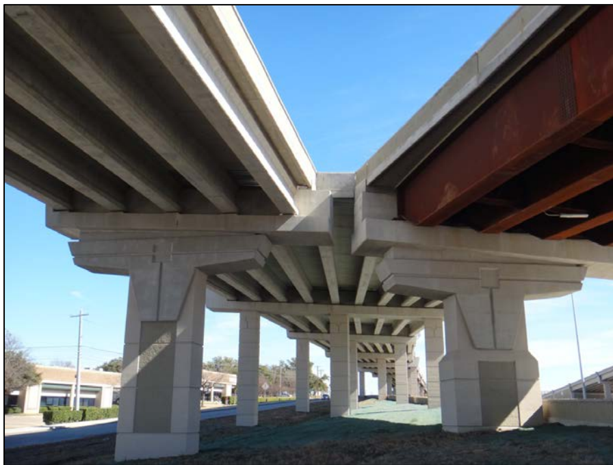
Westbound Manor Expressway bridges at the US 183 northbound and southbound split
