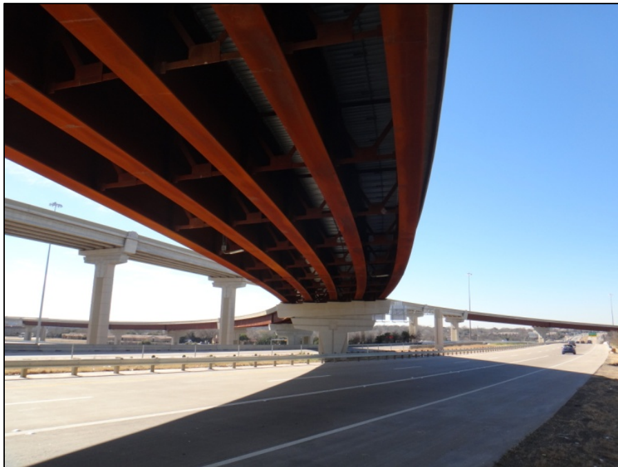
Mainlanes under the westbound US 290E to southbound US 183 Direct Connector
