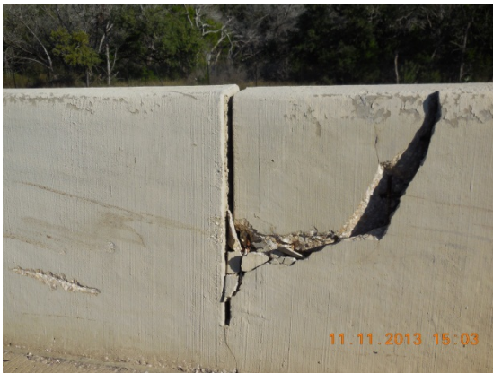
Northbound mainlane north of Avery Ranch Boulevard
