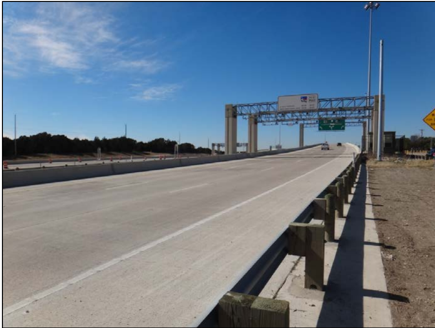
Manor Expressway Phase I approaching westbound toll gantries
