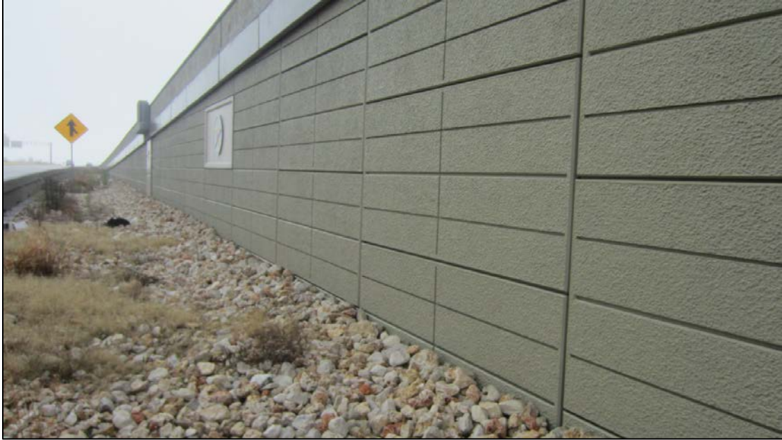
Retaining wall along the westbound Manor Expressway to southbound US 183 departure
