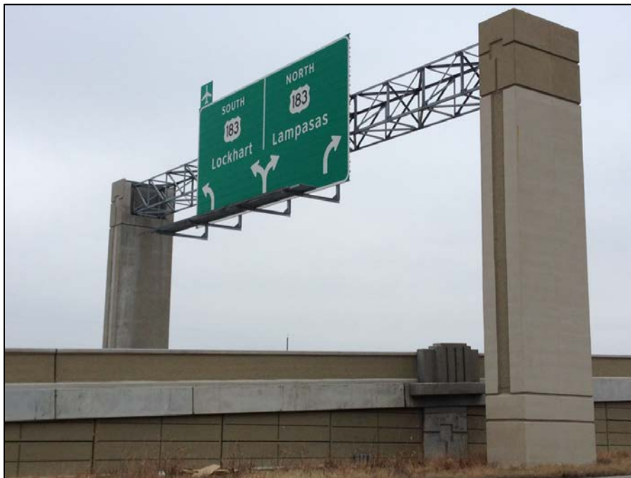
Overhead sign structure approaching westbound direct connectors
