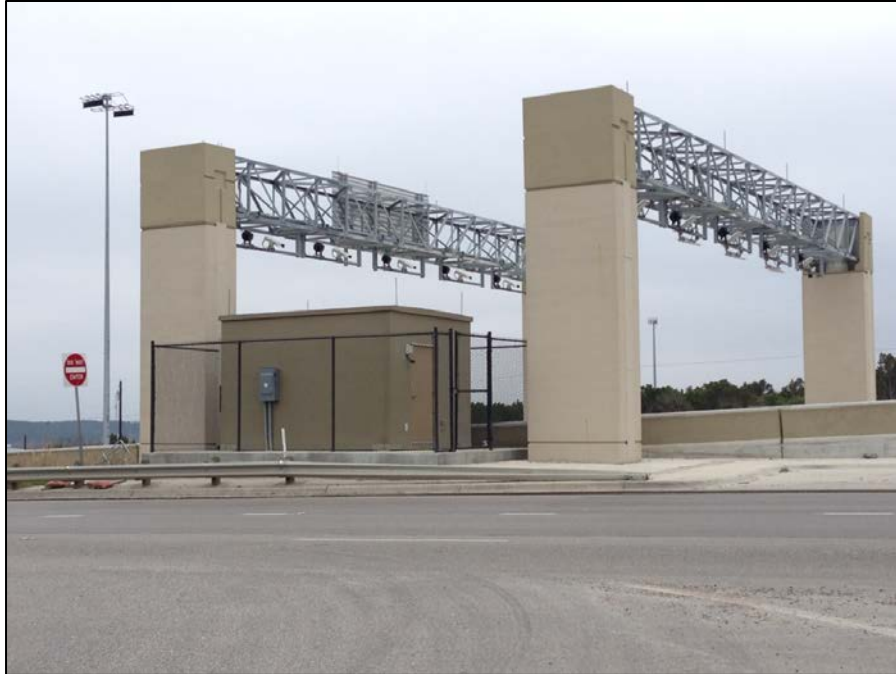
ILP building located at the Ramp 1 toll location
