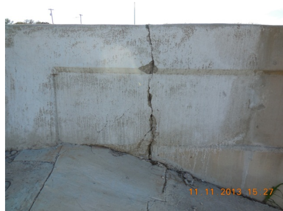
Northbound mainlane on south end of Spanish Oak Creek Bridge
