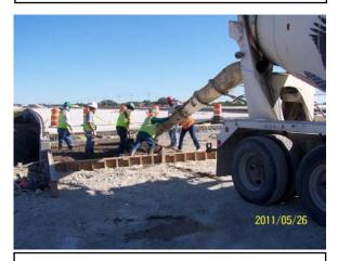
Placing supporting concrete for a bridge structure at Block House Creek
