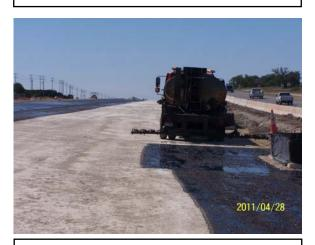
Placing asphalt on the cement-treated base near Block House Creek
