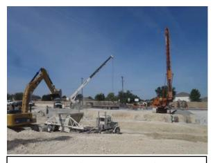
Drilled shaft construction at future Scottsdale Drive bridges
