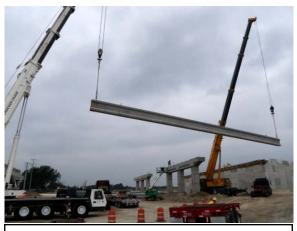
Placing beams at the 183A bridges over Hero Way
