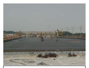
Preparing bridge deck for concrete placement at Block House Creek
