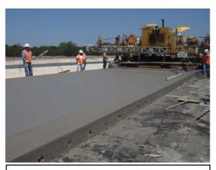
Applying surface finish to concrete pavement
