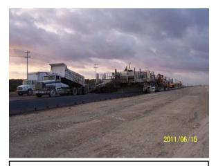
Placing concrete for paving on the mainlanes north of Crystal Falls Parkway
