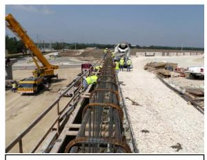
Placing concrete at a back wall for the 183A bridge over Hero Way
