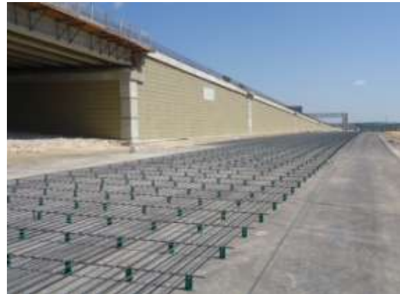
Westbound mainlane pavement near US 183 interchange (Looking East)
