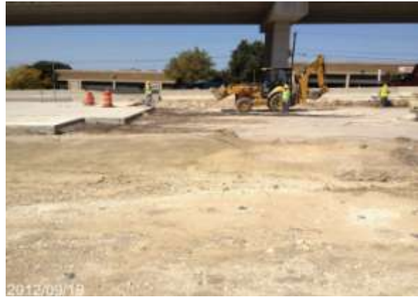
Completed US 290 Mainlane Concrete Paving (Looking North)
