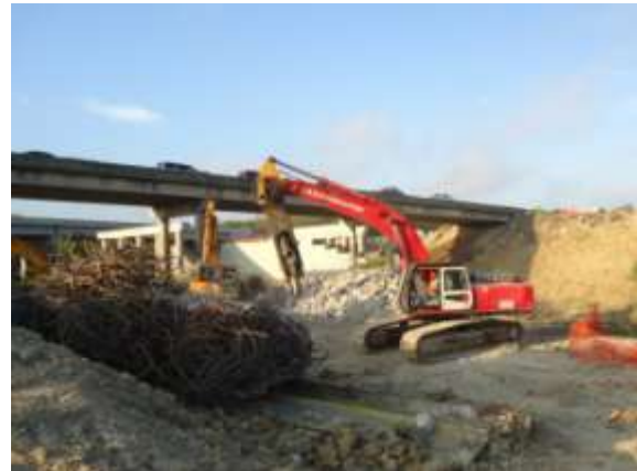
Demolition of westbound frontage road bridge at MOKAN crossing (Looking South)
