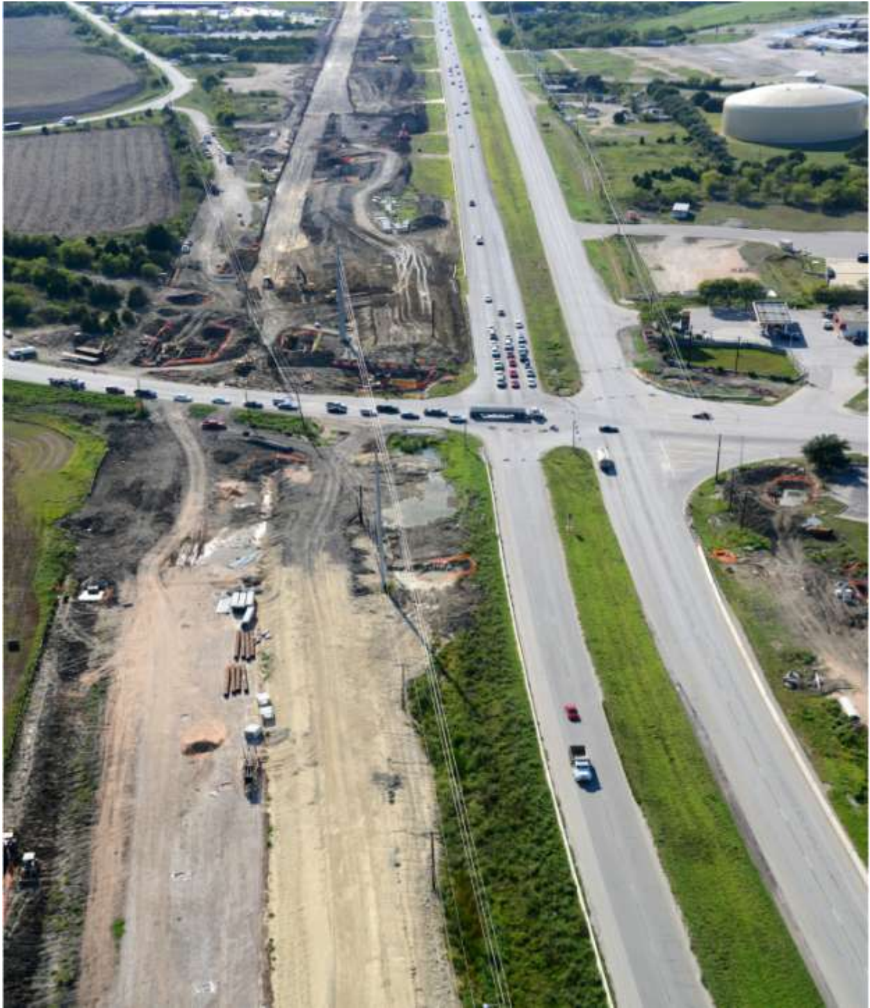
US 290 East at Giles Road Intersection looking west (Taken 9/21/2012)
