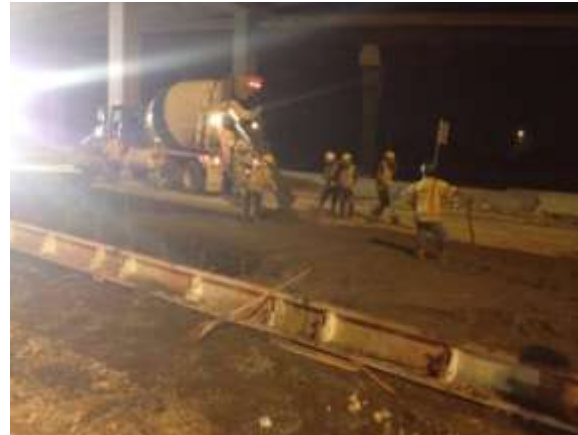
Placement of Concrete Paving Eastbound Mainlanes (Looking South)
