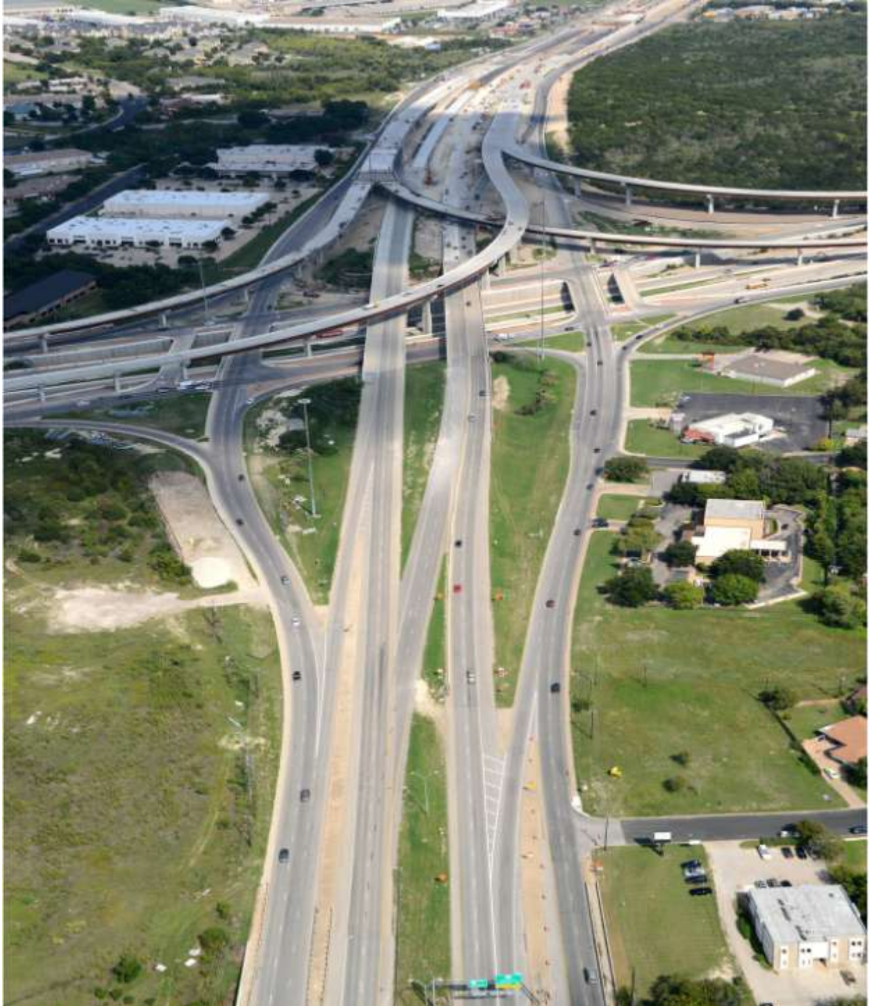
Manor Expressway Phase I Project (Looking East from US 290) (Taken 10/04/2012)
