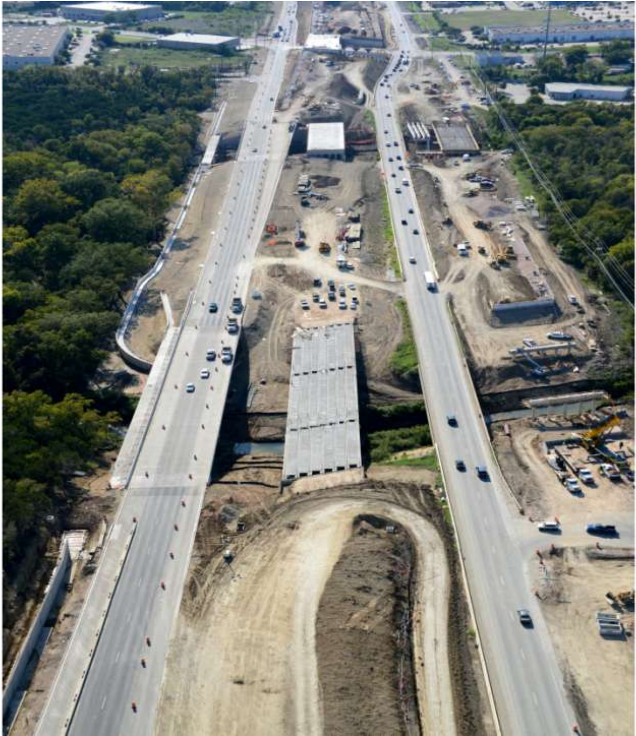
US 290 East at Chimney Hill Blvd looking west (Taken 9/21/2012)
