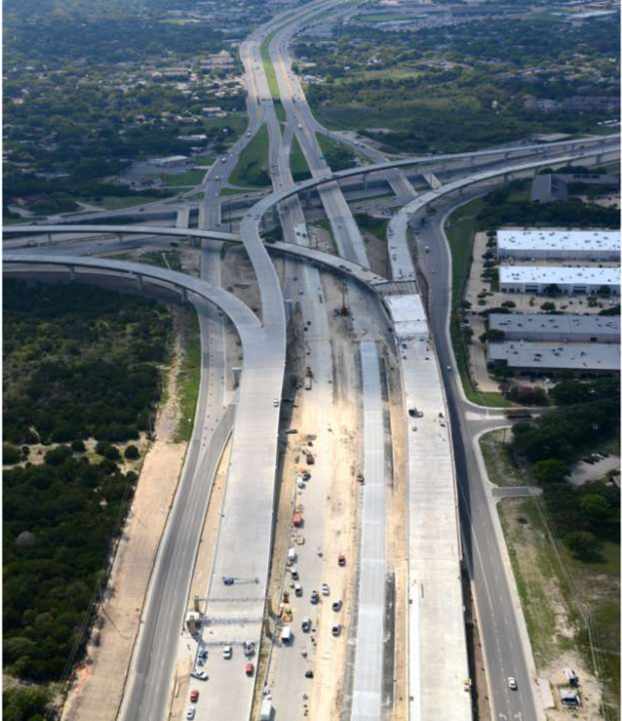
Manor Expressway Phase I Project (Looking West from US 290) (Taken 10/04/2012)
