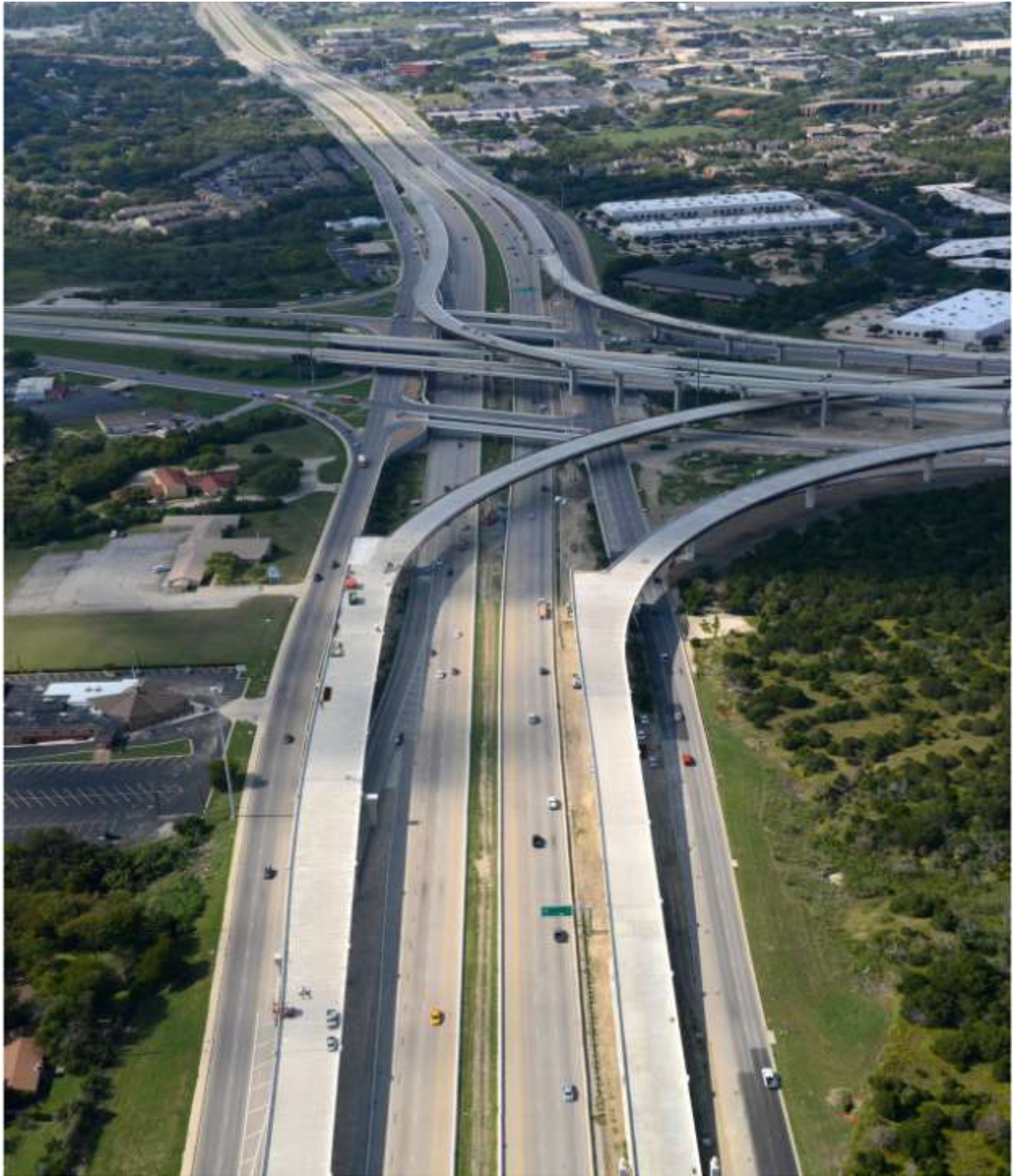
Manor Expressway Phase I Project (Looking North from US 183) (Taken 10/04/2012)
