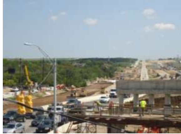
Westbound frontage road (at left) from Springdale intersection (Looking East)
