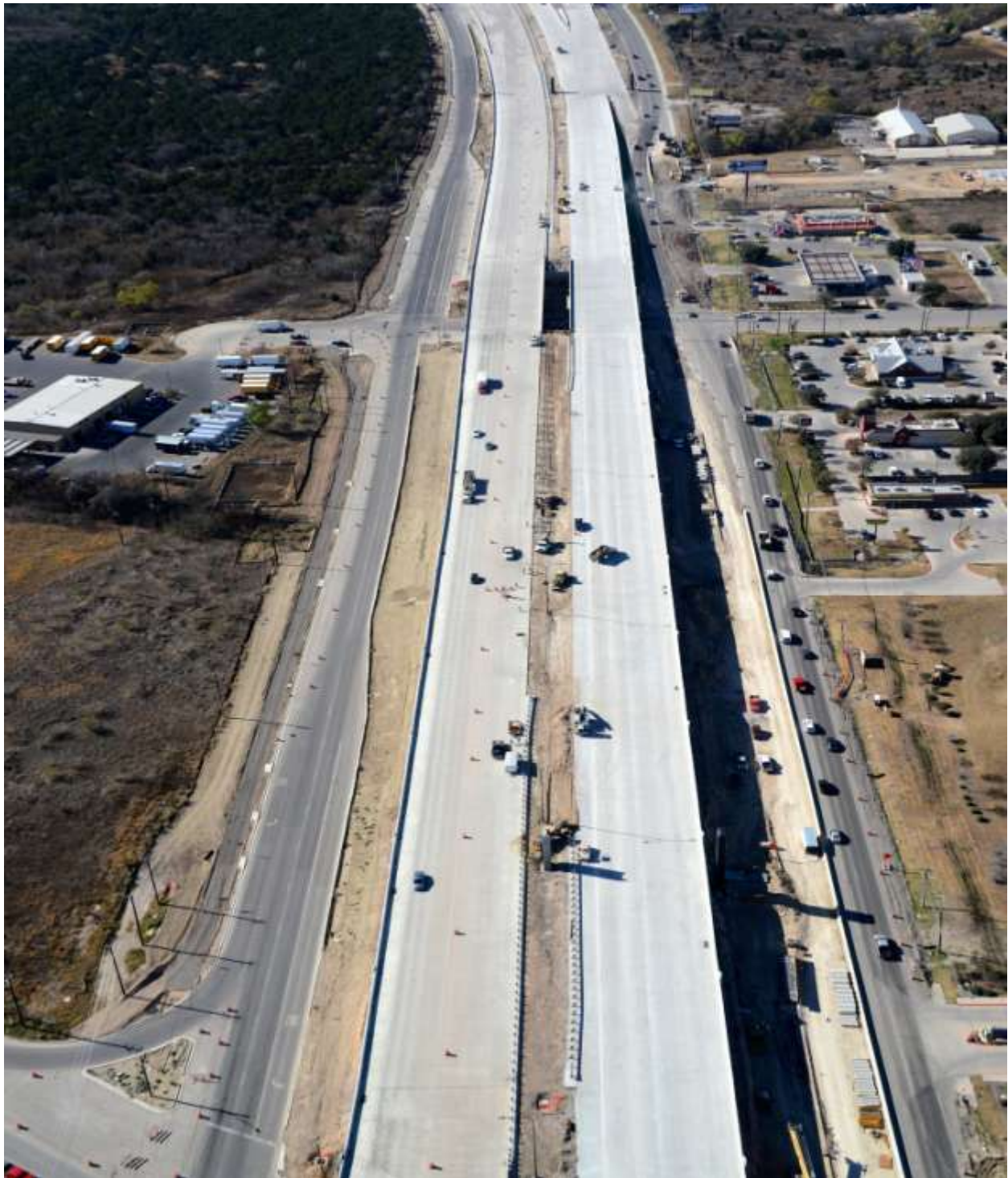
US 290 East at Springdale Road looking west (Taken 12/18/2012)
