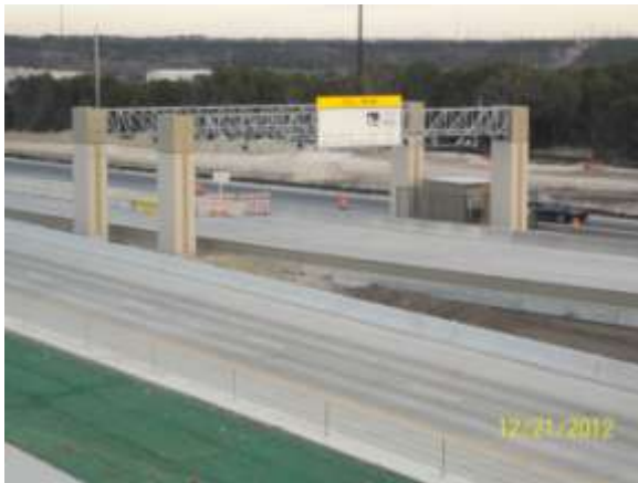
Completed South to East Toll Plaza and 290 EBML (Looking Southeast)
