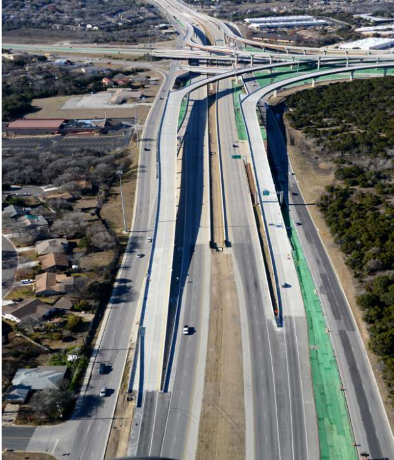
Manor Expressway Phase I Project (Looking North from US 183) (Taken 1/10/2013)
