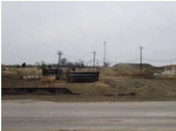
Installation of underground utilities west of Parmer Lane (Looking East)
