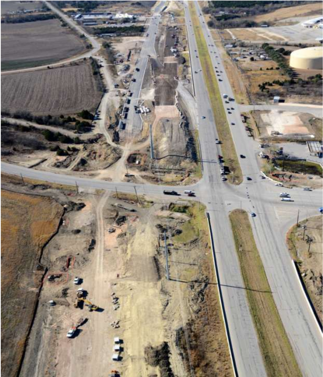
US 290 East at Giles Road Intersection looking west (Taken 12/18/2012)
