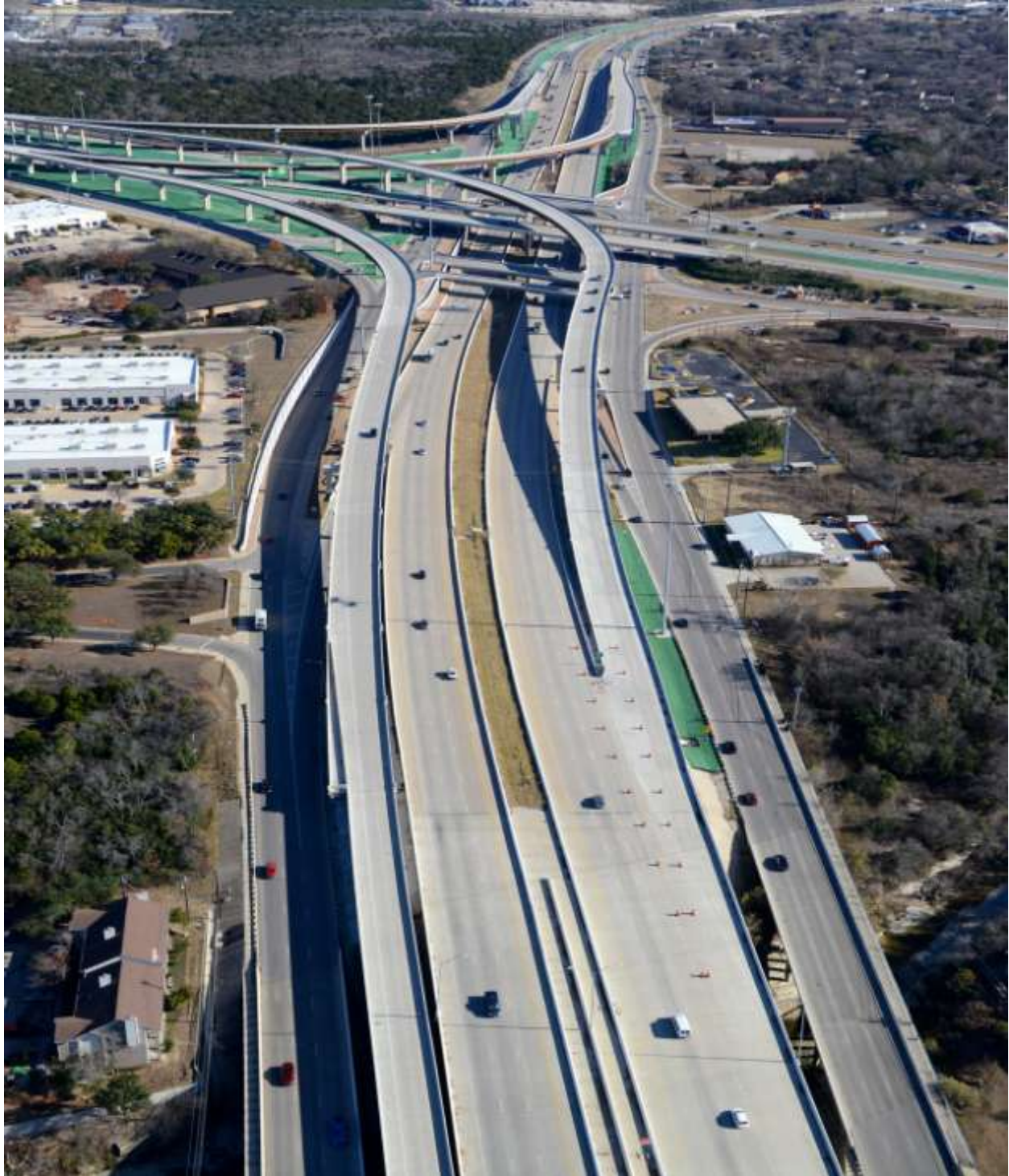
Manor Expressway Phase I Project (Looking South from US 183) (Taken 1/10/2013)
