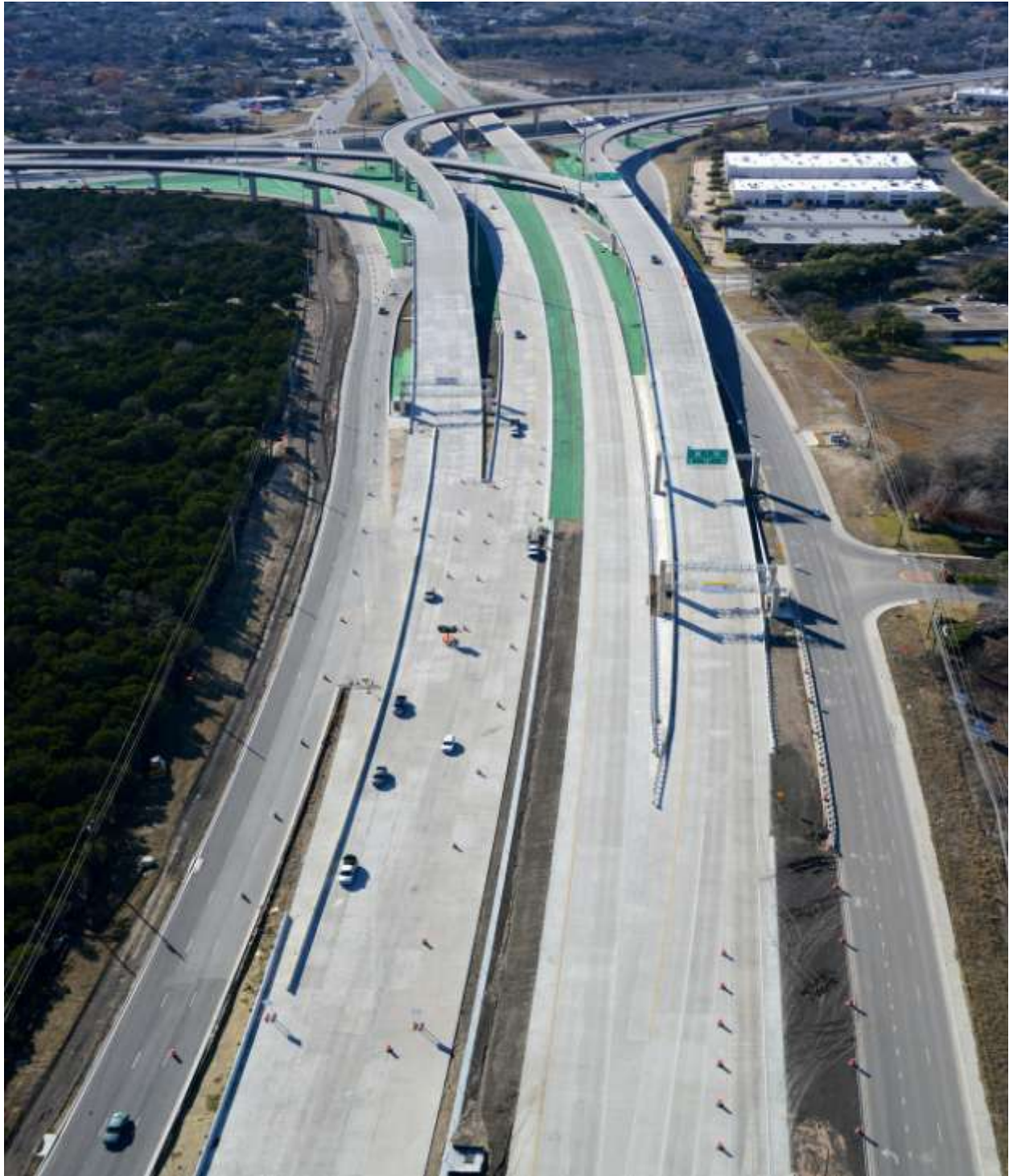
Manor Expressway Phase I Project (Looking West from US 290) (Taken 1/10/2013)
