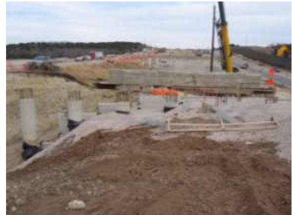
Placement of backfill behind Wall S2-10 (Looking East)
