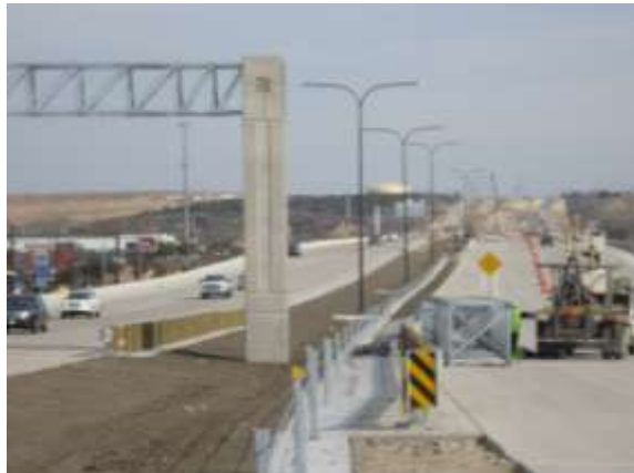
Completed eastbound and westbound mainlanes (Looking East)
