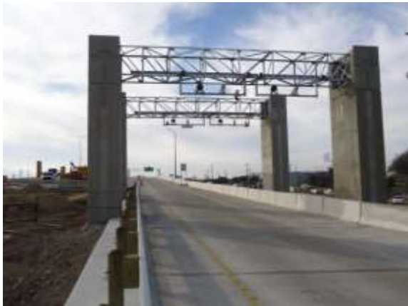
Ramp #3 Toll Gantry – westbound tolling point for Interim Development Work (Looking West)
