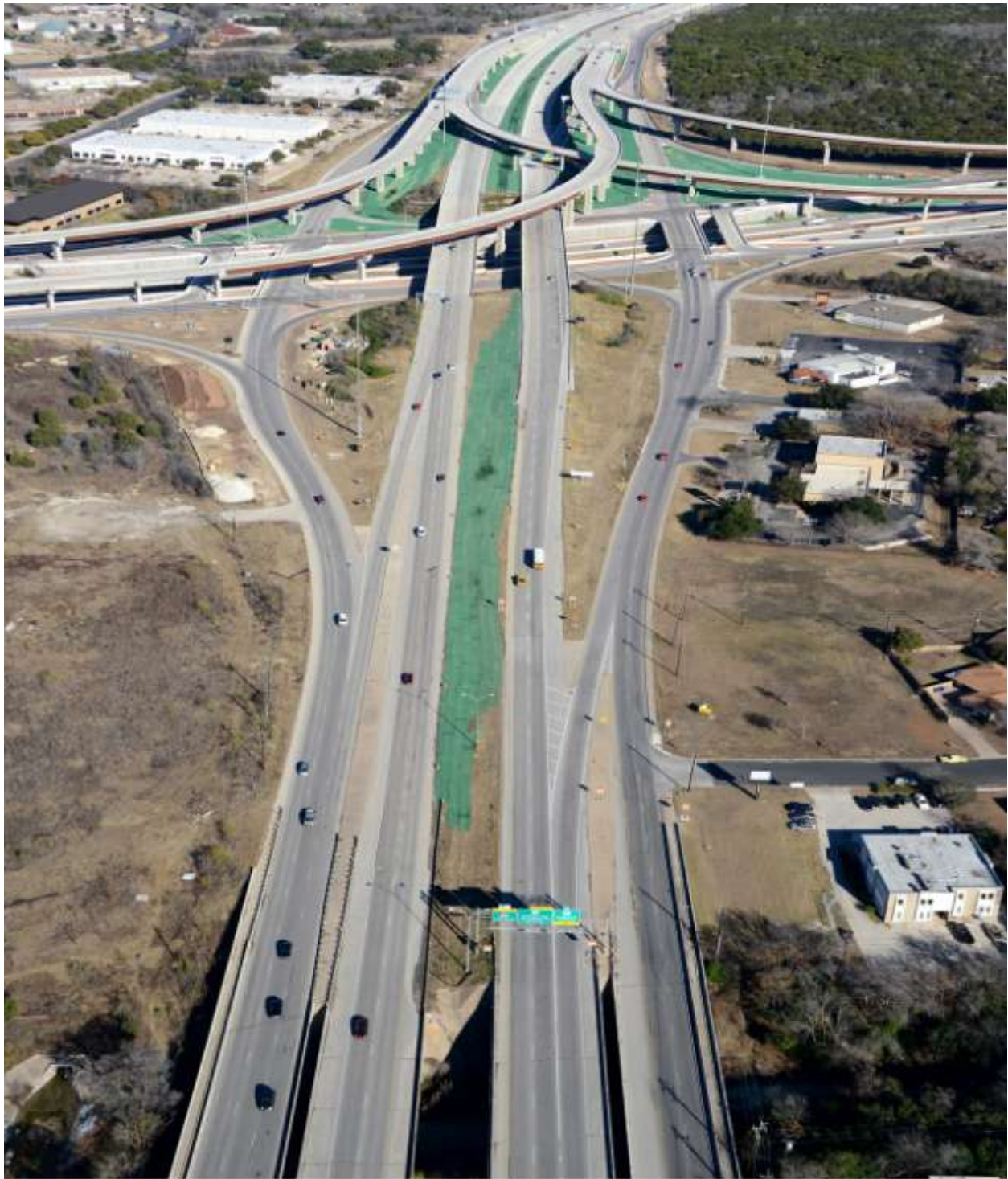
Manor Expressway Phase I Project (Looking East from US 290) (Taken 1/10/2013)
