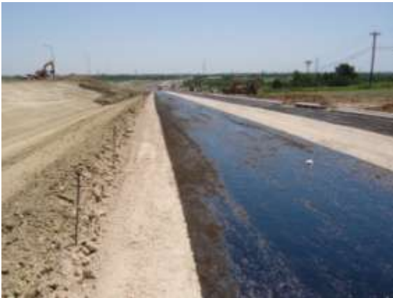
Prime coat placement west of Parmer Lane (Looking East)
