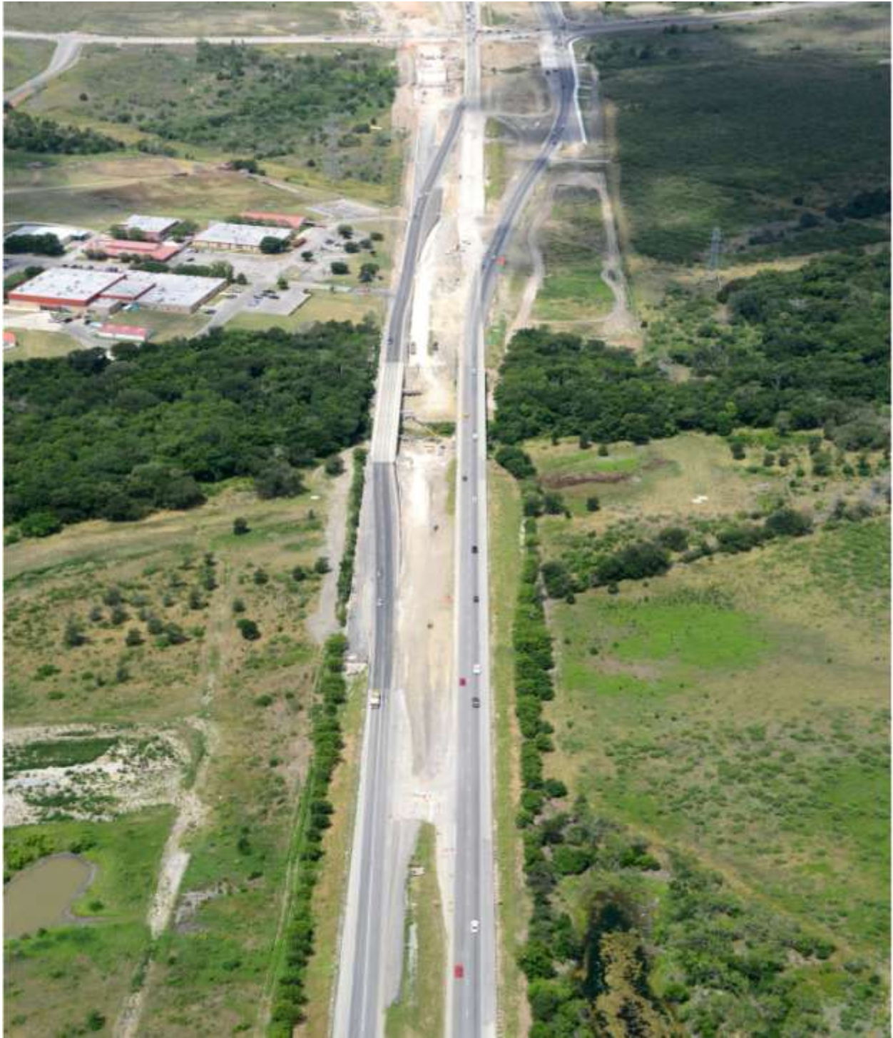
US 290 East looking west from Gilleland Creek (Taken 6/24/2013)
