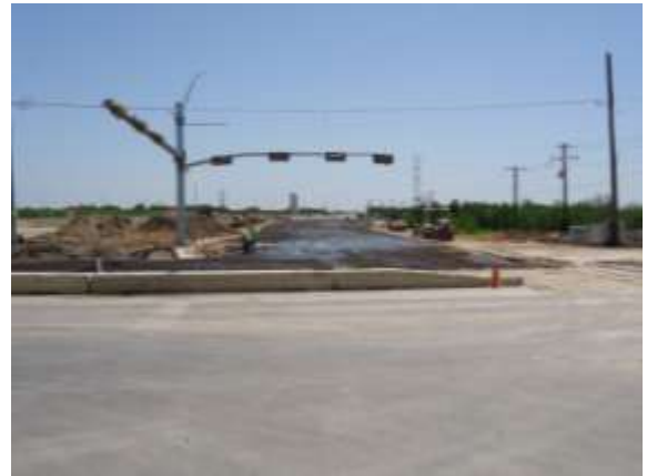
Eastbound frontage road construction east of Parmer Lane (Looking East)
