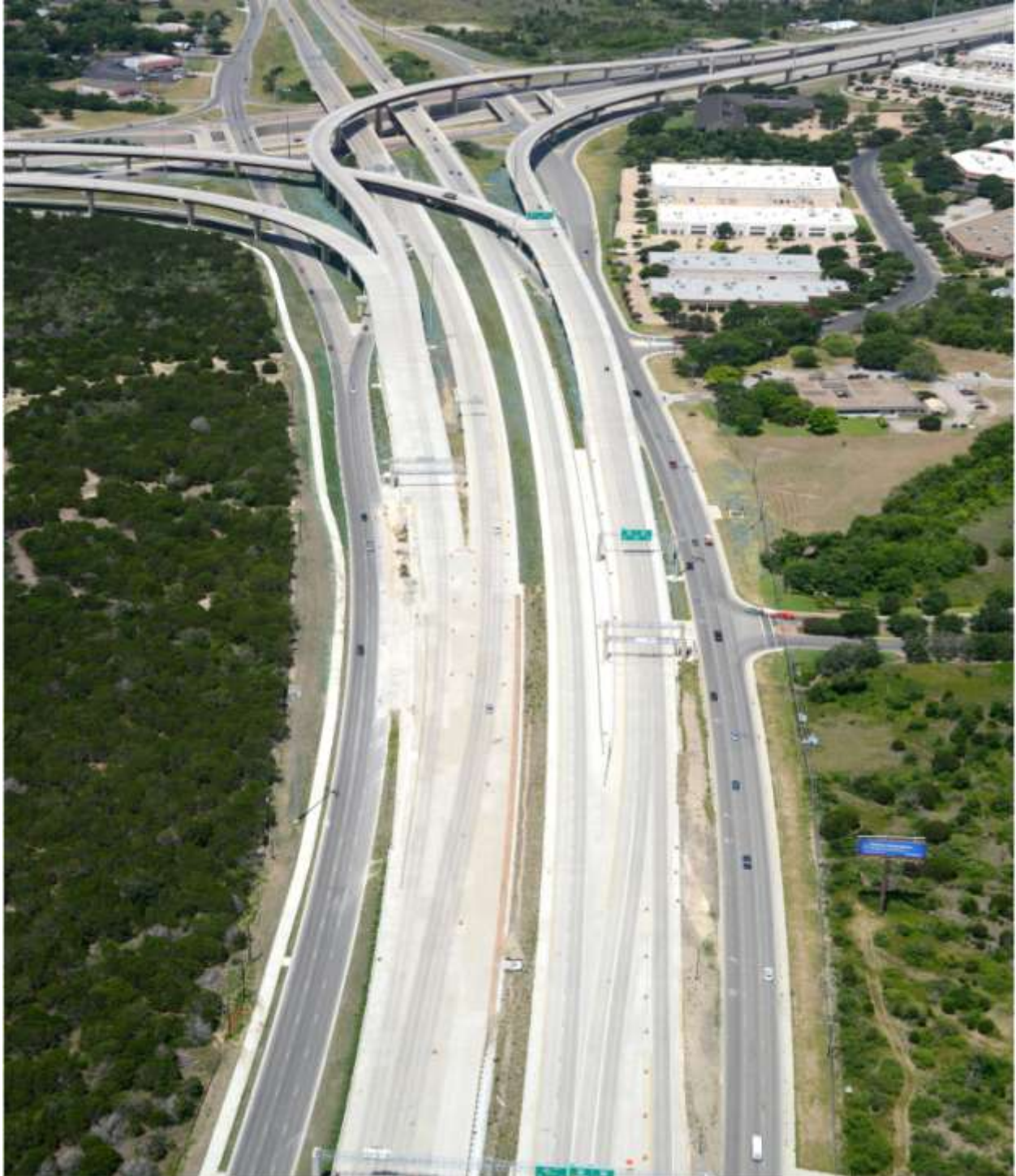
US 290 East at Tuscany Way looking west (Taken 6/24/2013)
