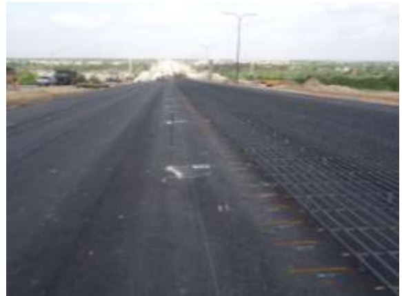
Tied steel for concrete pavement on the eastbound mainlanes (Looking West)
