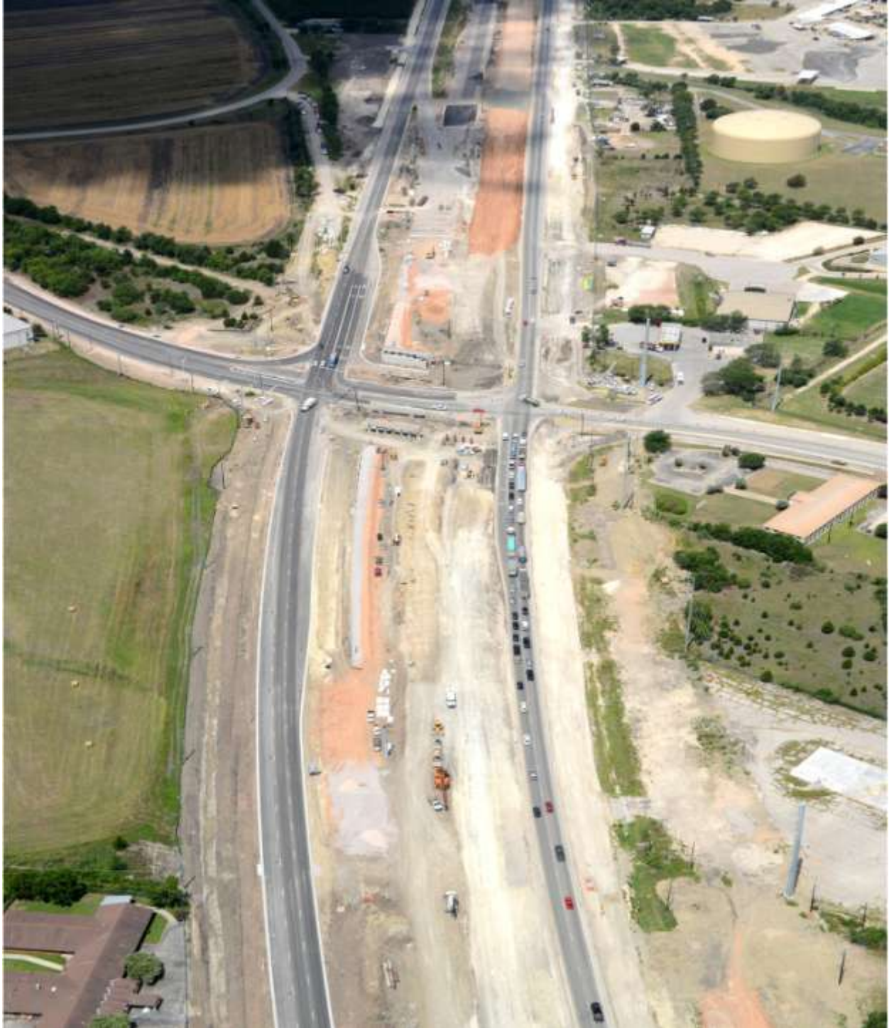
US 290 East at Giles Road Intersection looking west (Taken 6/24/2013)
