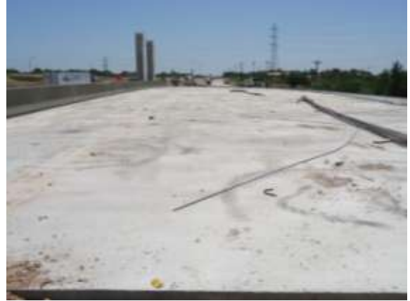
Construction of Eastbound frontage road bridge at Tributary #1C (Looking East)
