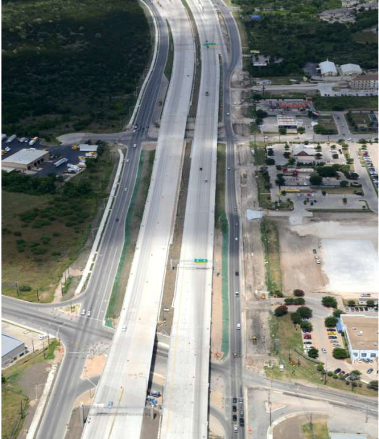
US 290 East at Springdale Road looking west (Taken 6/24/2013)
