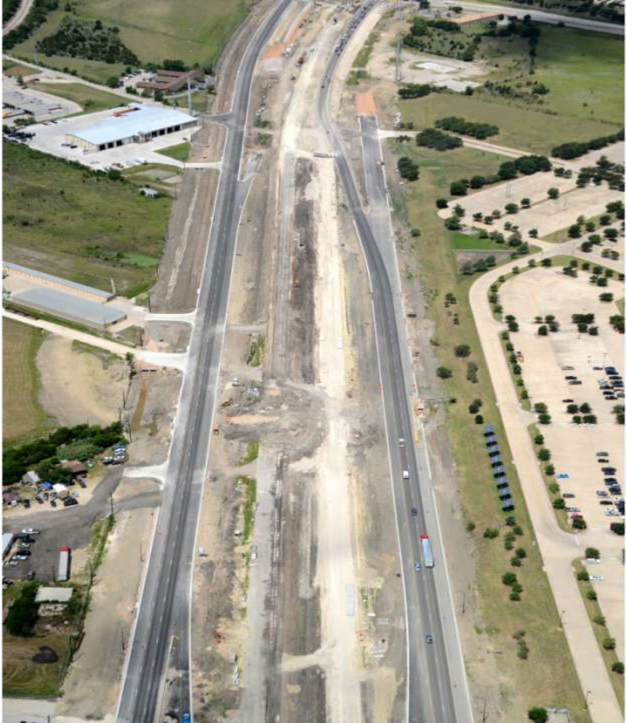
US 290 East at Crofford Lane Intersection looking west (Taken 6/24/2013)
