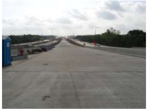
Concrete pavement on the eastbound mainlanes near Walnut Creek (Looking East)
