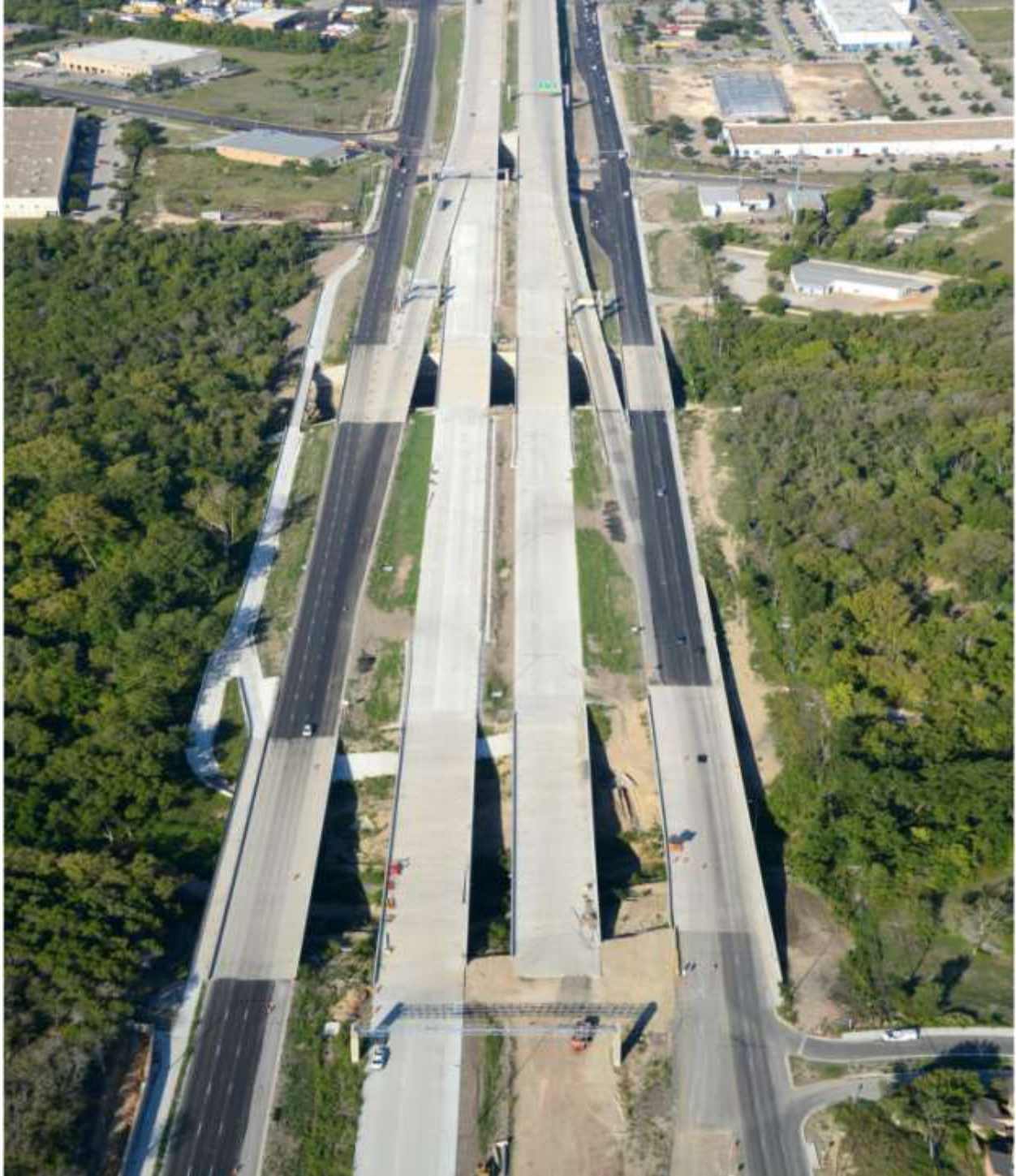
US 290 East at Chimney Hill Blvd looking west (Taken 9/25/2013)
