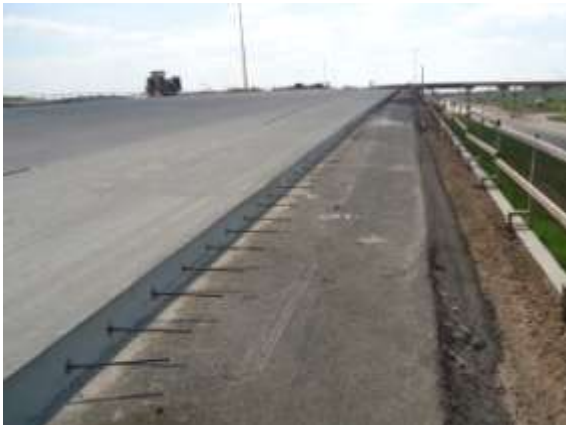
Concrete paving poured on the westbound mainlanes near SH 130 (Looking West)
