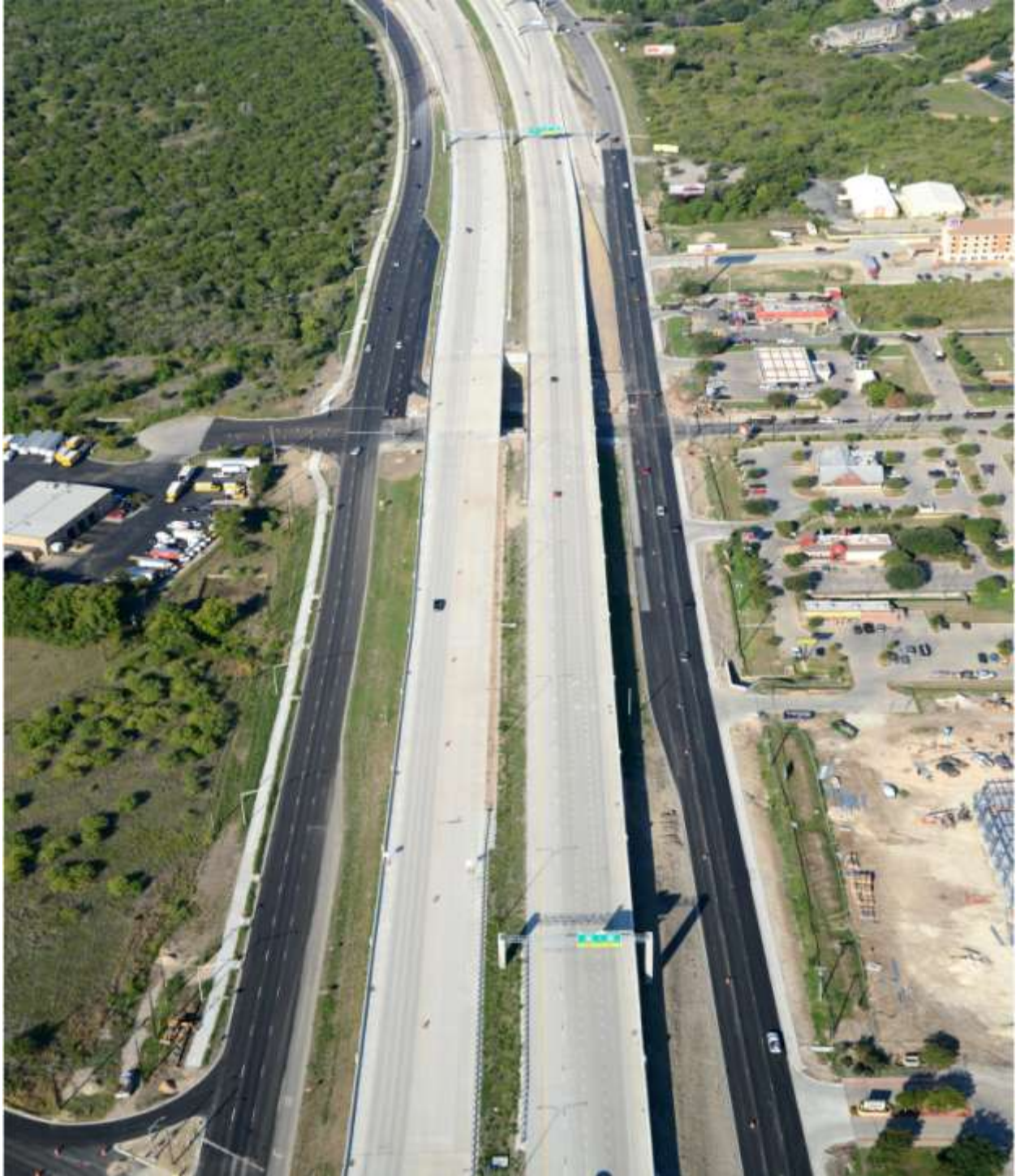
US 290 East at Springdale Road looking west (Taken 9/25/2013)
