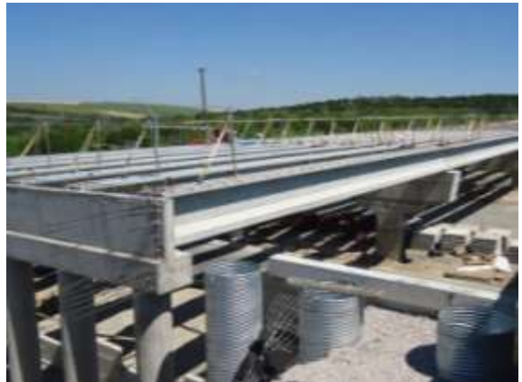
Construction of the westbound mainlane bridge at Arterial "A" (Looking East)
