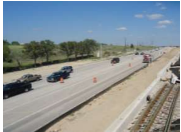
Westbound frontage road near completion east of Harris Branch (Looking Northeast)
