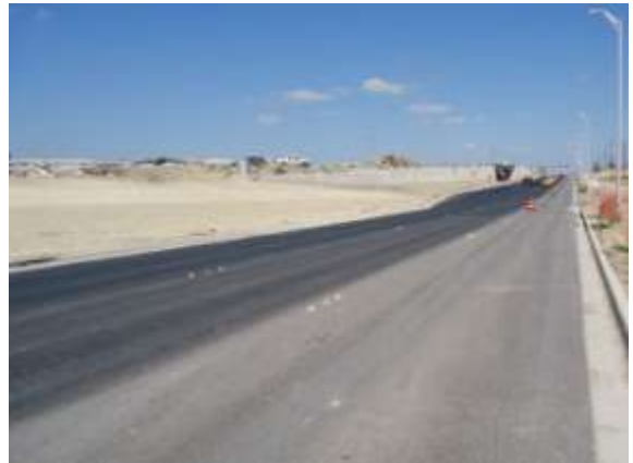
SMA placed west of the Harris Branch Parkway intersection (Looking East)
