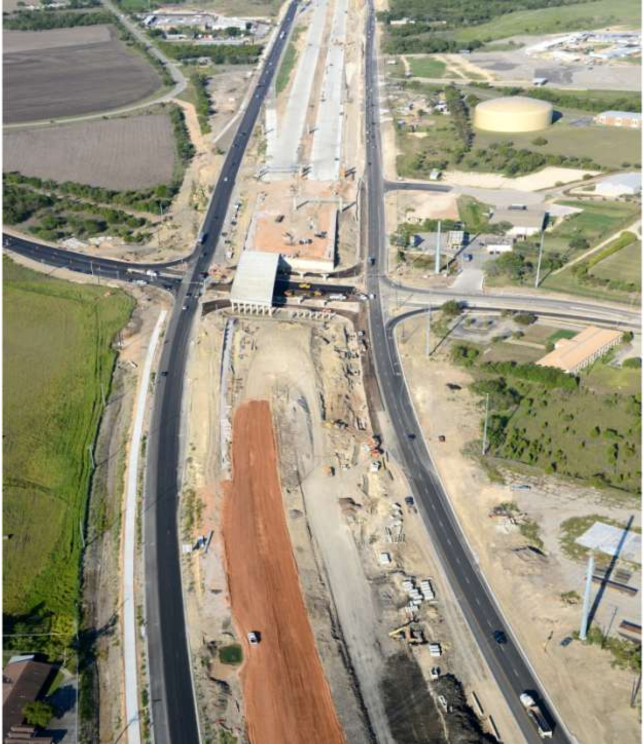
US 290 East at Giles Road Intersection looking west (Taken 9/25/2013)
