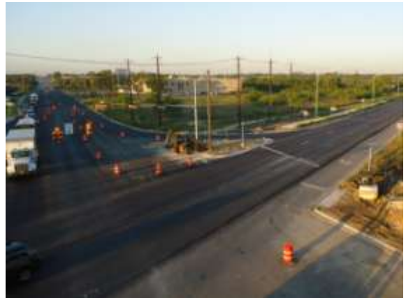
SMA has been placed at the Springdale Road intersection (Looking Southwest)
