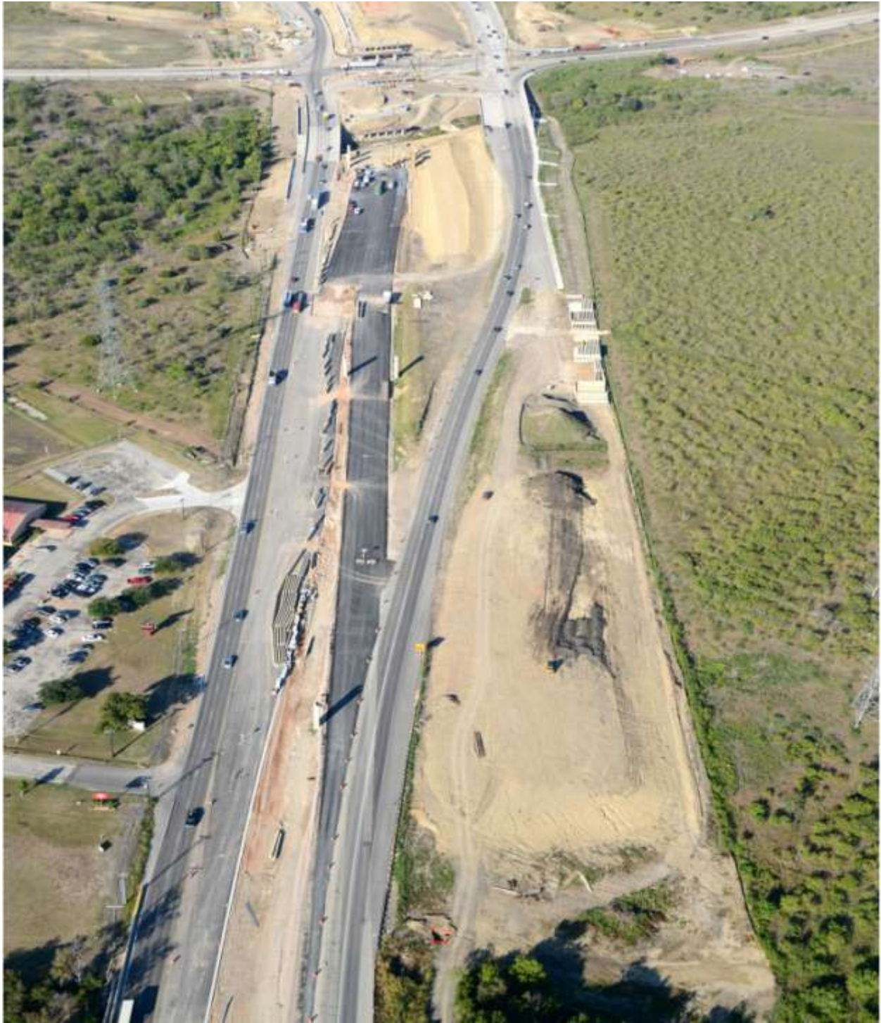
US 290 East looking west from Gilleland Creek (Taken 9/25/2013)
