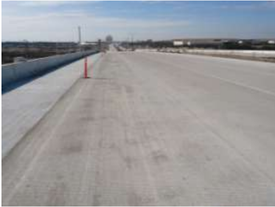
Concrete paving east of Harris Branch Parkway (Looking West)
