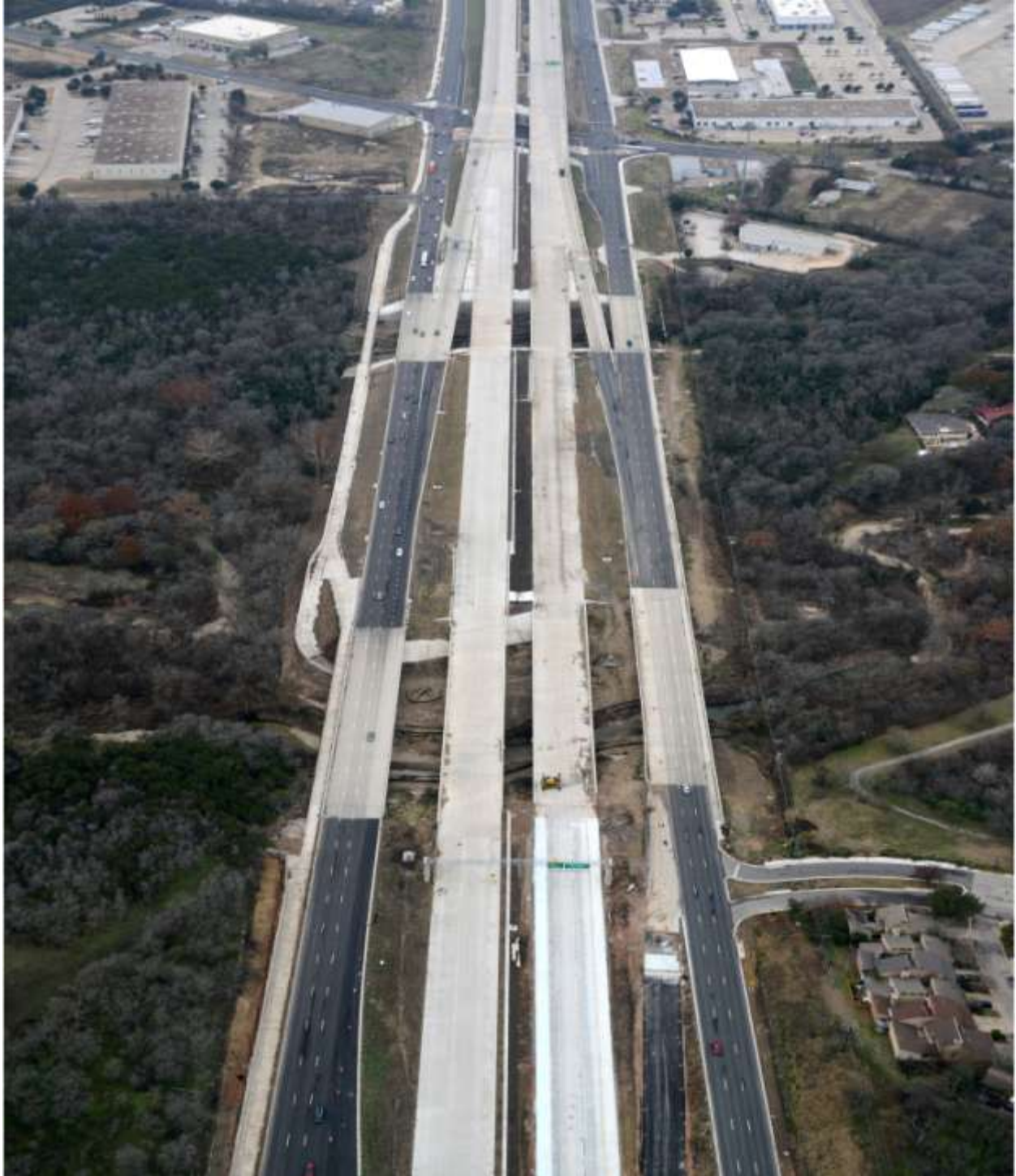
US 290 East at Chimney Hill Blvd looking west (Taken 12/16/2013)
