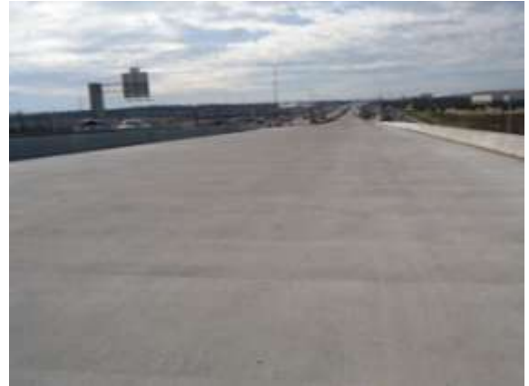
Concrete paving west of the Harris Branch Parkway intersection (Looking West)
