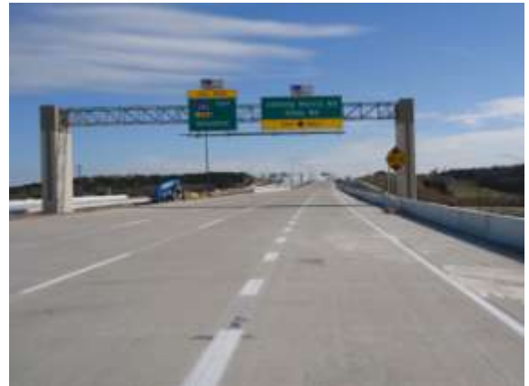
The overhead sign bridge has been installed near Arterial "A" (Looking East)
