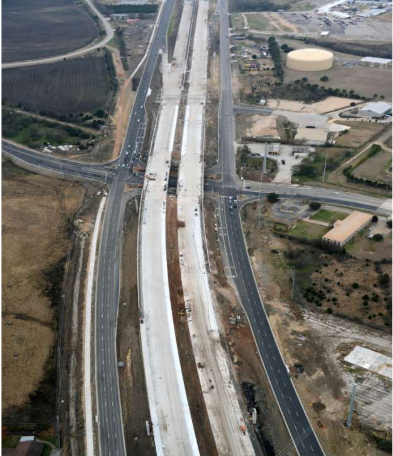
US 290 East at Giles Road Intersection looking west (Taken 12/16/2013)
