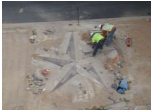
Hardscape pavers being installed at the Springdale Road intersection (Looking East)
