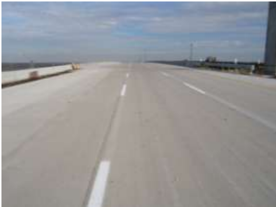
Concrete paving west of the SH 130 interchange (Looking West)
