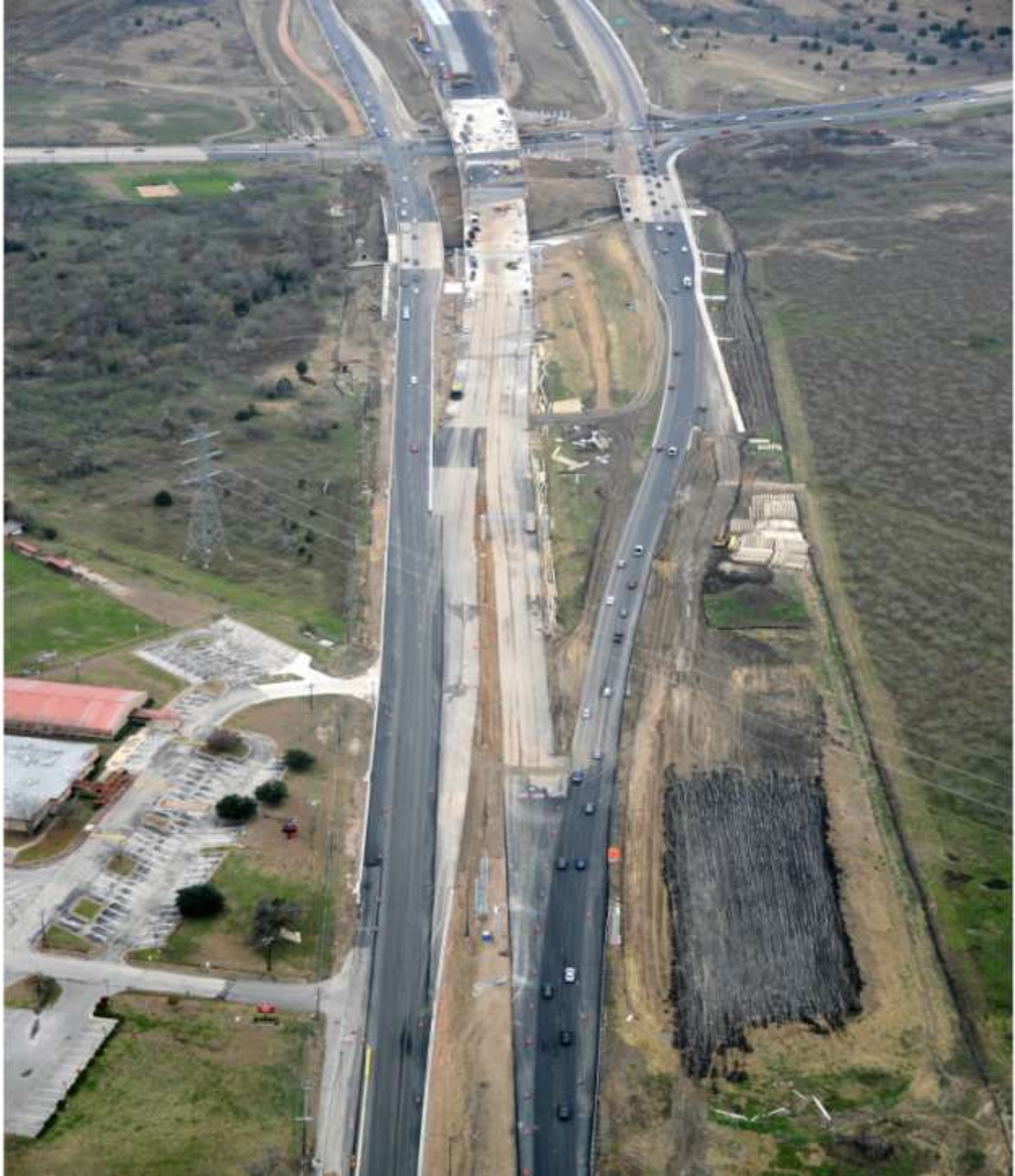
US 290 East looking west from Gilleland Creek (Taken 12/16/2013)
