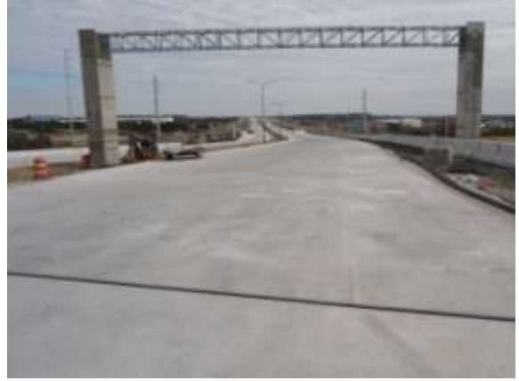
Concrete paving east of Giles Road (Looking East)
