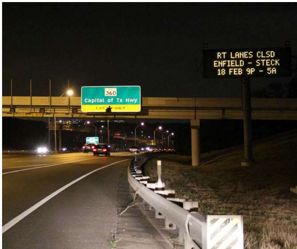
Advance signage for night-time lane closures on MoPac.
