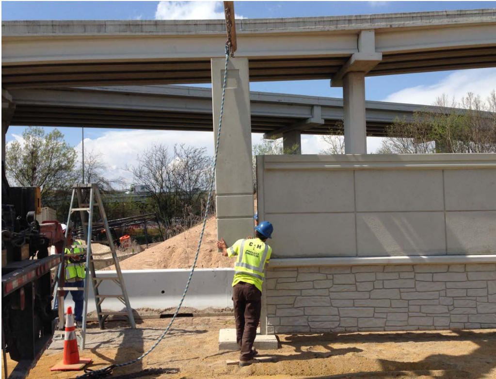
Sound wall mock-up installation.
