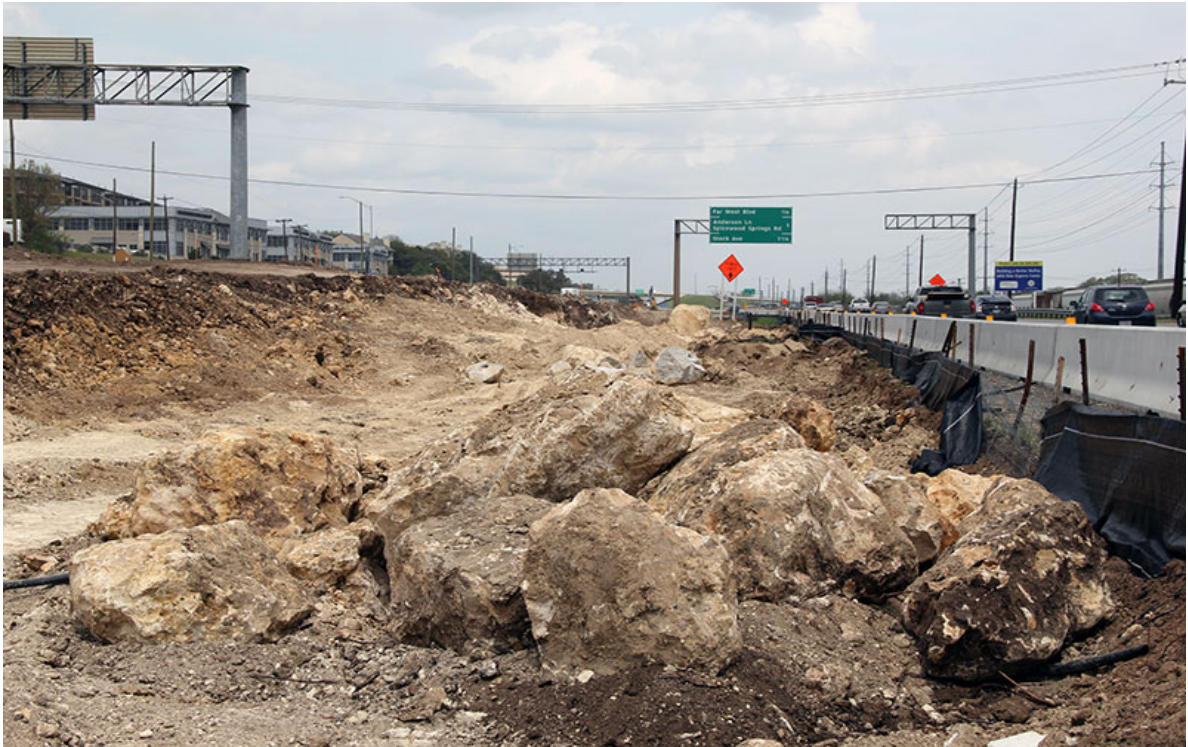
Heavy rock excavation to clear and grade the median north of RM 2222.
