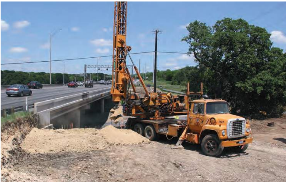
Construction of the MoPac Express Lanes
