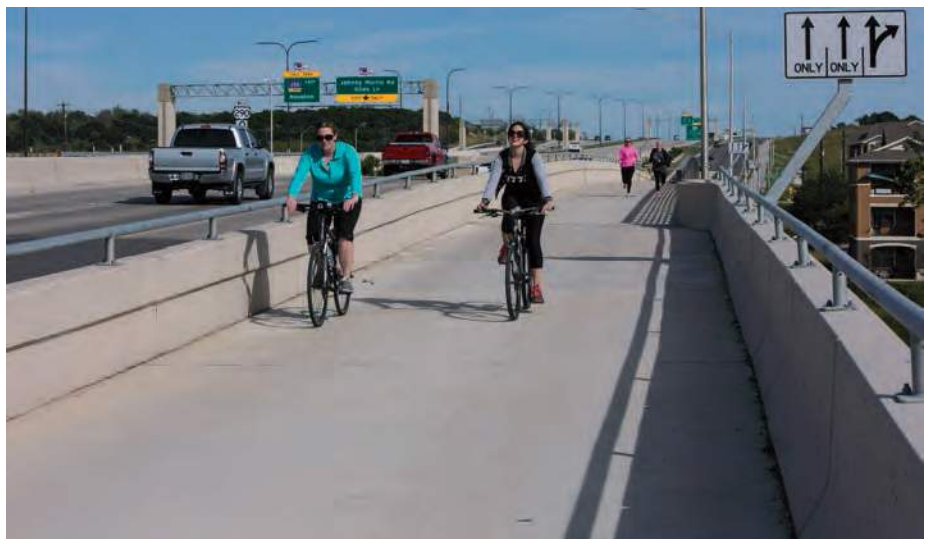
290 Toll (Manor Expressway – top) as well as the adjacent shared use (hike and bike path – above)
