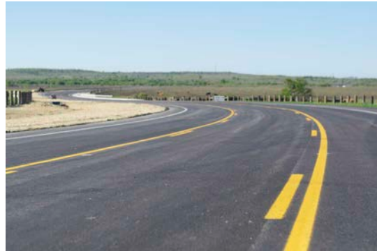
Kellam Rd. open to traffic
