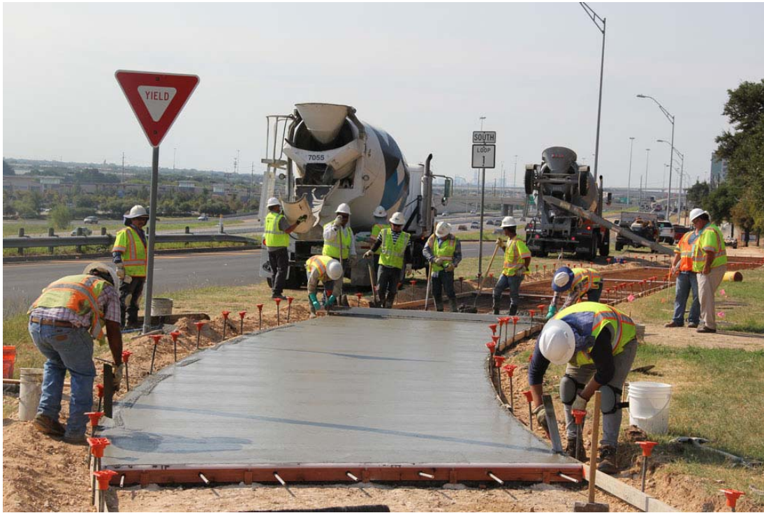
Shared Use Path Construction – October 2015
