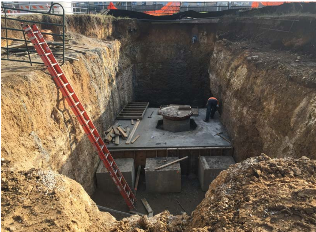
Boring for 42" Waterline at Camp Mabry – December 2015
