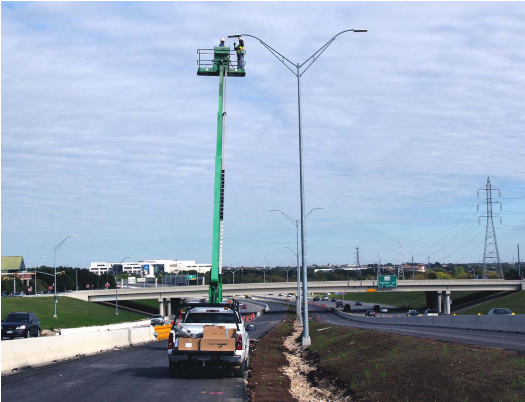
Installation of LED Roadway Illumination – November 2015
