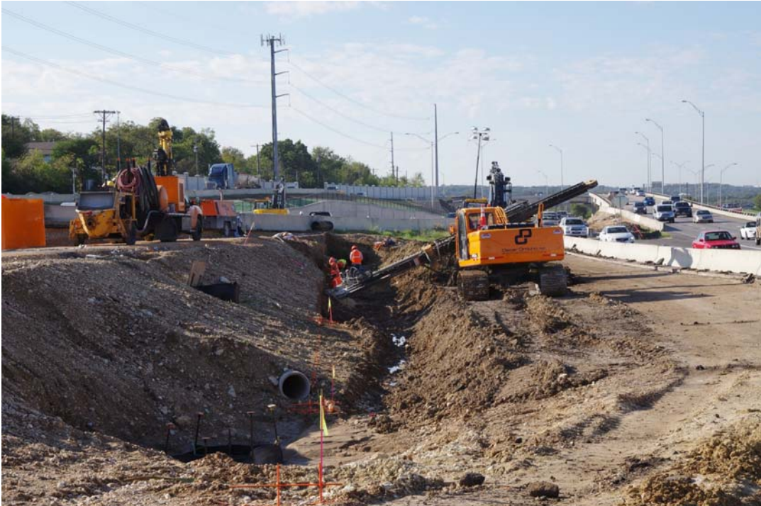
Northbound Undercrossing Excavation Shoring – October 2015
