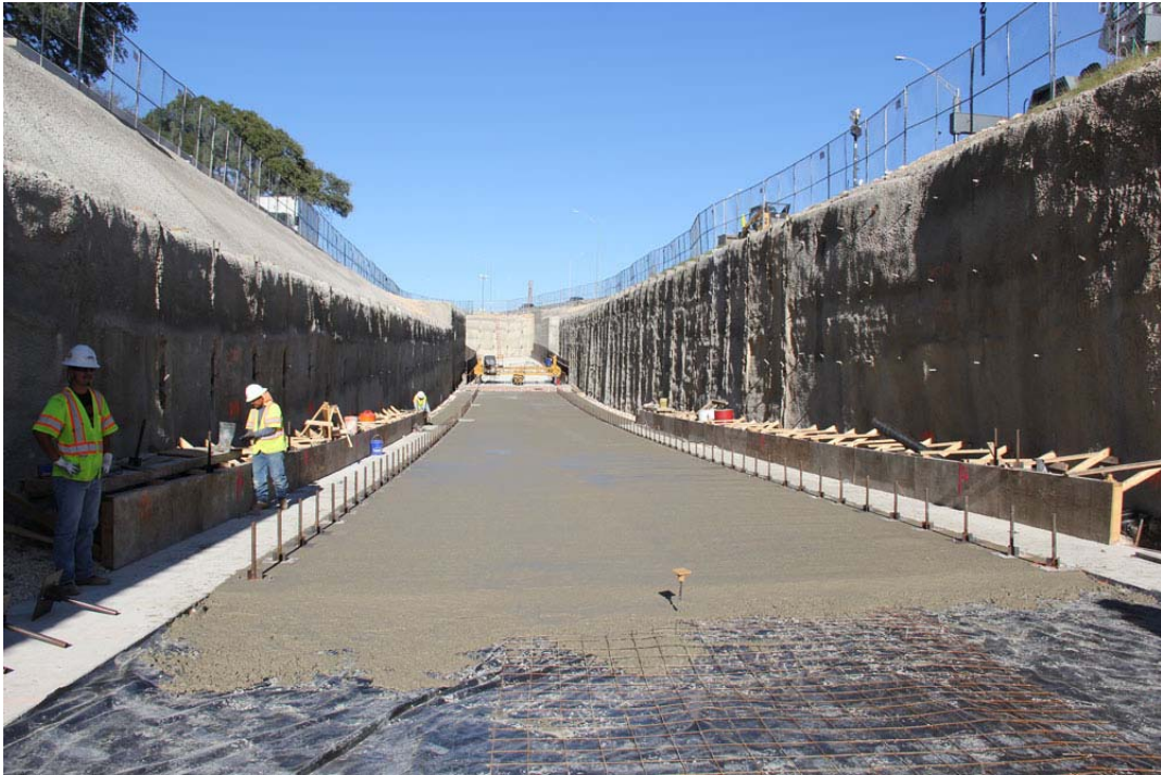
Southbound Undercrossing Construction – December 2015
