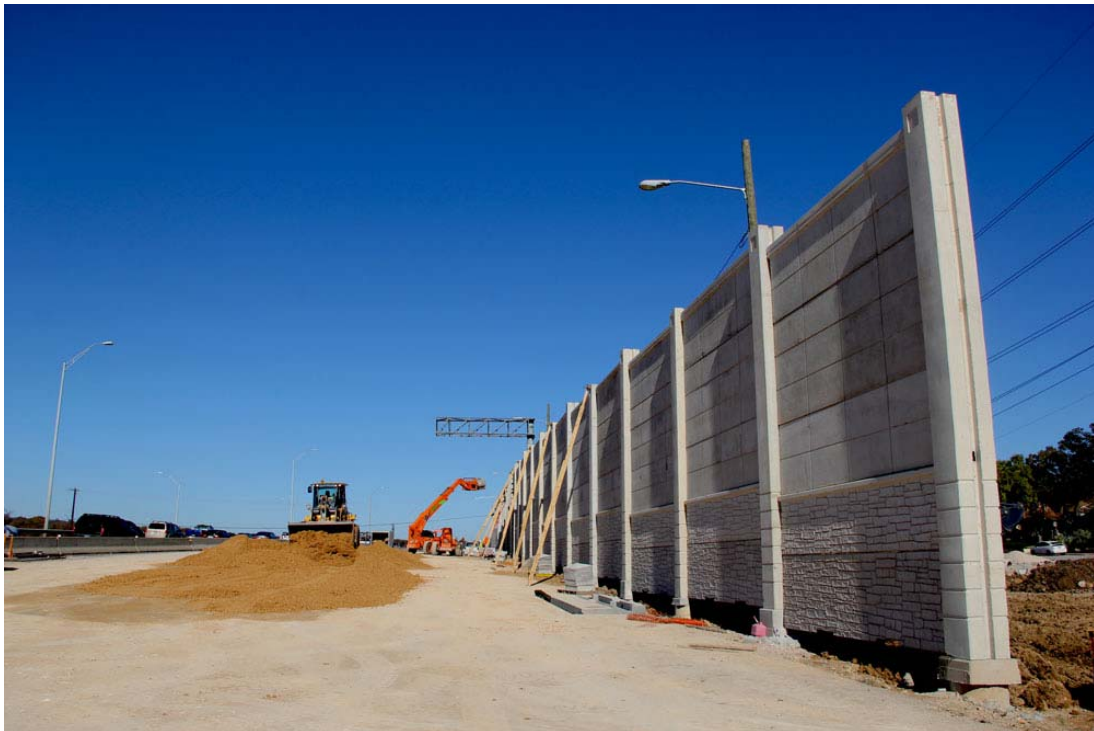
Sound Wall Construction – December 2015
