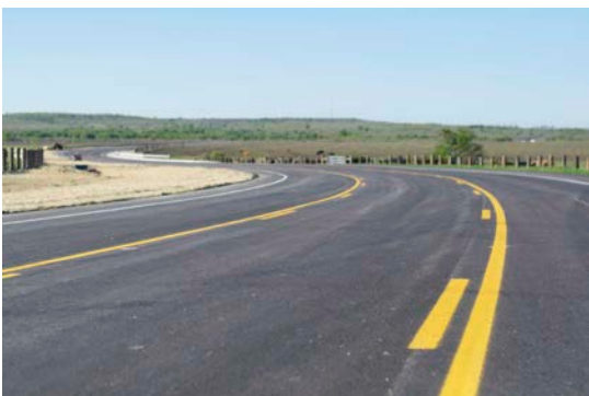
Kellam Rd. open to traffic
