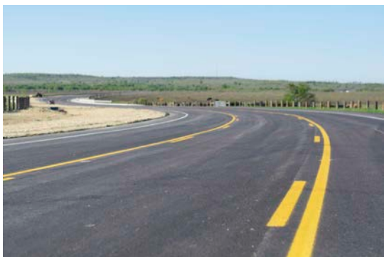
Kellam Rd. open to traffic
