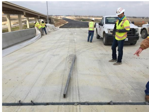
Bridge over SH 130 completed
