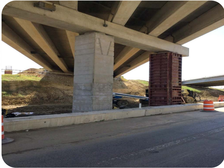
Column Work at Springdale/Manor (round columns to rectangular columns)
