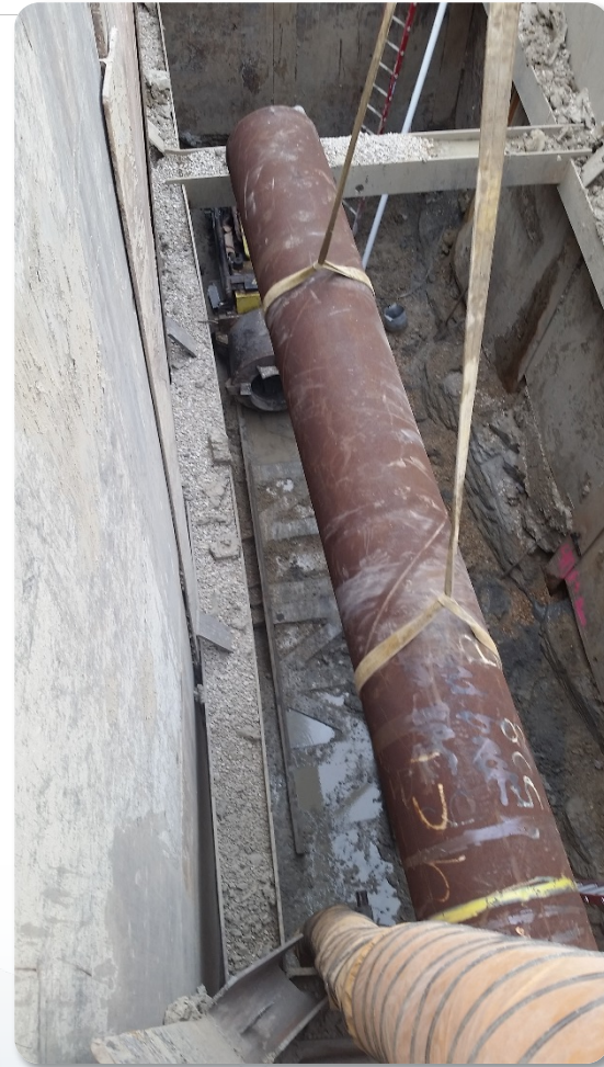
Little Walnut Creek - Boring Operation
