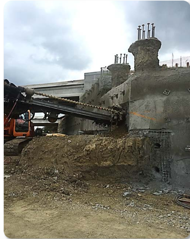
Soil Nail Wall Construction at Springdale/Manor Interchange – NE Abutment
