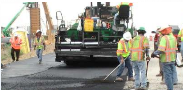
Warm Mix Asphalt Placement
