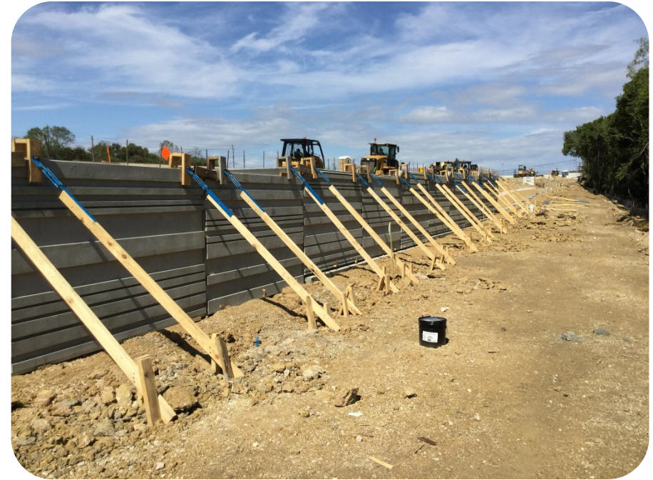
First MSE Wall Being Constructed SE of Springdale/Manor intersection
