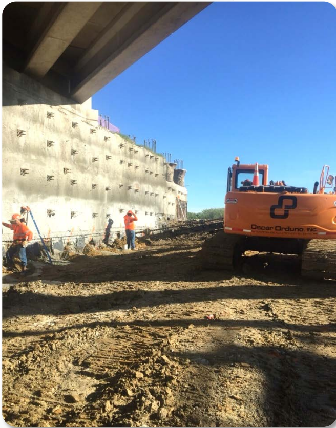
Soil Nail Wall Construction at Springdale/Manor Interchange – NE Abutment
