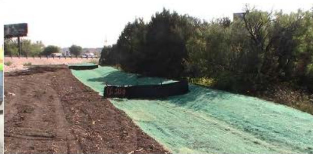
Soil Retention Blanket for improving Erosion Control
