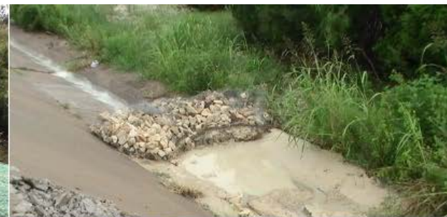
Rock Filter Dam for preserving Water Quality
