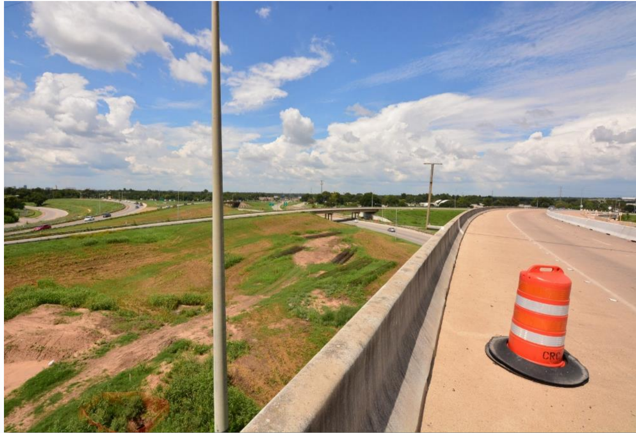
Colorado River Bridge – August 2016
