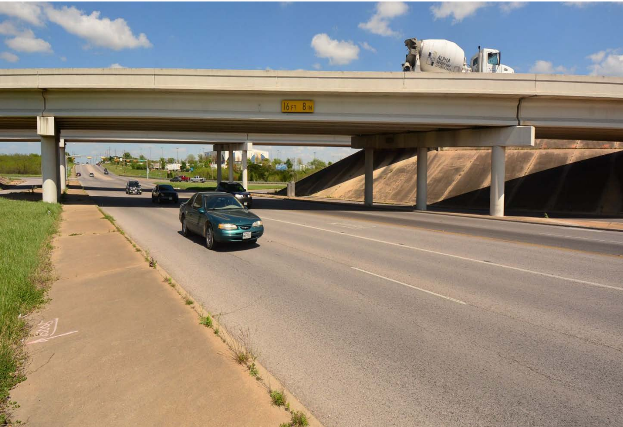
Springdale Before Cladding
