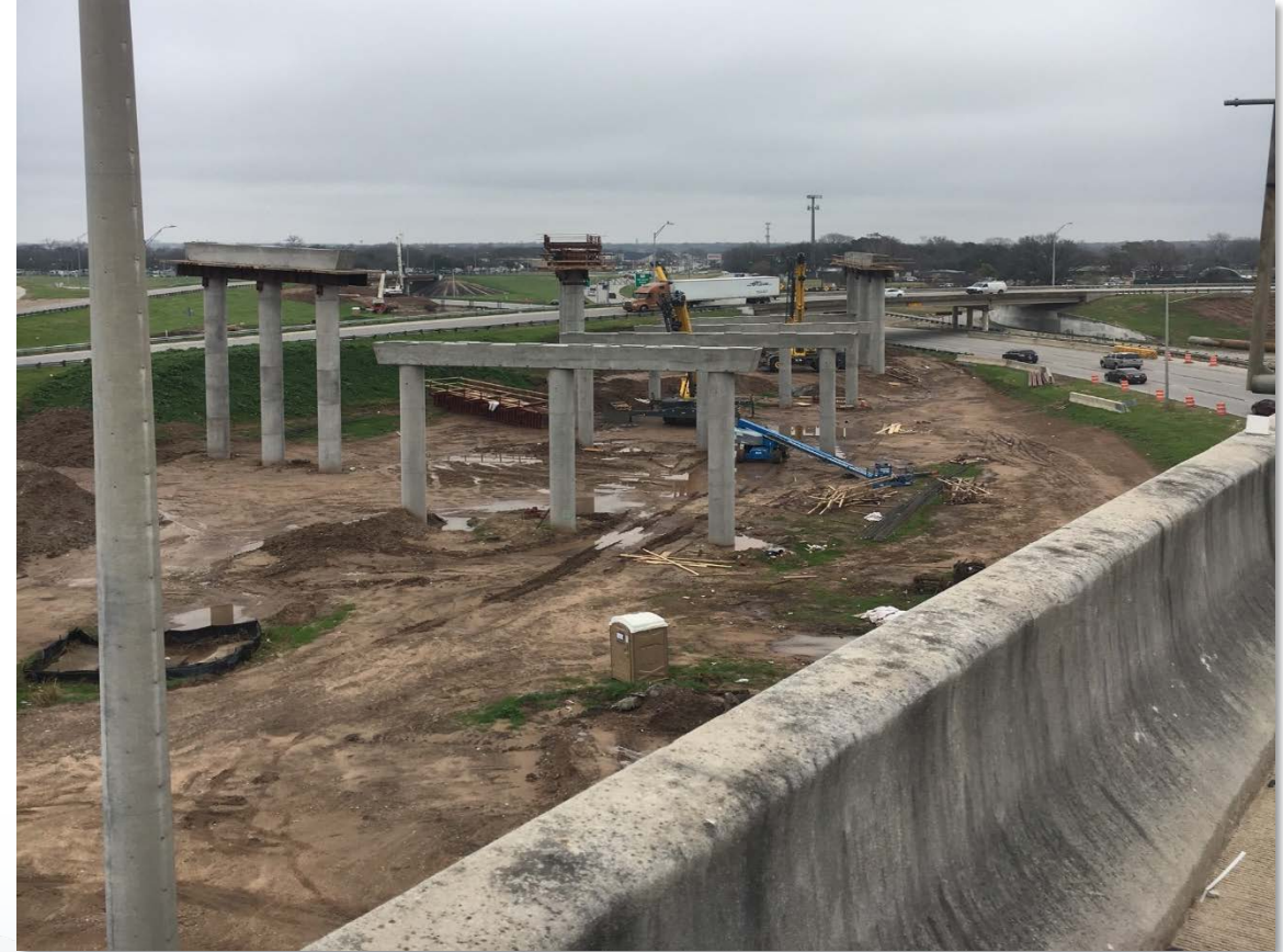
Colorado River Bridge – December 2016
