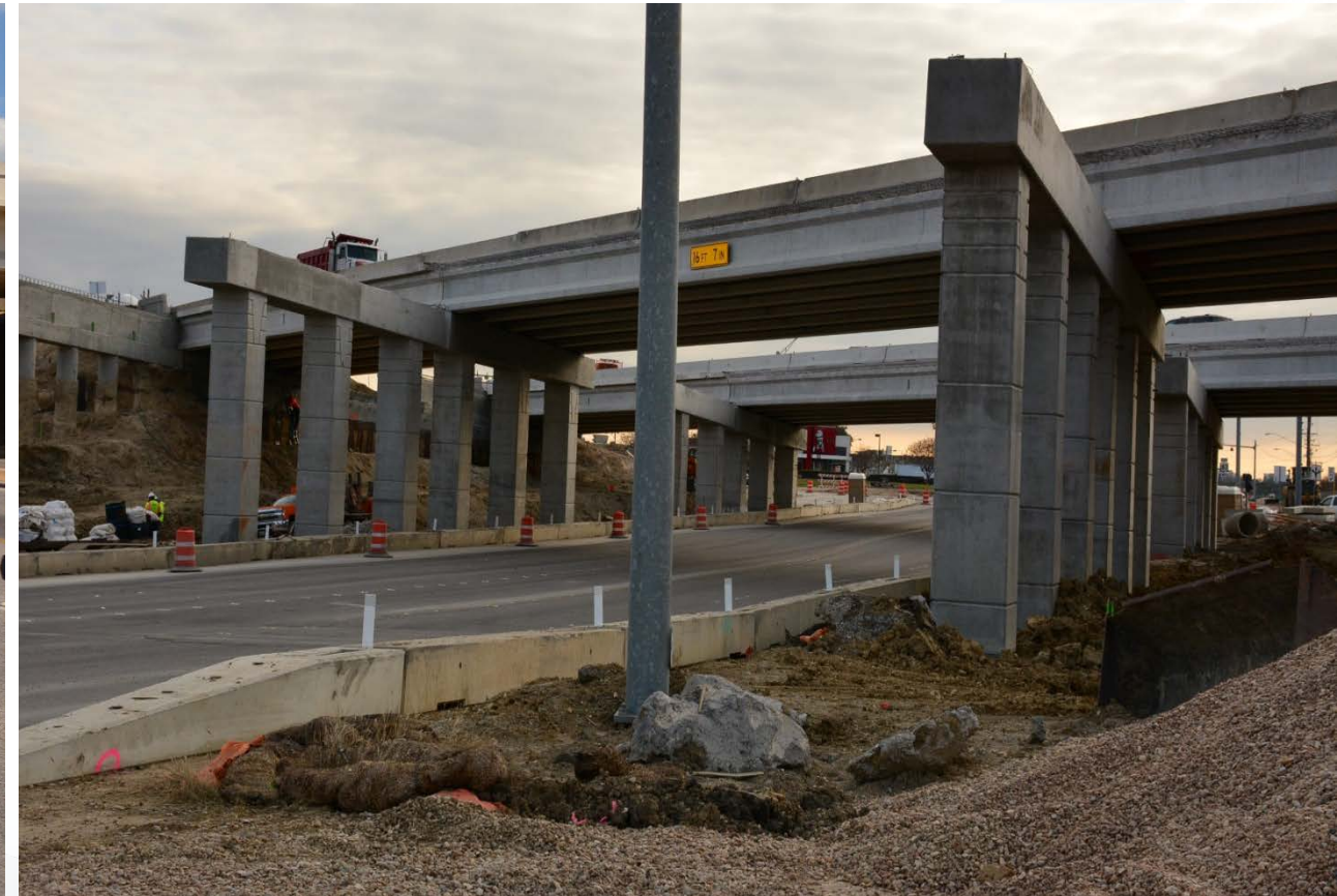
Springdale After Cladding
