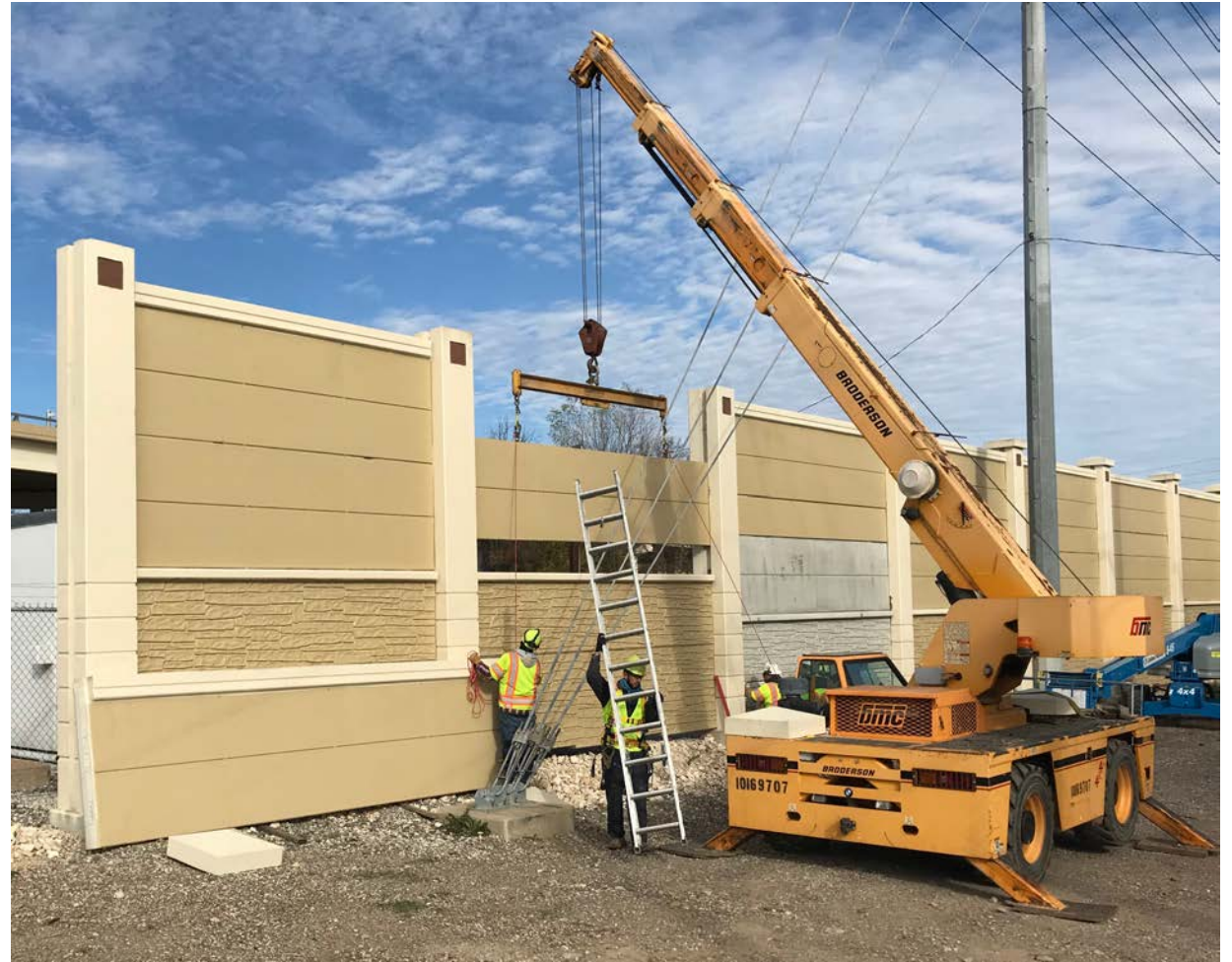
Wall 3 installation at RM 2222
