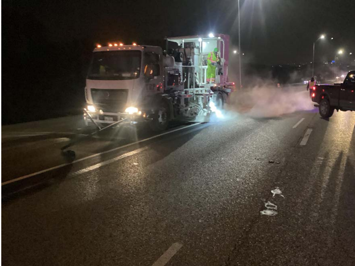
Pavement Marking Removal January 2024
