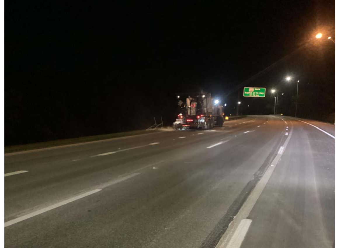
Pavement Marking Installation January 2024
