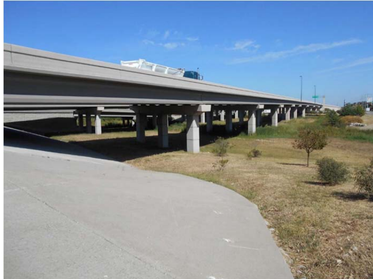
Northbound Mainlane Bridge at FM 1431
