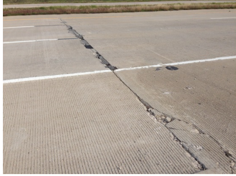
Southbound Mainlanes North of RM 1431
