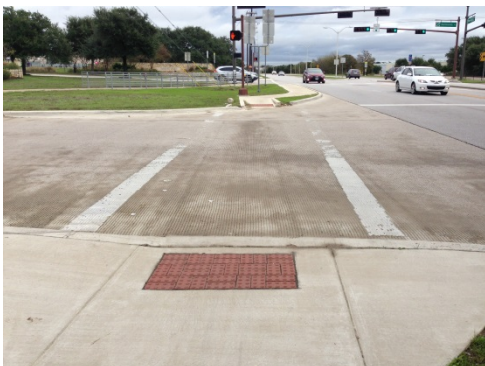
Observed Crosswalk Fading
