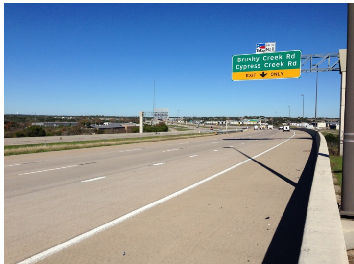
183A Turnpike at Brushy Creek looking North
