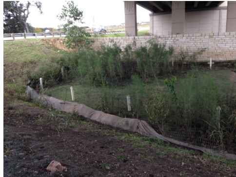
Observed Vegetation in Sand Filter Basin
