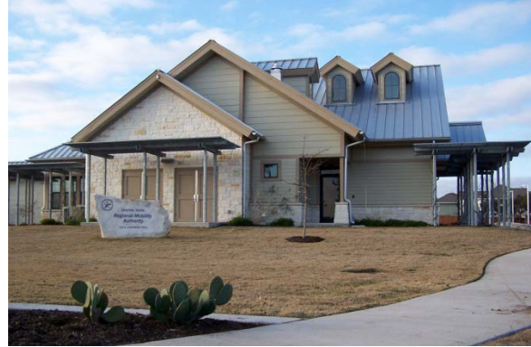
183A Turnpike Traffic Operations Center (formerly called Field Operations Building)
