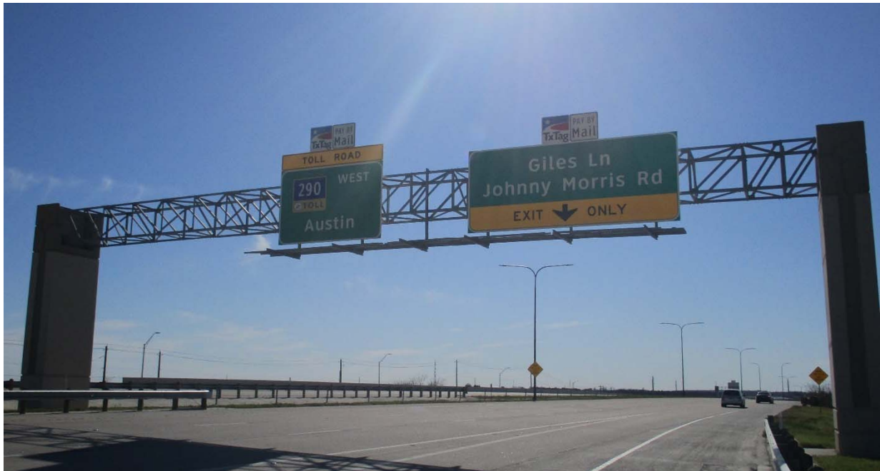
Overhead sign structure westbound approaching Johnny Morris Rd
